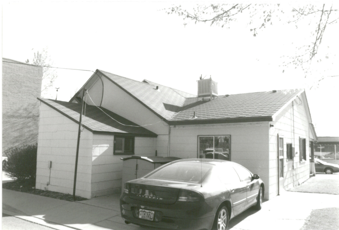
5BL8039 717 Main Street, Louisville House / City of Louisville Parks and Recreation Building 27 April 2000 Negative located at: City of Louisville 749 Main Street, Louisville, CO 80027 Photographed by Carl McWilliams Roll CM-11 Frame 8 View to NW
