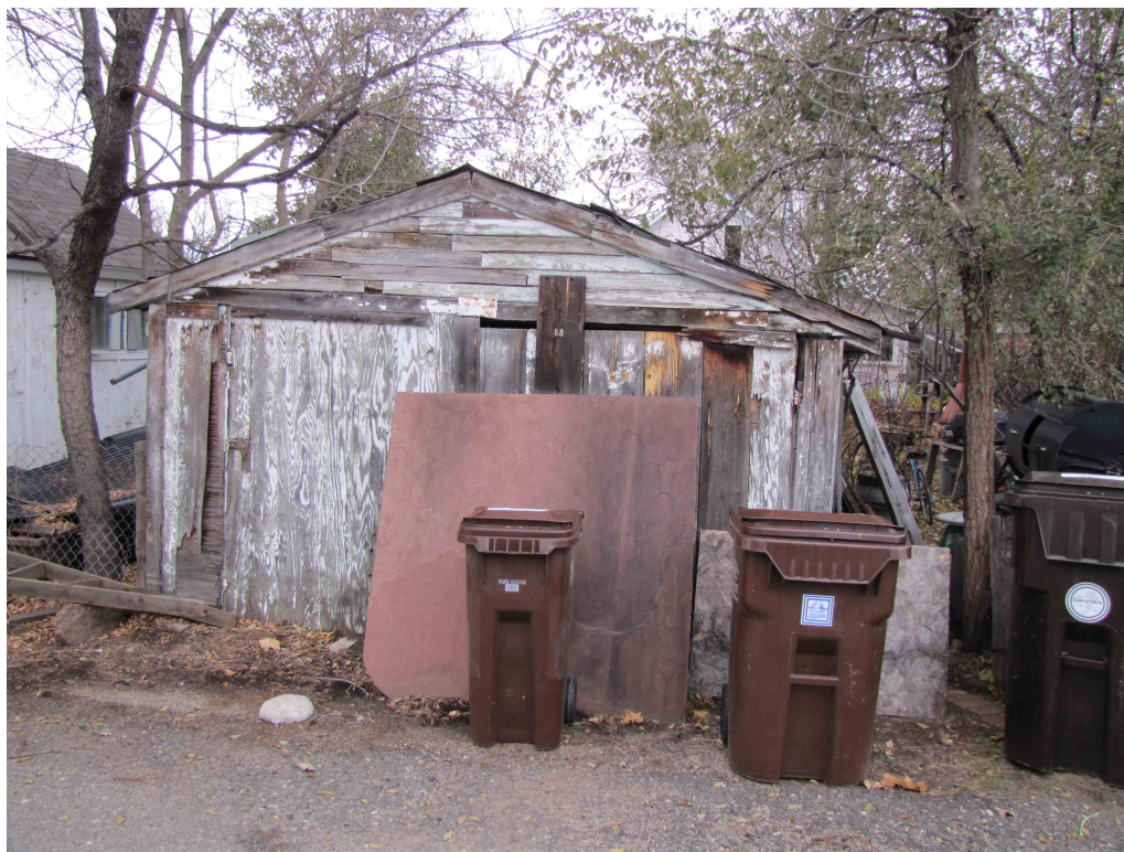
5BL7978_617LaFarge_05 Garage West
