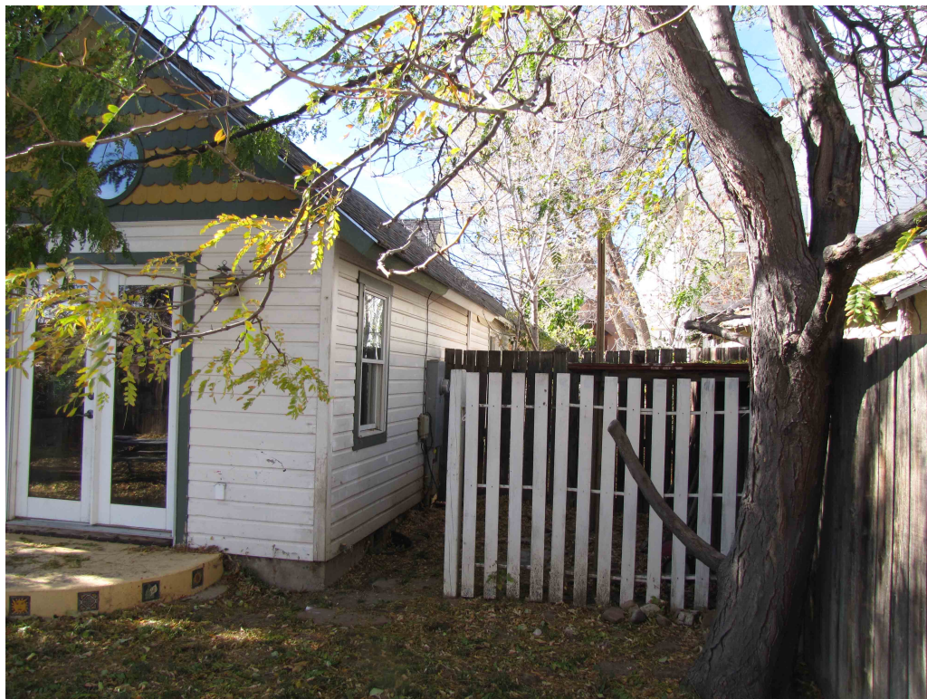
5BL7992_824LaFarge_07 northeast side
