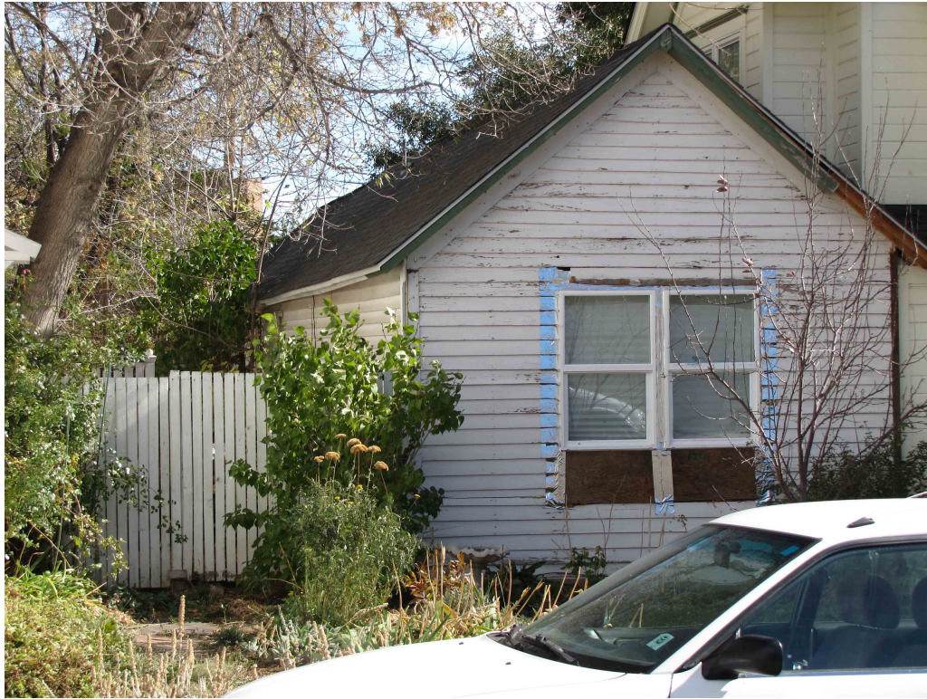
5BL7992_824LaFarge_03 North, original house
