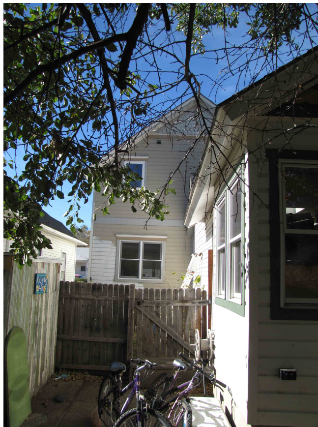
5BL7992_824LaFarge_05 East side of 2-story addition
