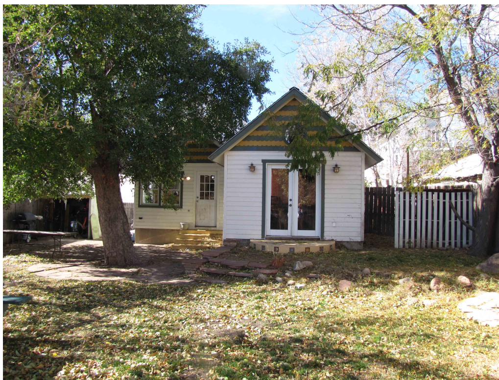
5BL7992_824LaFarge_06 Addition, east
