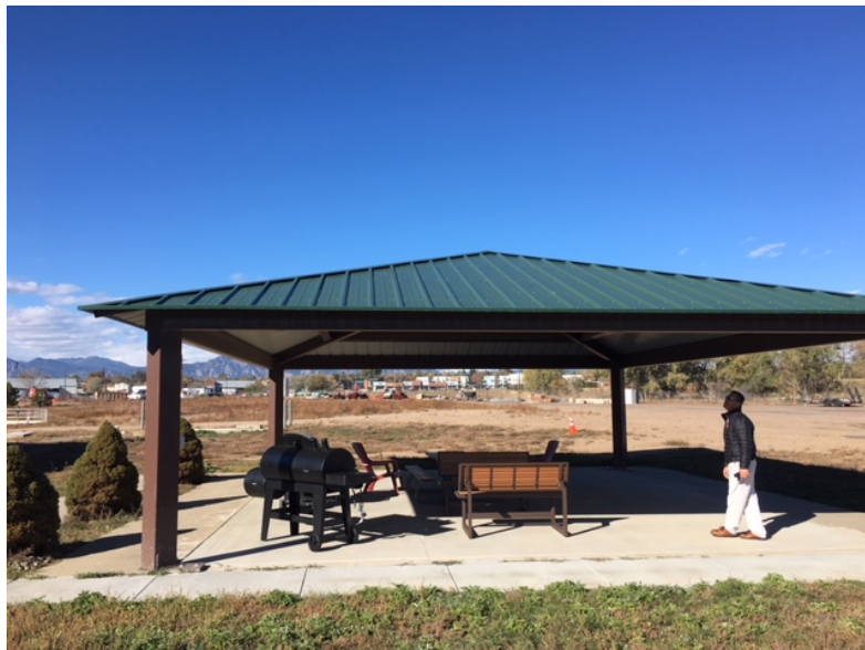
Photo #1 - Waste Water Pavilion
