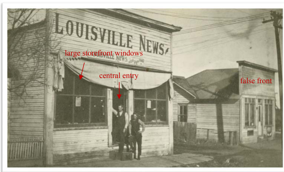
Figure 89. Buildings on the north side of Pine Street between Main and Front Streets, early 1900s (photo credit: Louisville Historical Museum).
