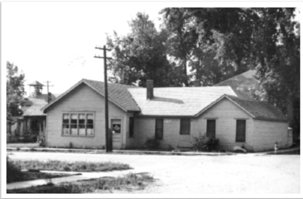
Figure 83. Assessor card photograph of 800/804 Spruce Street, 1948 (Louisville Historical Museum 2017).
