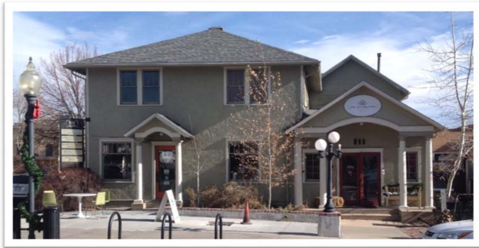
Figure B.13. 844 Main Street mixed-use residential and commercial.
