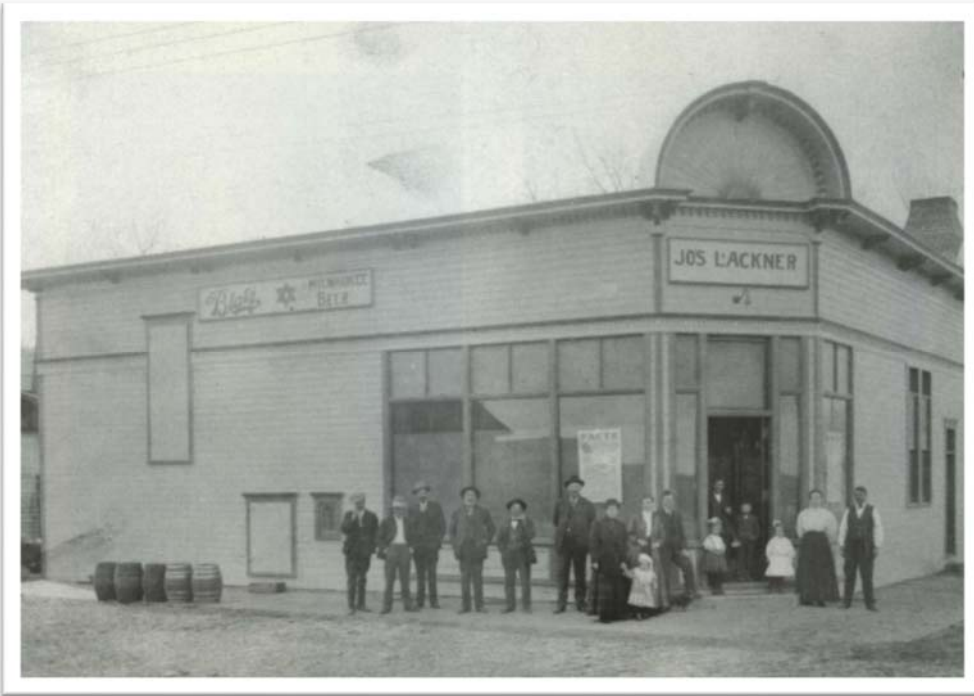
Figure 121. 1006 Pine Street, 1908 (photo credit: Louisville Historical Museum).
