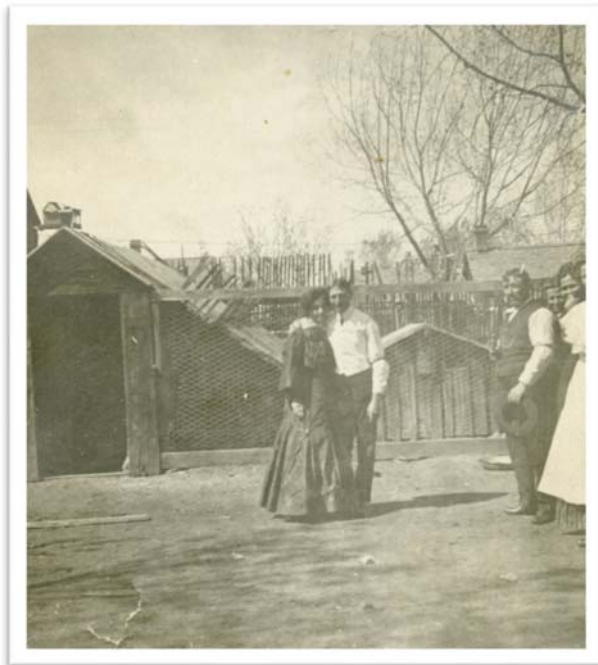
Figure 72. Chicken coop, formerly located behind 717 Main Street, ca. 1910 (photo credit: Louisville Historical Museum).
