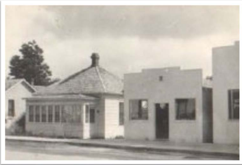
Figure 57. Assessor card photograph of 920 Main Street (right-center), 1948 (Louisville Historical Museum 2017).
