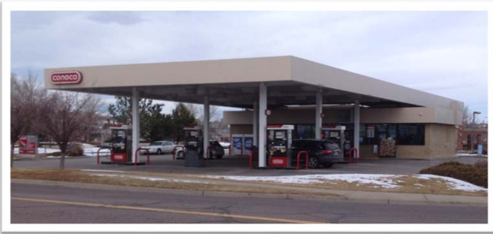
Figure 163. 520 McCaslin Boulevard today.
