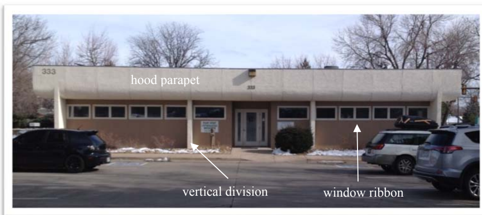
Figure 181. 333 W. South Boulder Road today.
