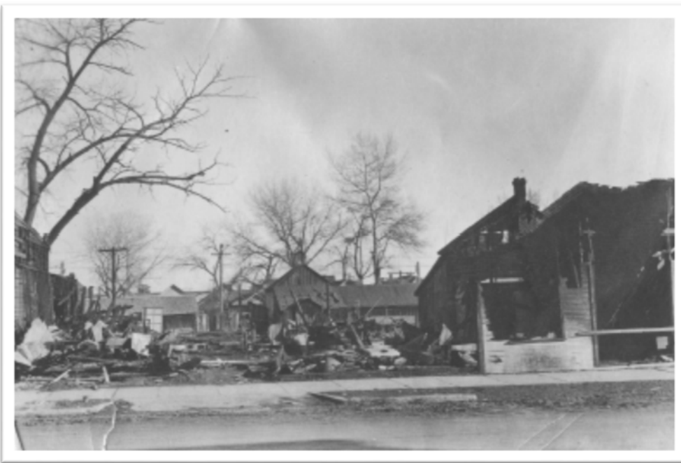
Figure 9. Site of the 1926 fire, after the Telephone Exchange rubble was removed (photo credit: Louisville Historical Museum).
