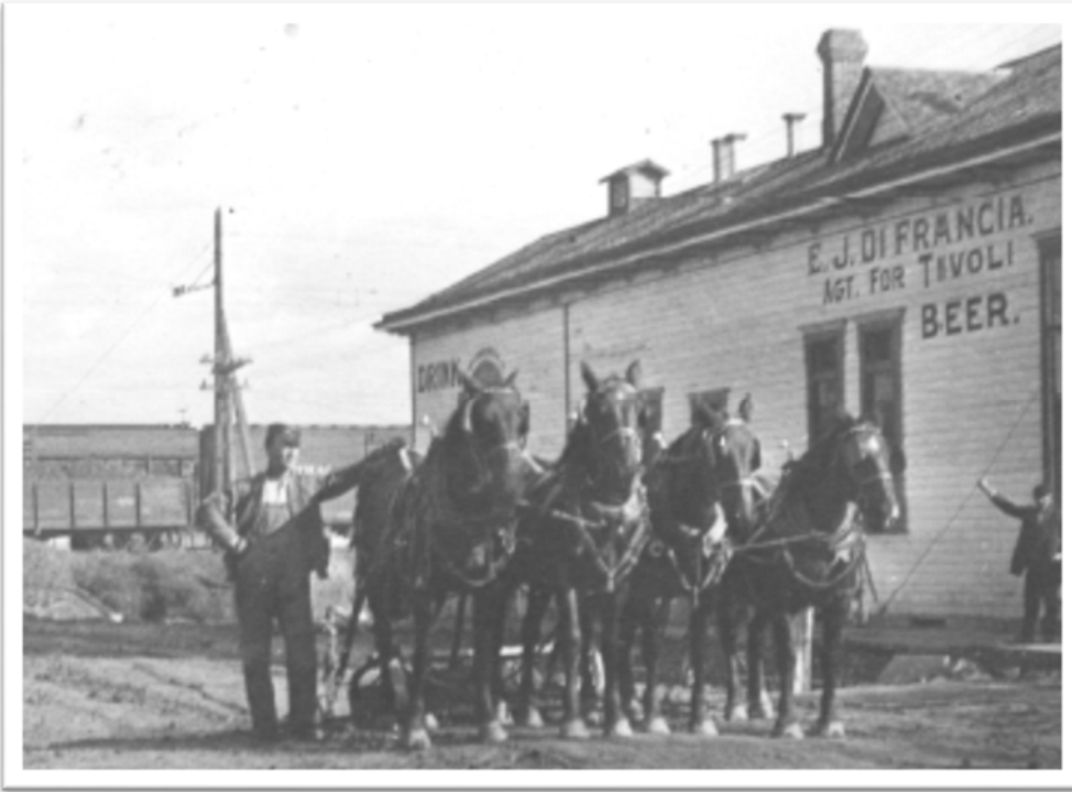
Figure 40. Franzia's/Di Francia's Saloon on Front Street, 1913 (photo credit: Louisville Historical Museum).
