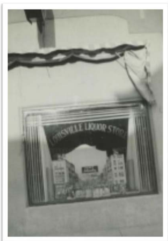
Figure 152. 820 Main Street partial façade, 1930s (photo credit: Louisville Historical Museum).
