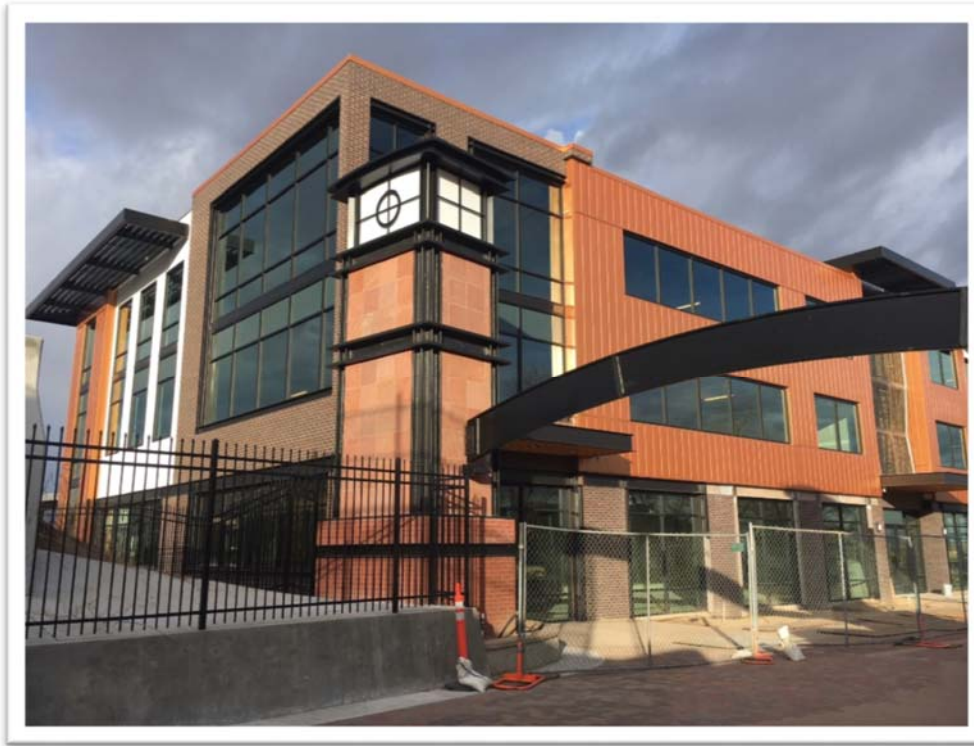
Figure 190. 21st-Century Modern commercial building in DELO today.
