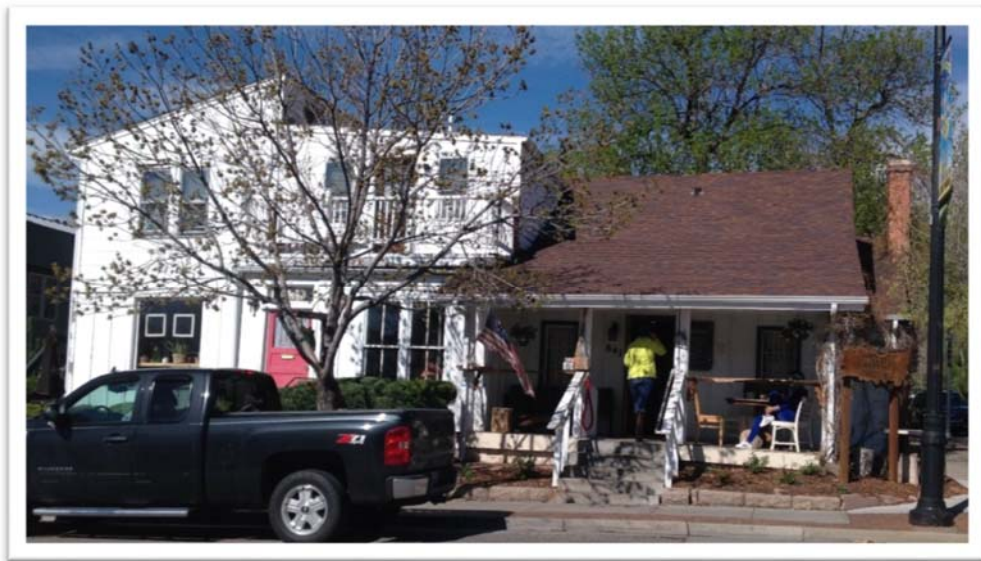
Figure B.11. 641 Main Street mixed-use residential and commercial.
