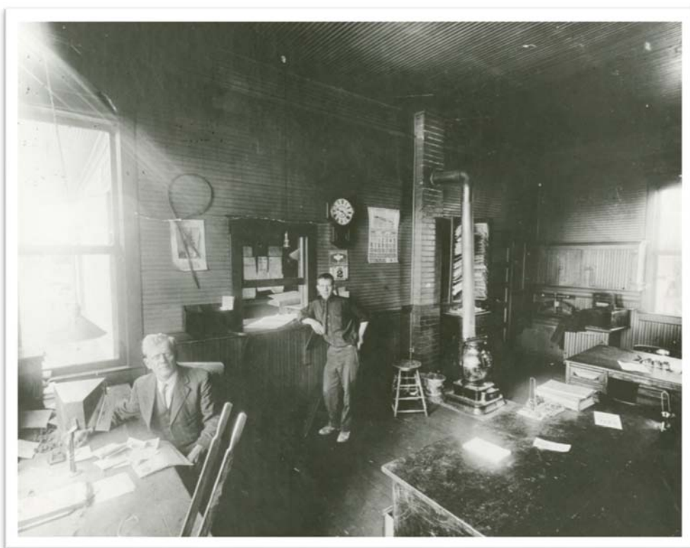
Figure 90. C&S depot interior, 1920 (photo credit: Louisville Historical Museum).
