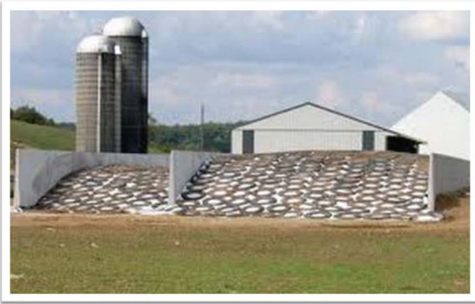
Figure 36. Bunker silo in Ontario, Canada, today (Bunker Silo Sidewalls 2018).
