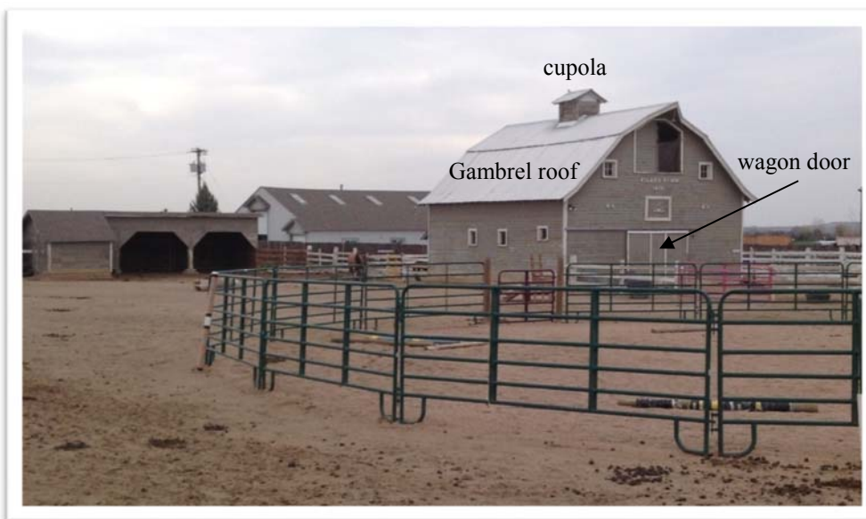
Figure 130. Gambrel roof barn on the Kilker Farm, today.
