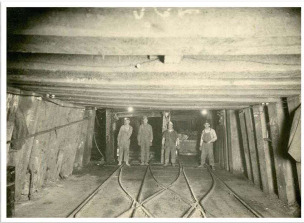
Figure 94. Coal car rails and men in the Hi-Way Mine, unknown date (photo credit: Louisville Historical Museum).
