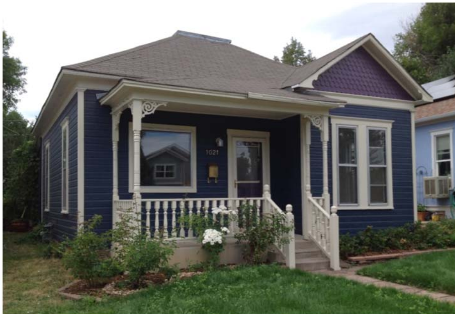
Figure B.20. 1021 La Farge Avenue.
