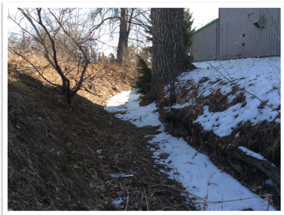
Figure B.2. Davidson Highline Lateral Ditch.
