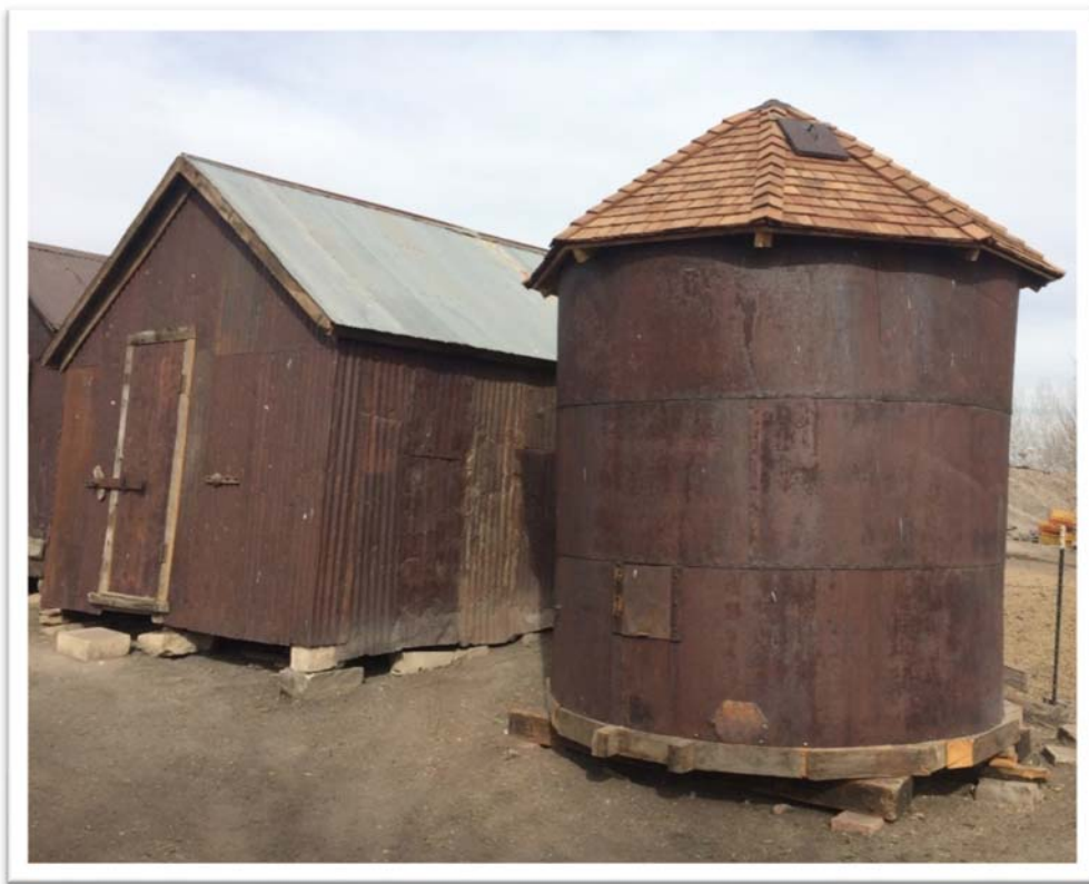
Figure 40. Metal granaries at the Harney-Lastoka/7th Generation Farm, 2016 (photo credit: Carol Beam).
