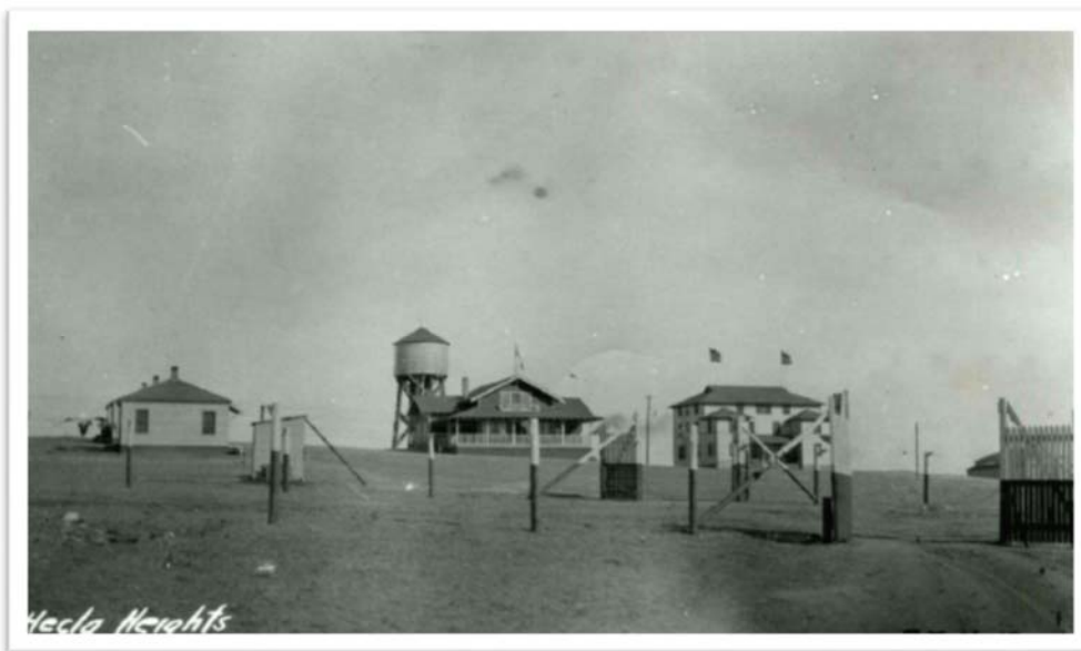
Figure 109. Hecla Mine houses, water tank, casino, and boarding house within a fenced compound, 1914 (photo credit: Louisville Historical Museum).
