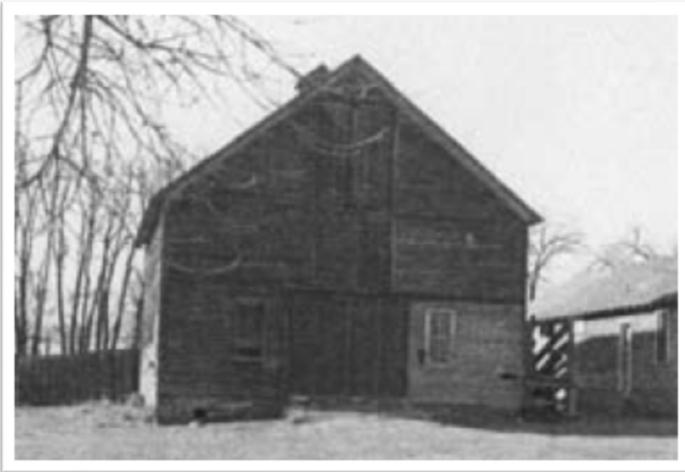
Figure 123. Gable roof barn on the Naeve Farm, late 1940s or early 1950s (LHM 2017).
