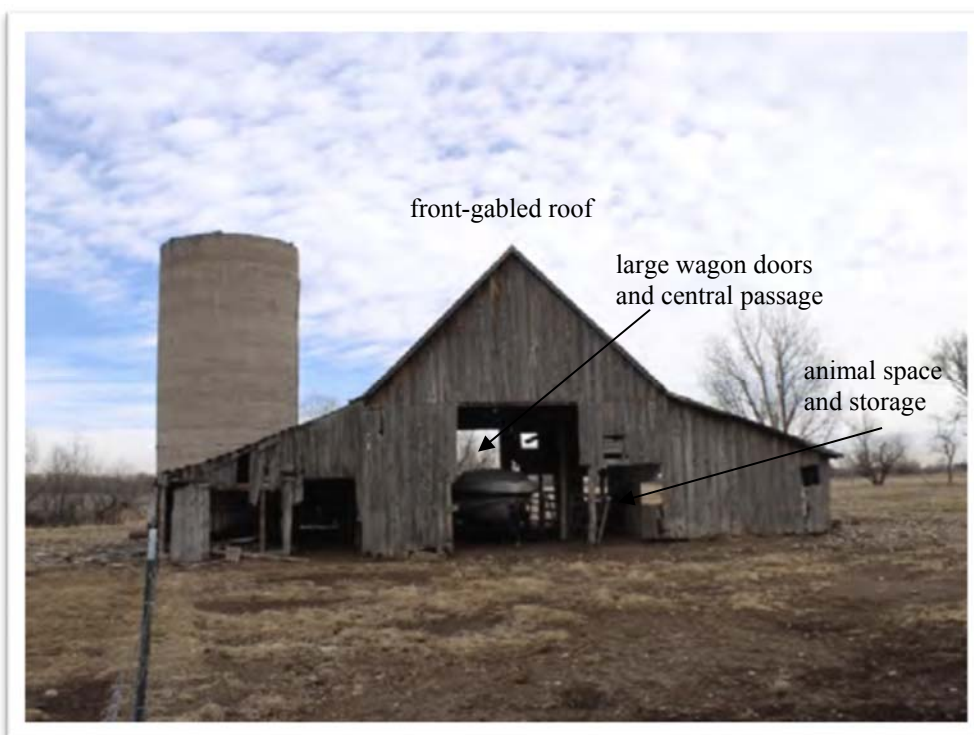
Figure 120. Transverse Frame barn (photo credit: Carol Beam [Wolfenbarger 2006:43]).
