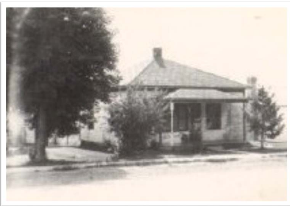
Figure 141. Assessor card photograph of 540 Lincoln Avenue, 1948 (Louisville Historical Museum 2017).
