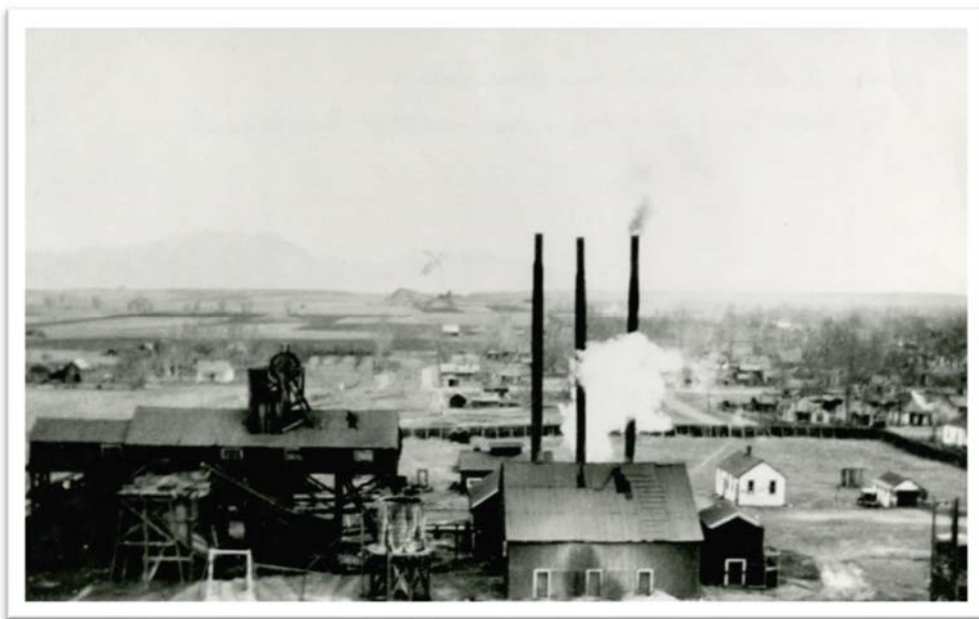
Figure 107. Acme Mine buildings, view to west, pre-1901 (photo credit: Louisville Historical Museum).
