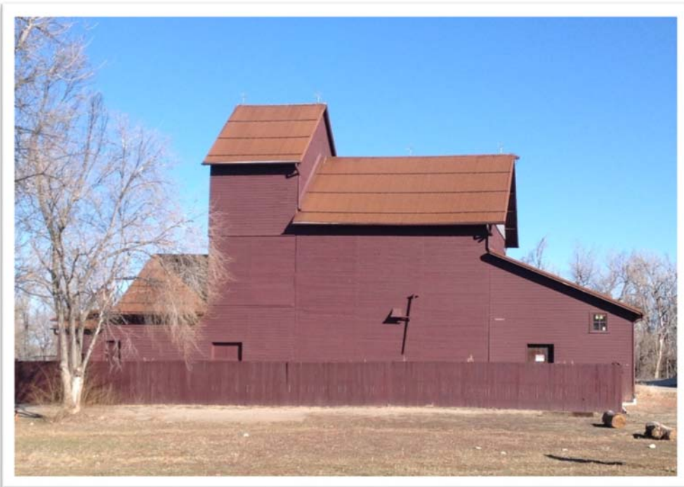
Figure 31. Louisville grain elevator, today.
