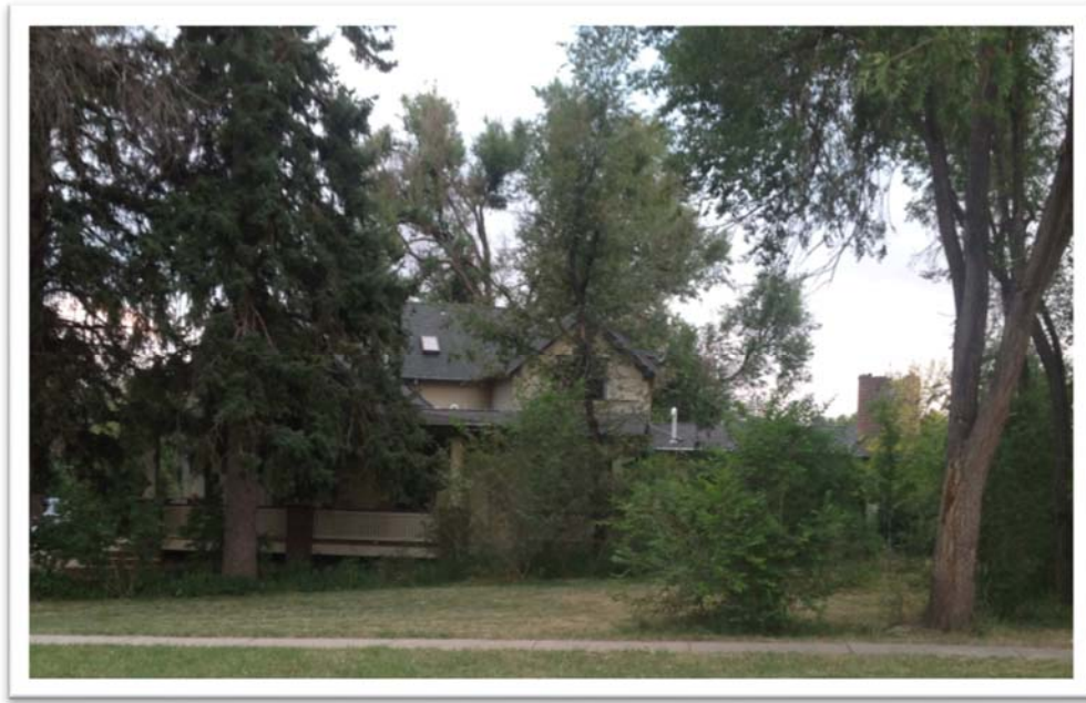
Figure B.17. 310 W. Spruce Street.
