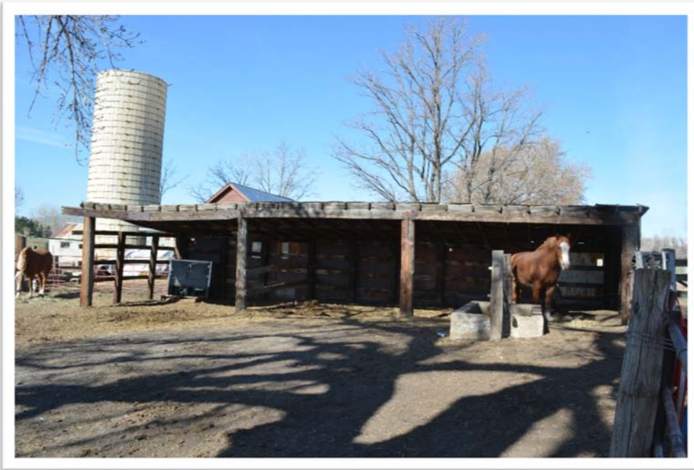
Figure 42. Loafing shed at the Harney-Lastoka/7th Generation Farm, 2016 (photo credit: Carol Beam).
