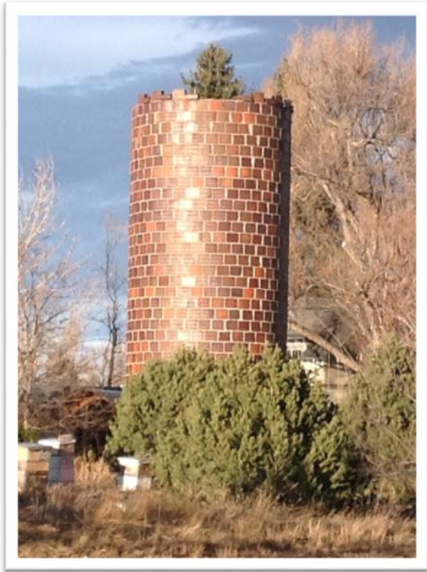
Figure 32. Hollow glazed-clay tile silo on the former Gosselin Farm between Pine and W. Spruce Streets, today.
