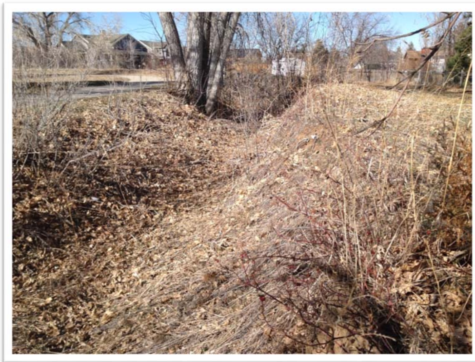
Figure 21. Louisville Lateral Ditch, today.
