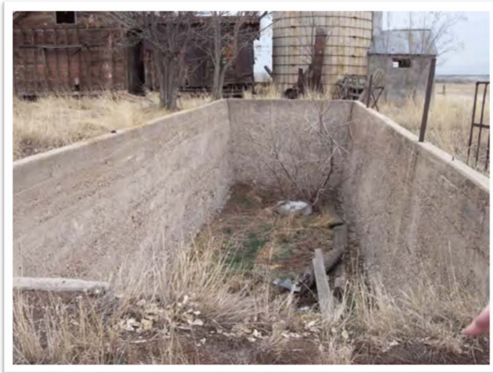
Figure 35. Trench silo on the Harney-Lastoka/7th Generation Farm, ca. 2006 (photo credit: Carol Beam [Wolfengarger 2006:49]).
