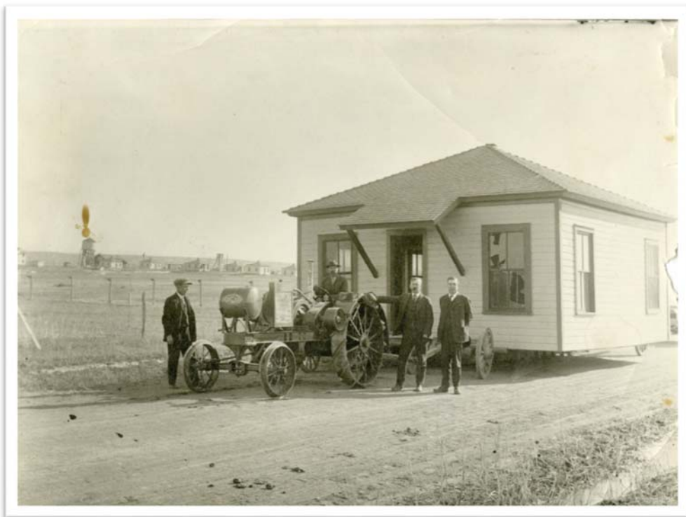
Figure 138. Type E house being moved from Hecla Heights into town, 1916 (photo credit: Louisville Historical Museum).
