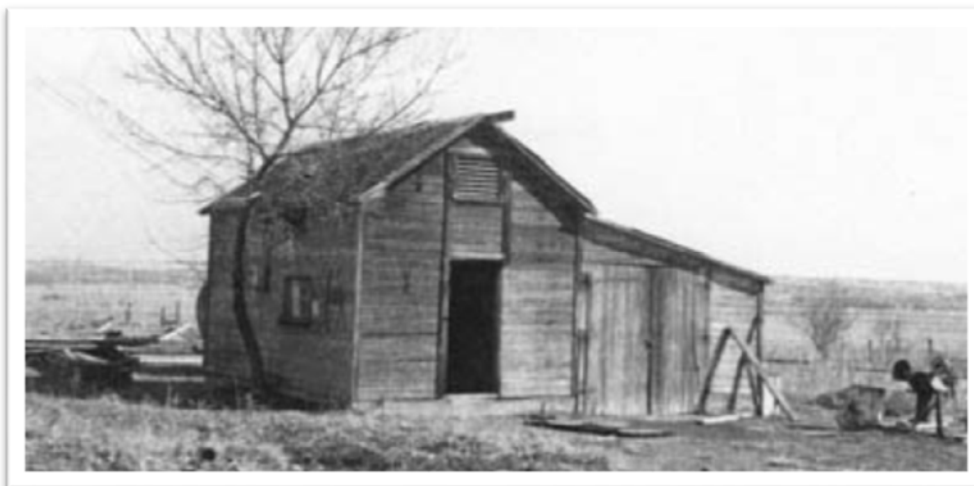
Figure 126. Broken Gable barn on the Naeve Farm, late 1940s or early 1950s (LHM 2017).
