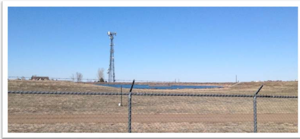
Figure 23. Louisville Reservoir, today.
