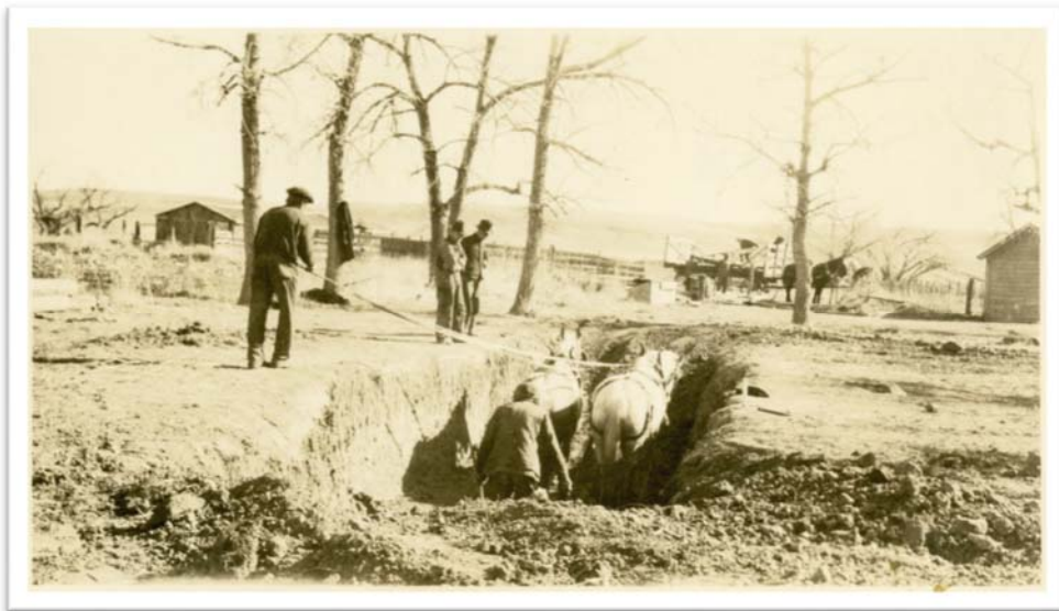
Figure 93. Excavating the shaft of the Hi-Way Mine, 1927 (photo credit: Louisville Historical Museum).
