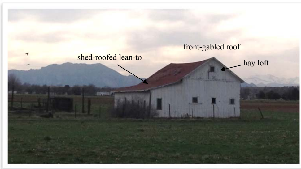
Figure 125. Broken Gable barn on the Kerr/Mayhoffer Farm, today.
