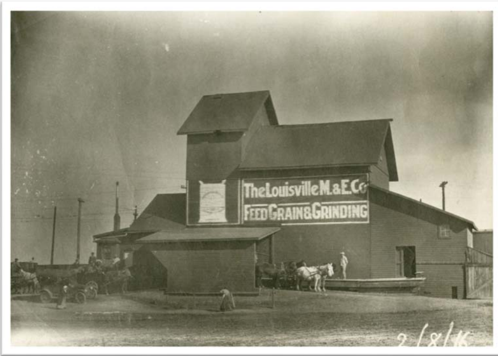
Figure 30. Louisville grain elevator, 1916 (photo credit: Louisville Historical Museum).
