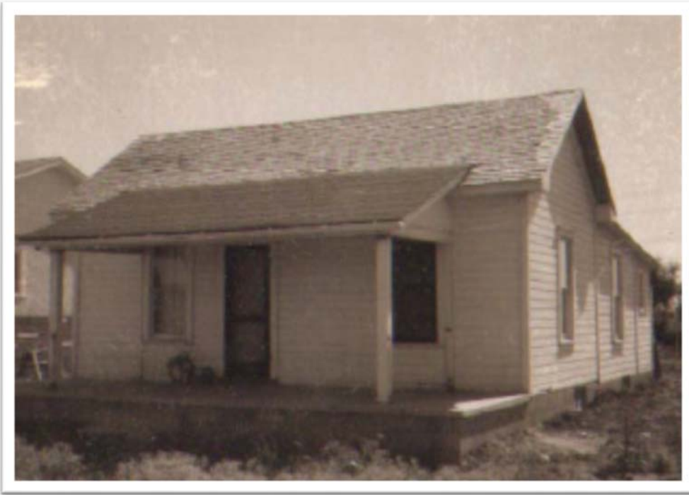
Figure 90. Assessor card photograph of 1300 Lincoln Avenue in 1960 (LHM 2017).
