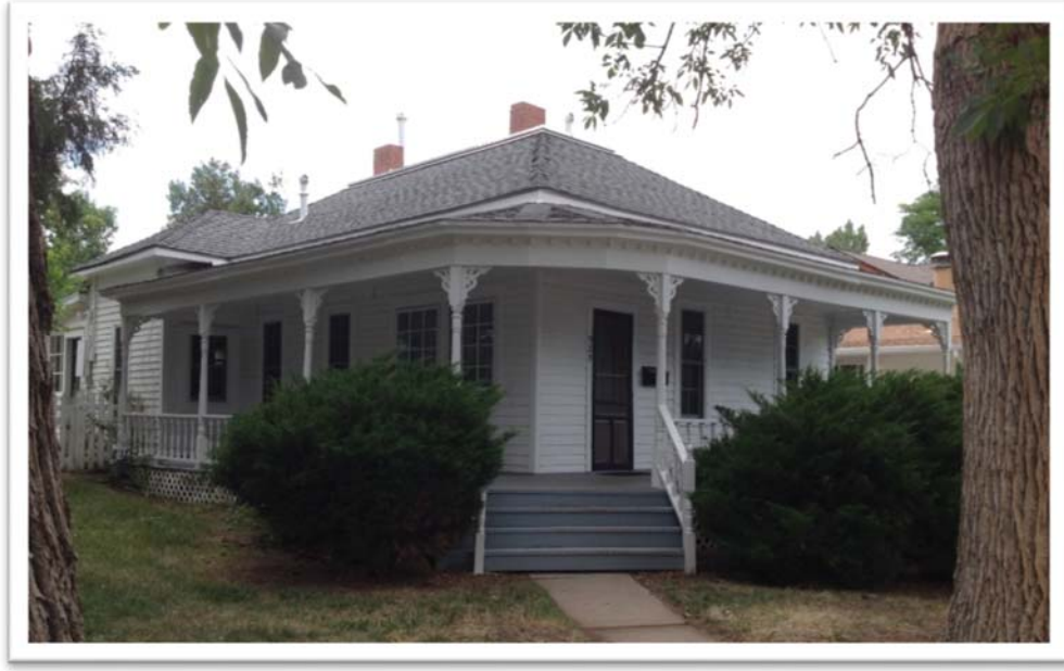
Figure B.11. 925 Jefferson Avenue.
