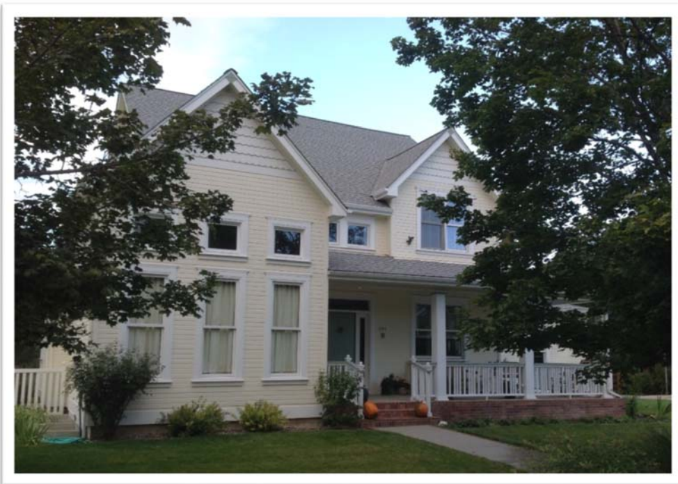
Figure 105. New Traditional house at 255 McKinley Park Lane constructed in 1997.
