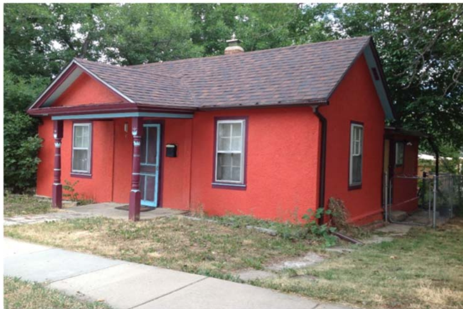
Figure B.3. 620 Jefferson Avenue.
