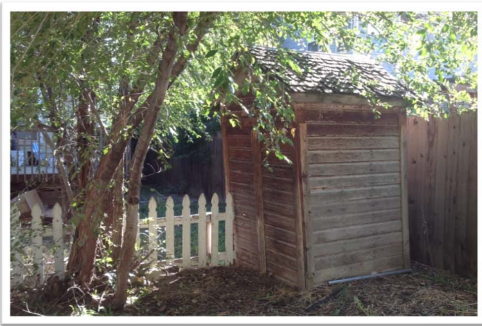
Figure 138. Outbuilding at 733 Pine Street today.
