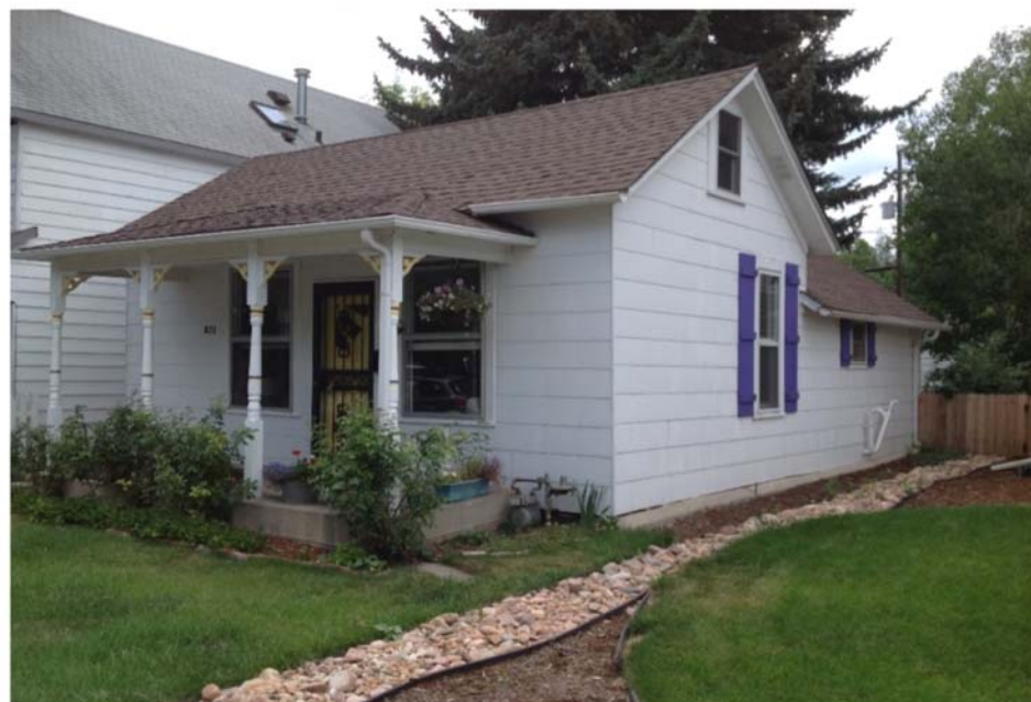
Figure B.4. 821 La Farge Avenue.
