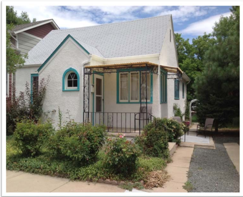
Figure B.5. 1008 La Farge Avenue.
