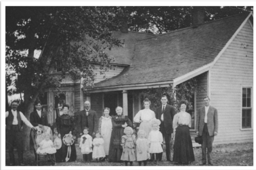
Figure 81. Historical photograph of 225 Roosevelt Avenue in 1908 (photo credit: LHM).
