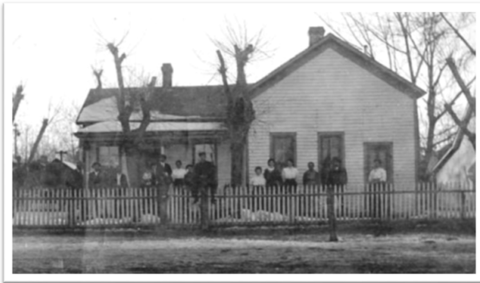
Figure 9. Austin-Niehoff House, ca. 1895 to 1900 (photo credit: LHM).
