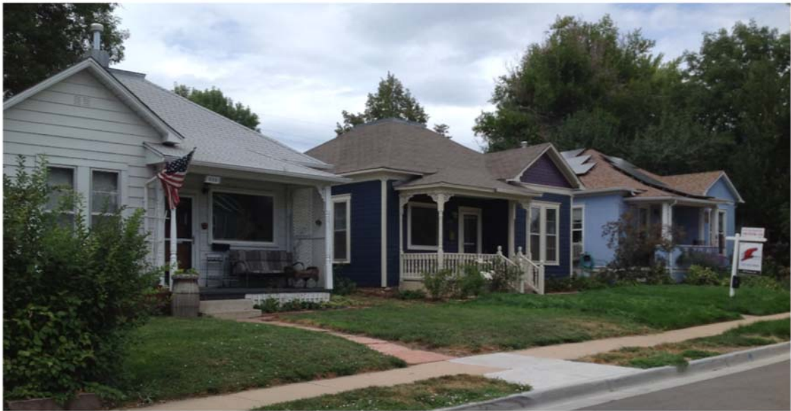
Figure B.51. Pyramidal/Hipped houses at 1013, 1021, and 1029 La Farge Avenue.
