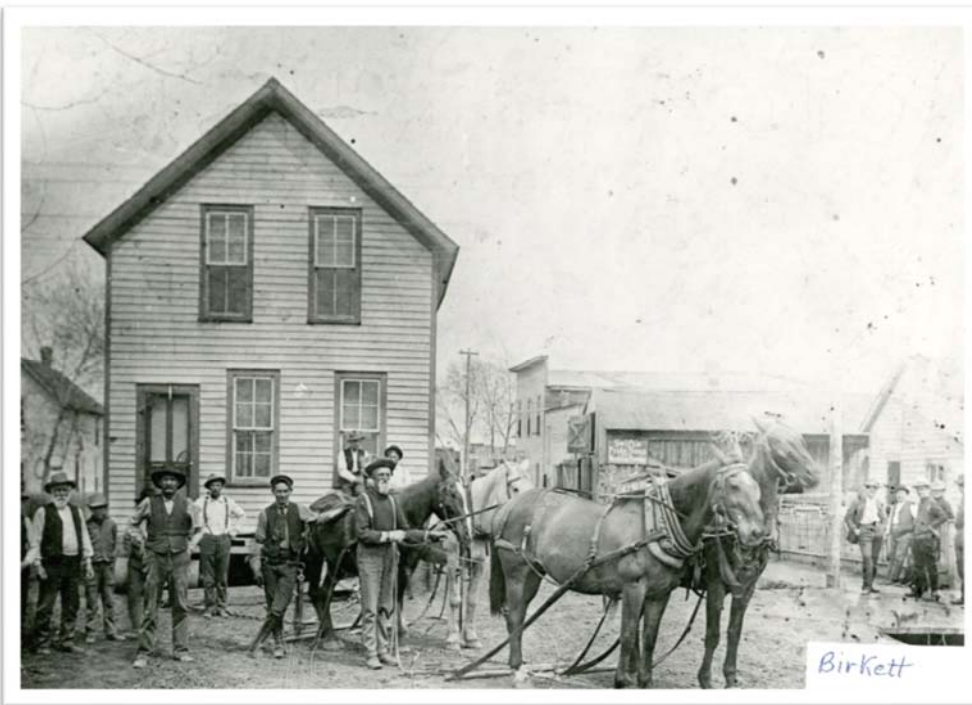
Figure 142. Moving a house in the early 1900s (photo credit: LHM).
