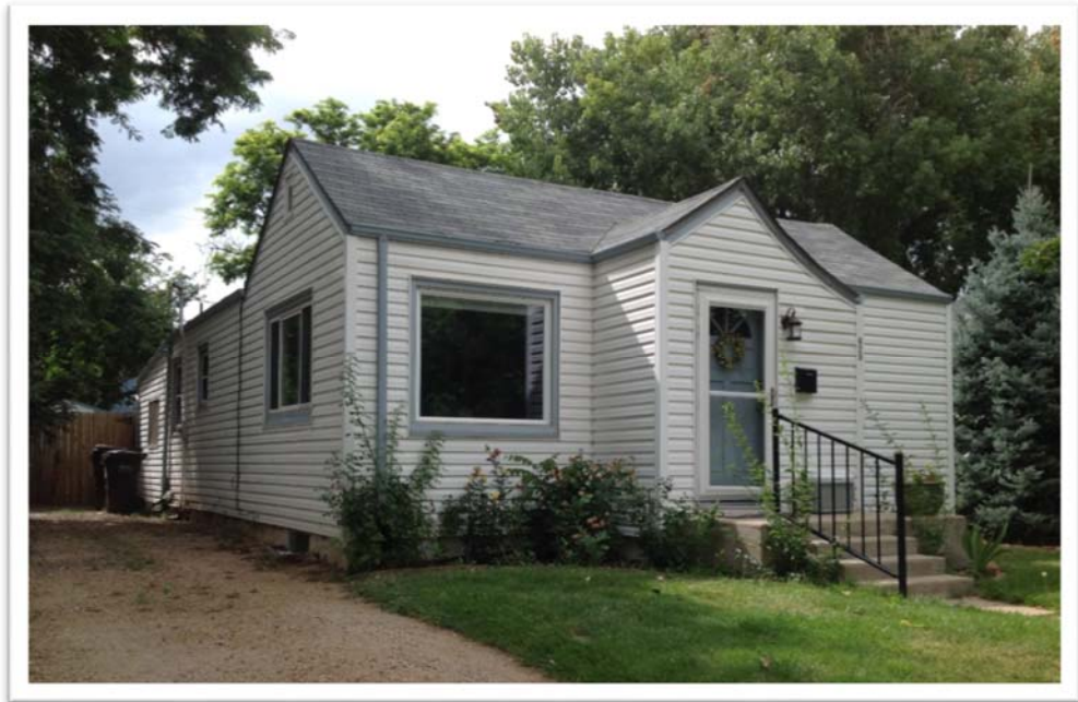
Figure B.48. 629 McKinley Avenue.
