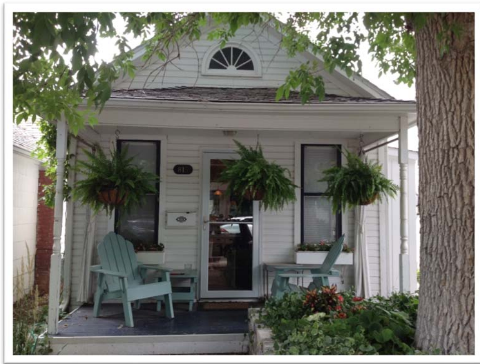
Figure B.12. 815 La Farge Avenue.
