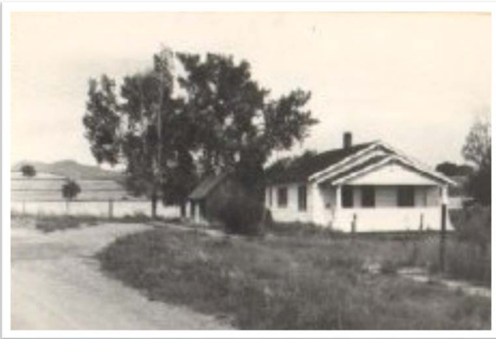
Figure 70. Assessor card photograph of 1201 Lincoln Avenue in 1948 (LHM 2017).
