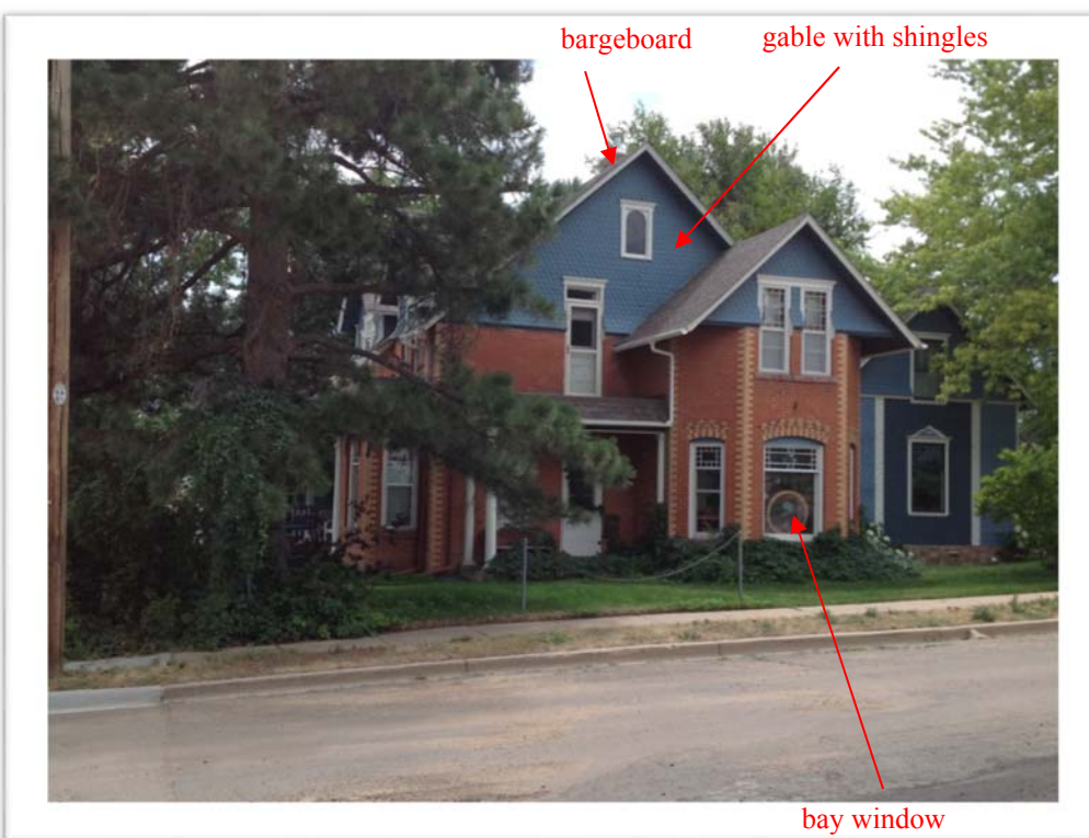
Figure 111. 1045 La Farge Avenue today, side view.
