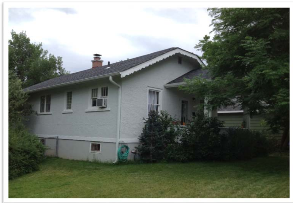
Figure B.29. 1208 Jefferson Avenue.
