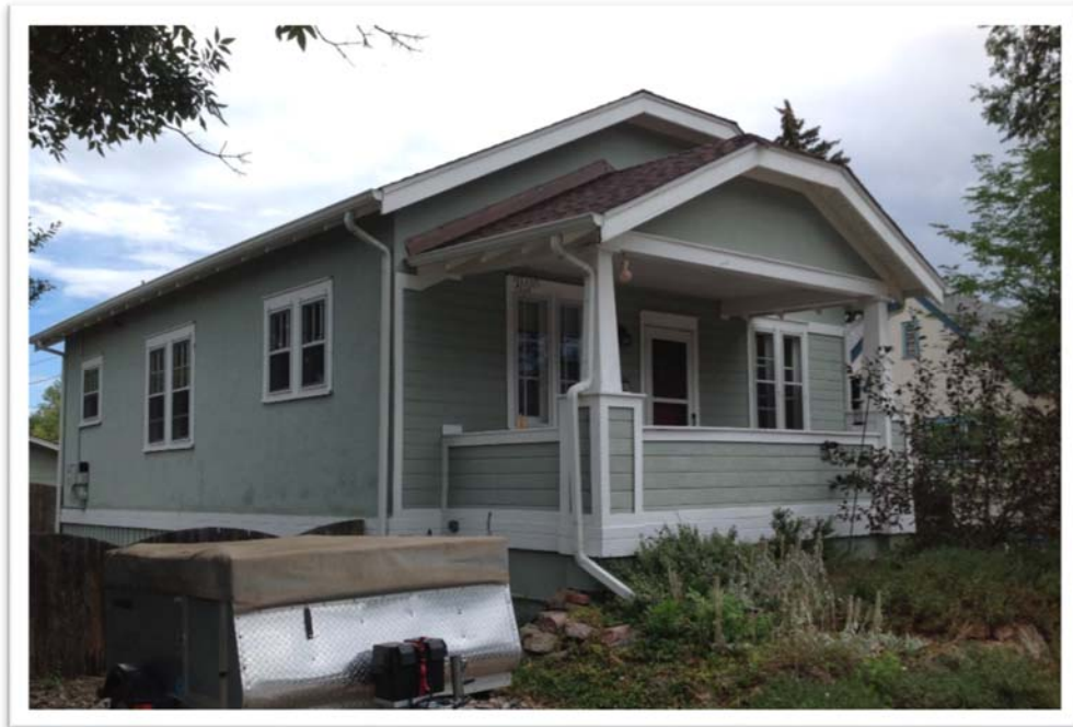
Figure B.28. 560 Jefferson Avenue.
