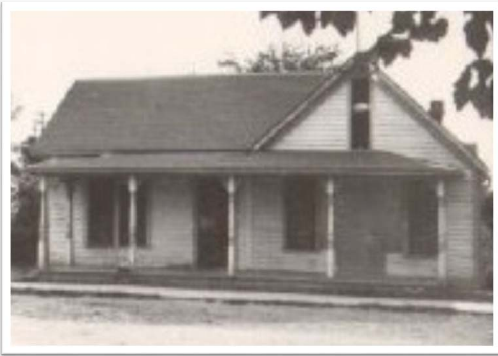
Figure 19. Assessor card photograph of 928 La Farge Avenue in 1948 (LHM 2017).
