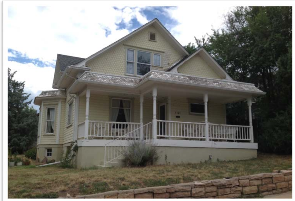
Figure B.19. 1101 Jefferson Avenue.
