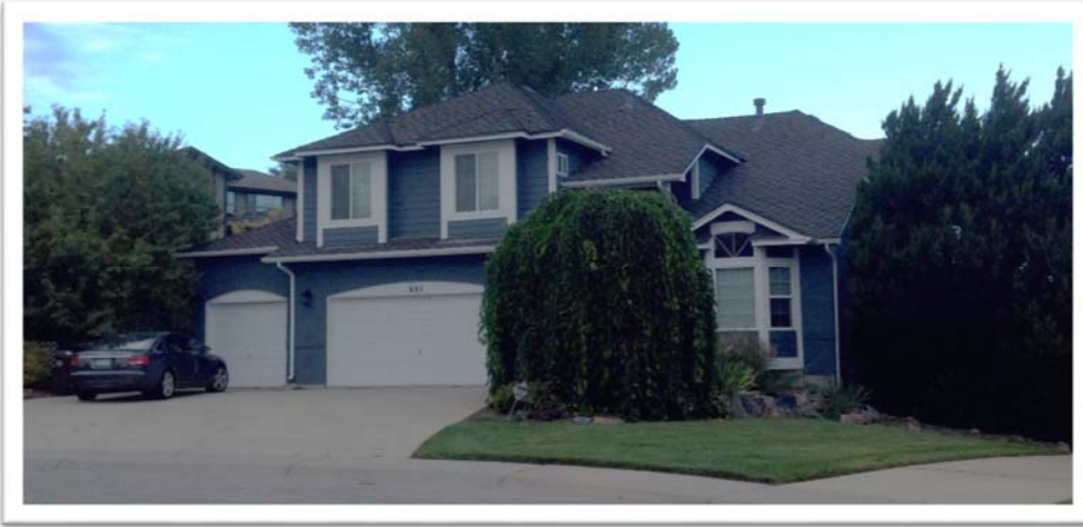
Figure 104. Millennium Mansion house at 651 Tamarisk Court constructed in 1991.
