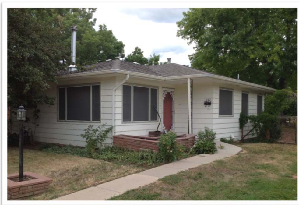
Figure B.47. 557 Jefferson Avenue.
