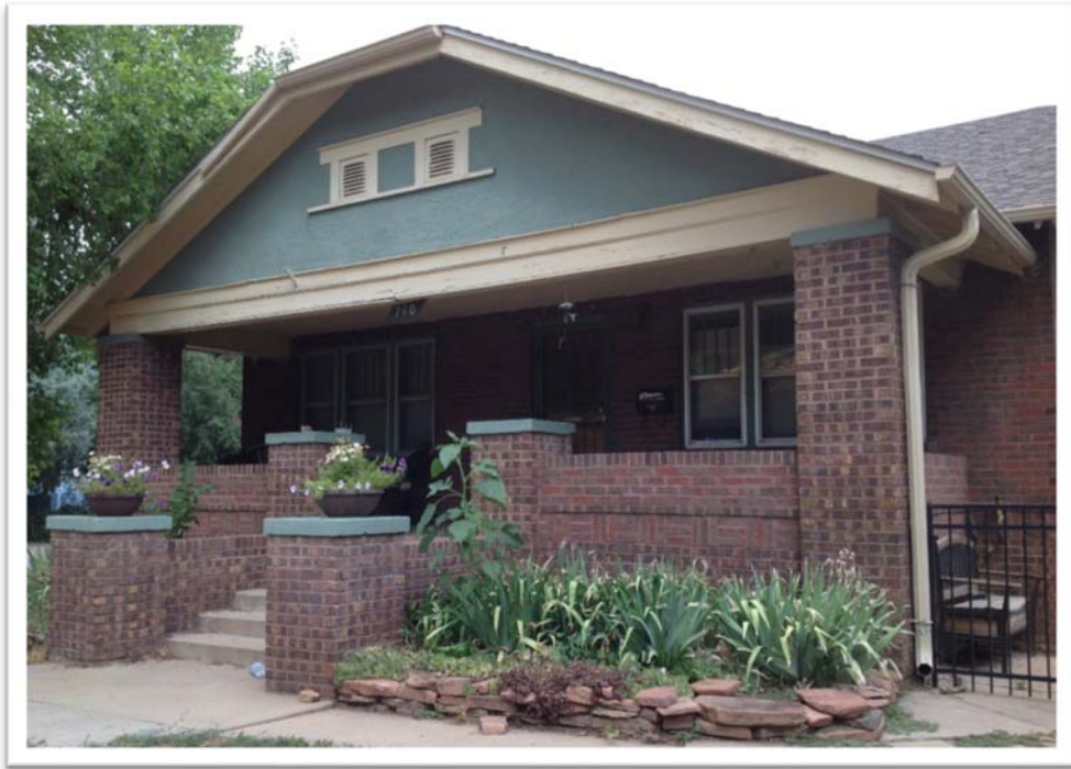
Figure B.26. 740 Garfield Avenue.
