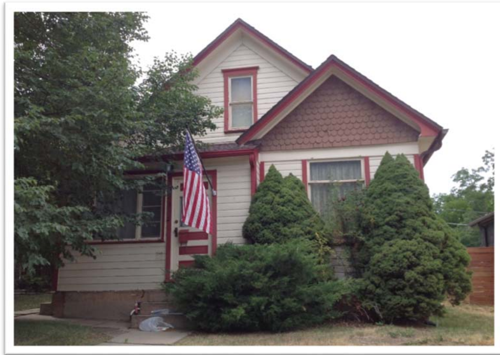
Figure B.13. 1145 La Farge Avenue.
