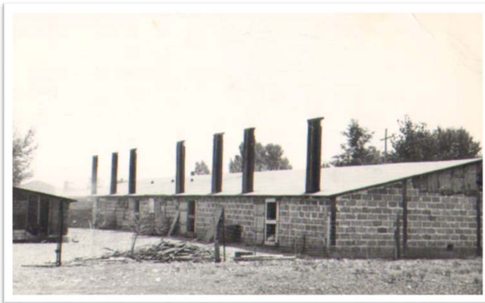
Figure 72. Chicken coop, formerly located behind 1245 Grant Avenue (LHM 2017).
