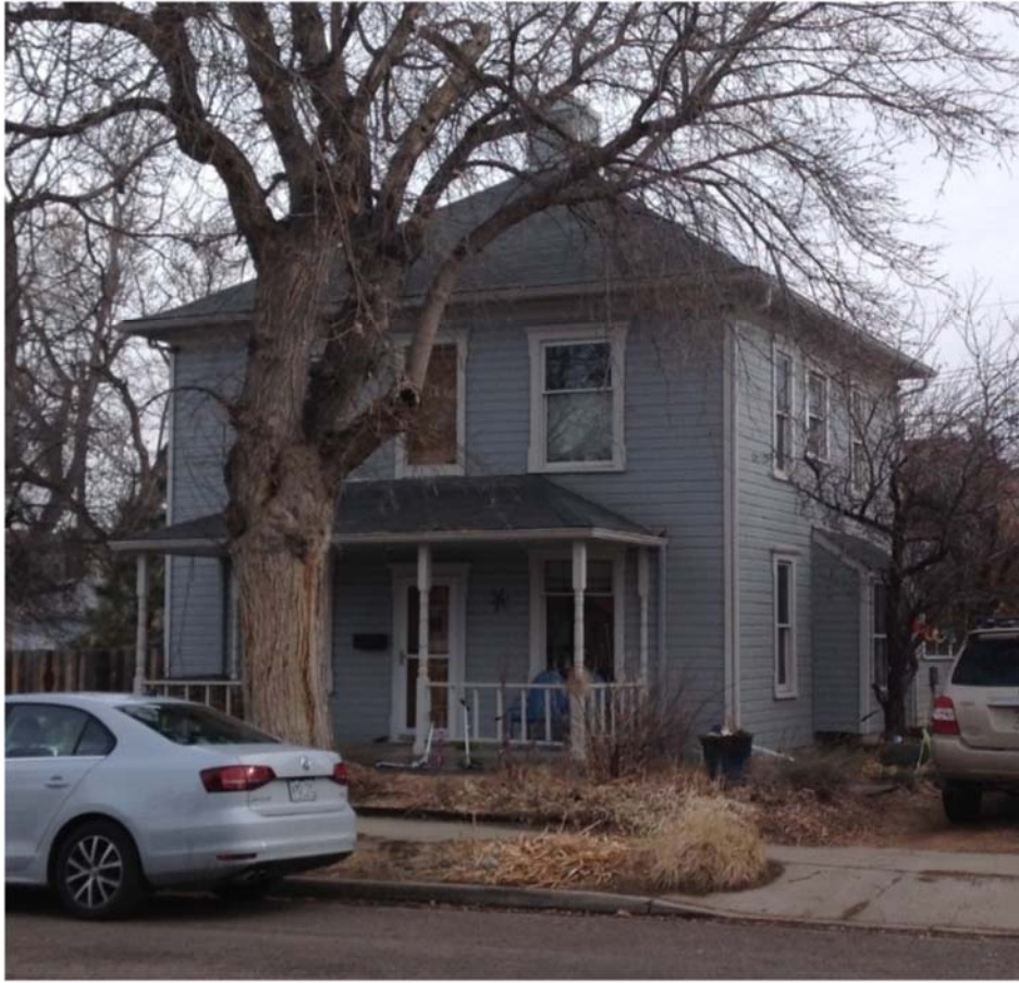
Figure B.23. 728 La Farge Avenue.
