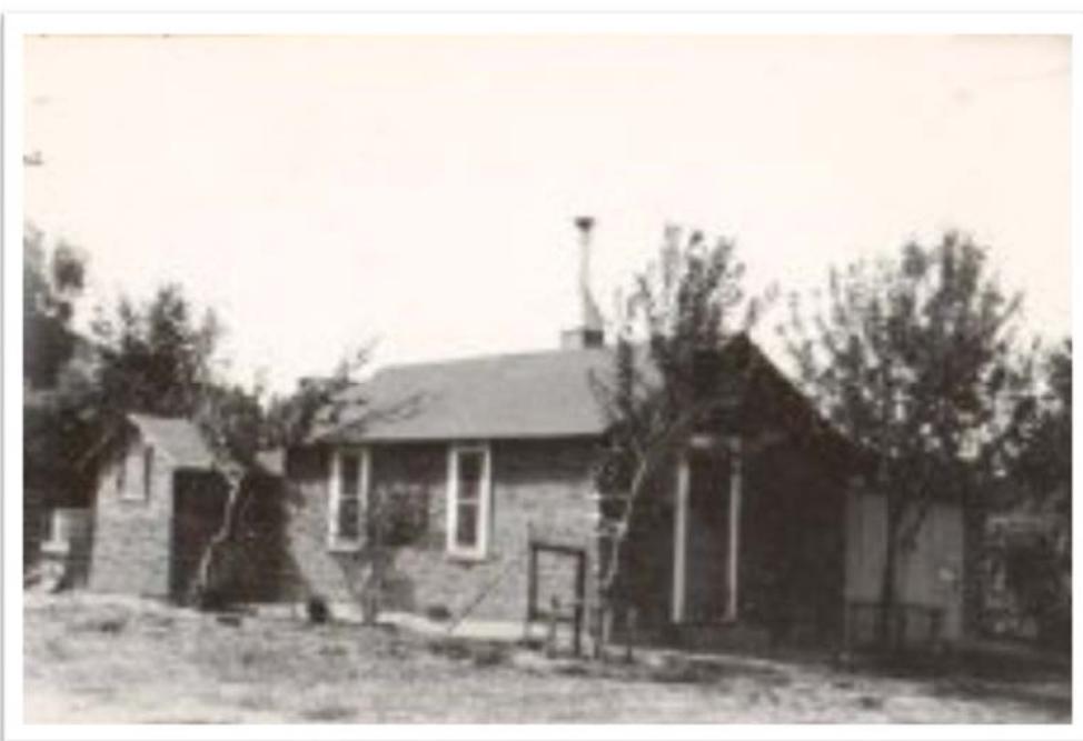
Figure 65. Assessor card photograph of 1131 Spruce Street in 1948 (LHM 2017).
