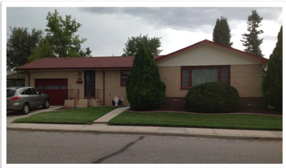
Figure B.49. 741 West Street.
