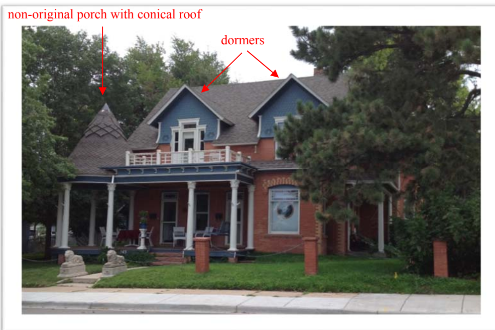
Figure 110. 1045 La Farge Avenue today, front view.
