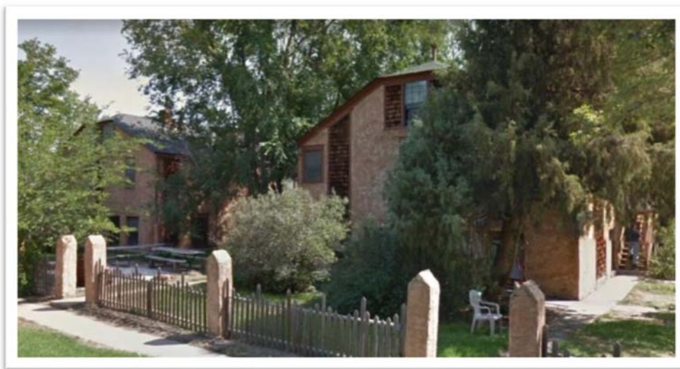
Figure 58. Former Louisville High School now remodeled into two apartment buildings.
