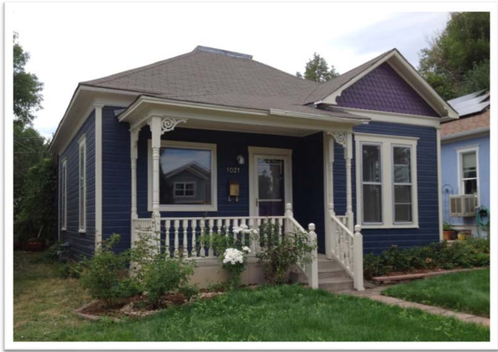
Figure B.15. 1021 La Farge Avenue.
