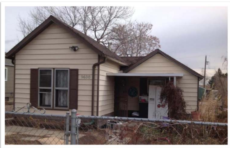
Figure 32. 1436 Cannon Street prior to recent demolition.
