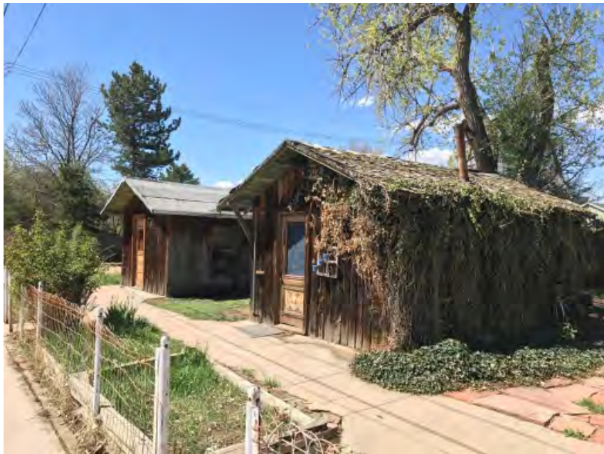
Picture 15 – View of both cabins, 801 is in the background and 809 is in the foreground.
