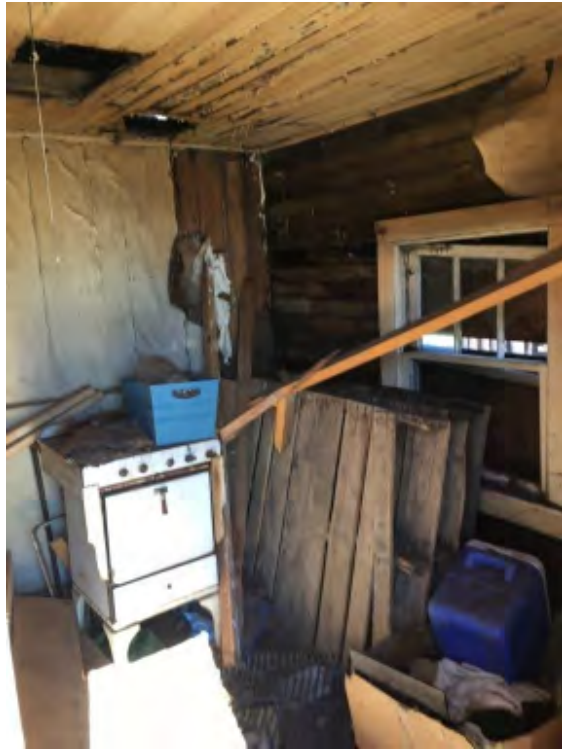
Picture 23 – View of front room. Gas stone in the corner, located to the back of the front room to the north side. Note ceiling is beaded board, nailed to rough-sawn 2x4 ceiling joists.
