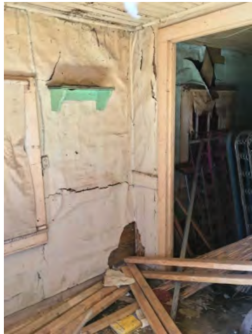
Picture 24 – View of the southwest corner of the front room, walls were covered in a wall paper. Note window casing, all the windows and door were cased and the casing was painted.
