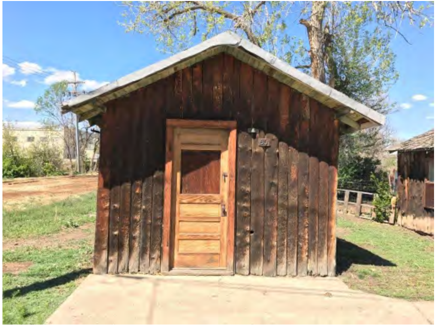
Picture 4 – East elevation of Cabin 801.
