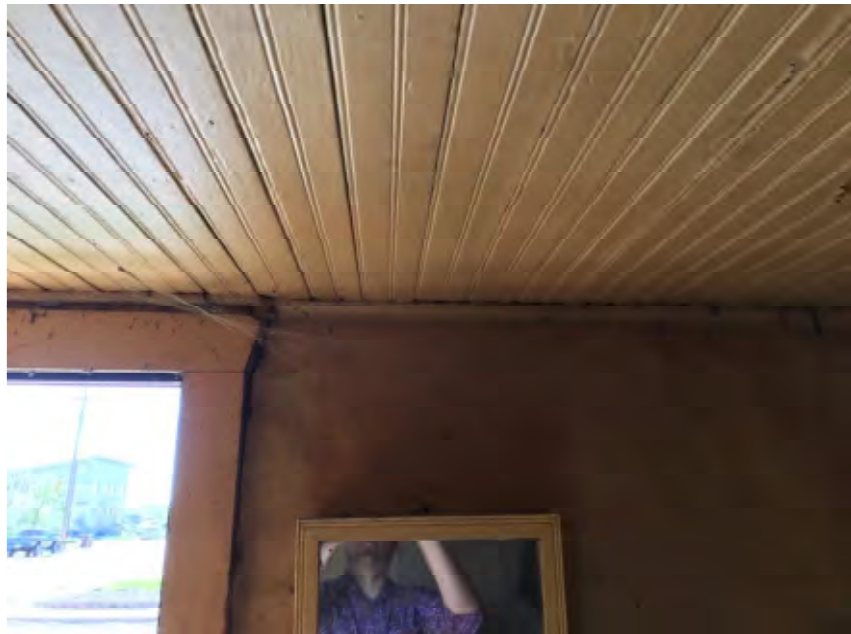
Picture 26 – Ceiling treatment. T&G beaded board. Also note the casing around the entry door, 1x4 pine casing.
