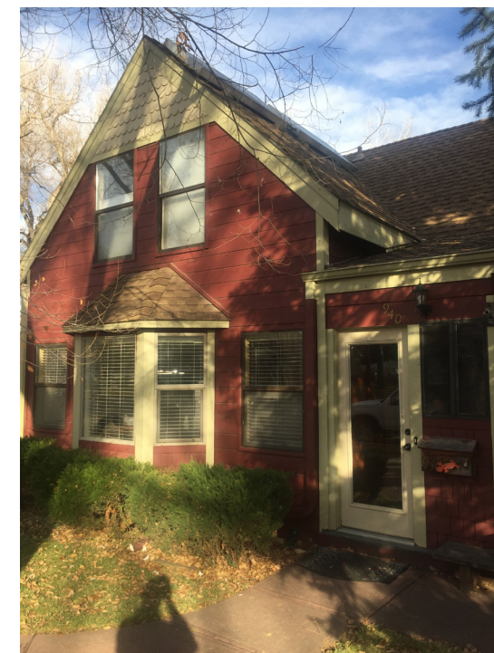
View of front of home
