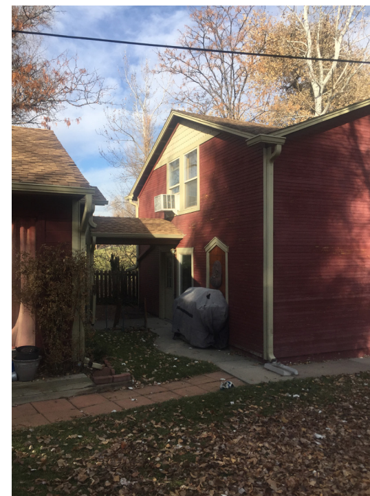
View of covered breezeway connection
