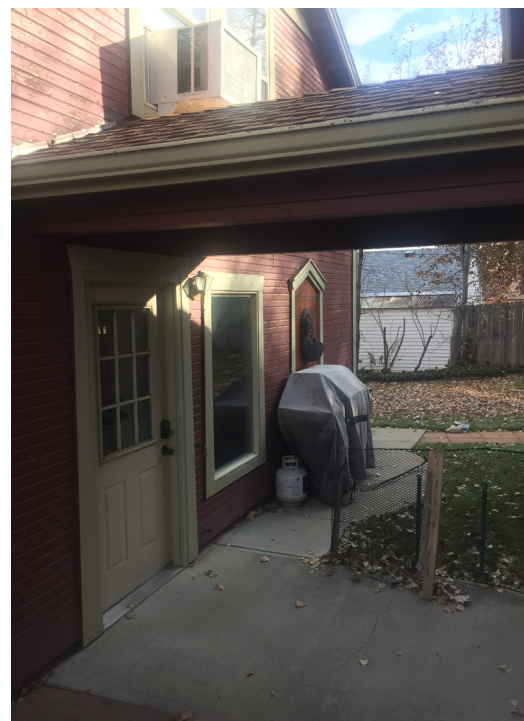
View of covered breezeway at Garage
