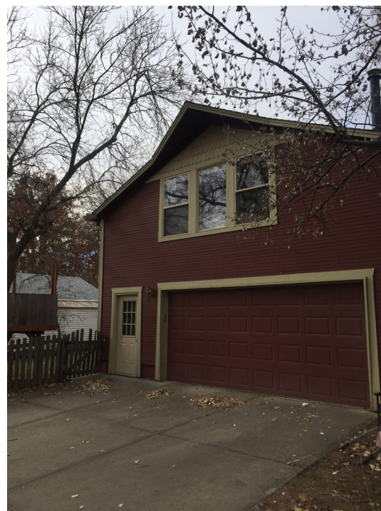
View of Garage from rear alley
