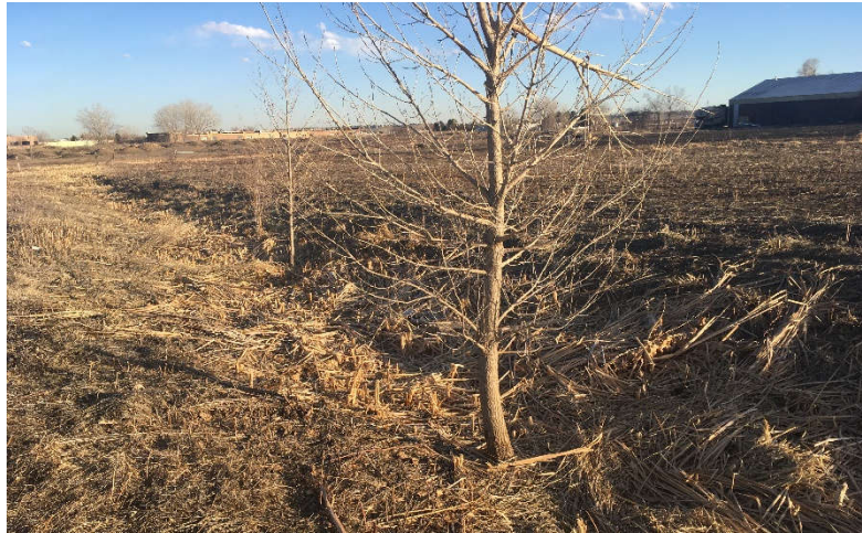
Description: Stormwater Outfall Channel View Direction: East
