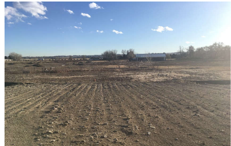
Description: General Site View View Direction: South
