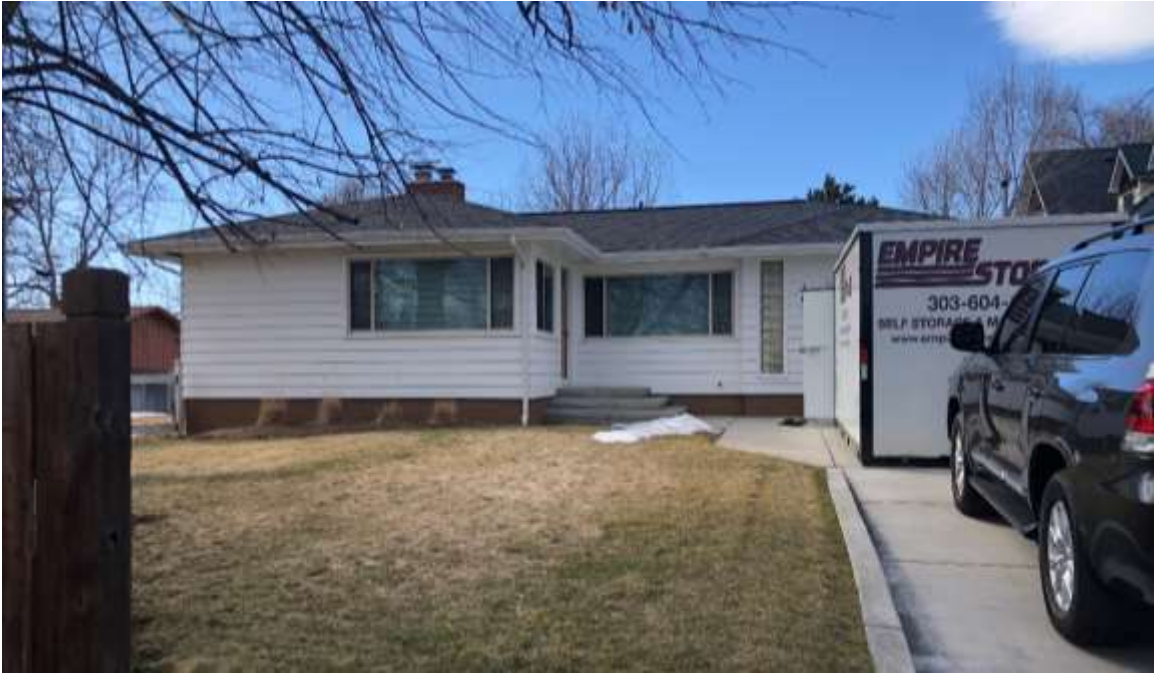
105 Roosevelt Avenue. East view, 2020.
