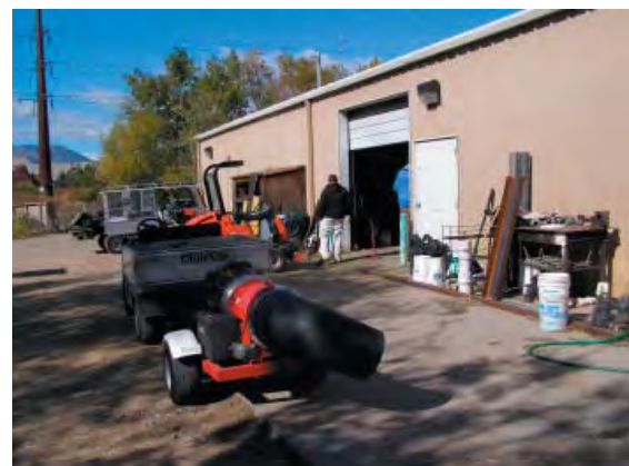
Maintenance facility is undersized to accommodate equipment storage.
