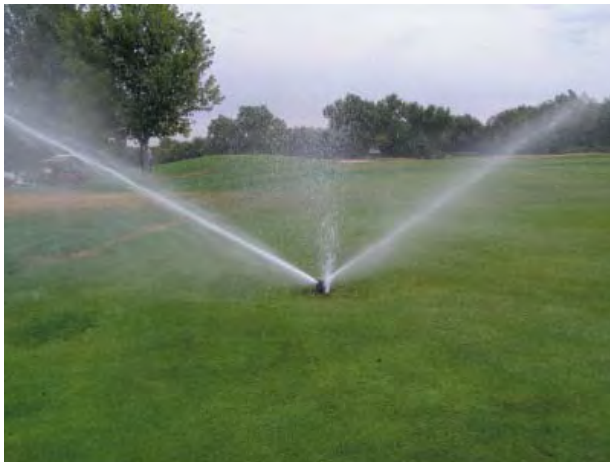
Leaking irrigation head.
