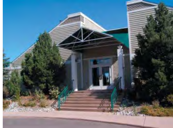
Clubhouse main entrance is overgrown & dated.
