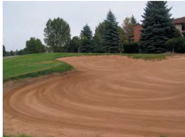
Collapsing bunker face & contaminated sand.
