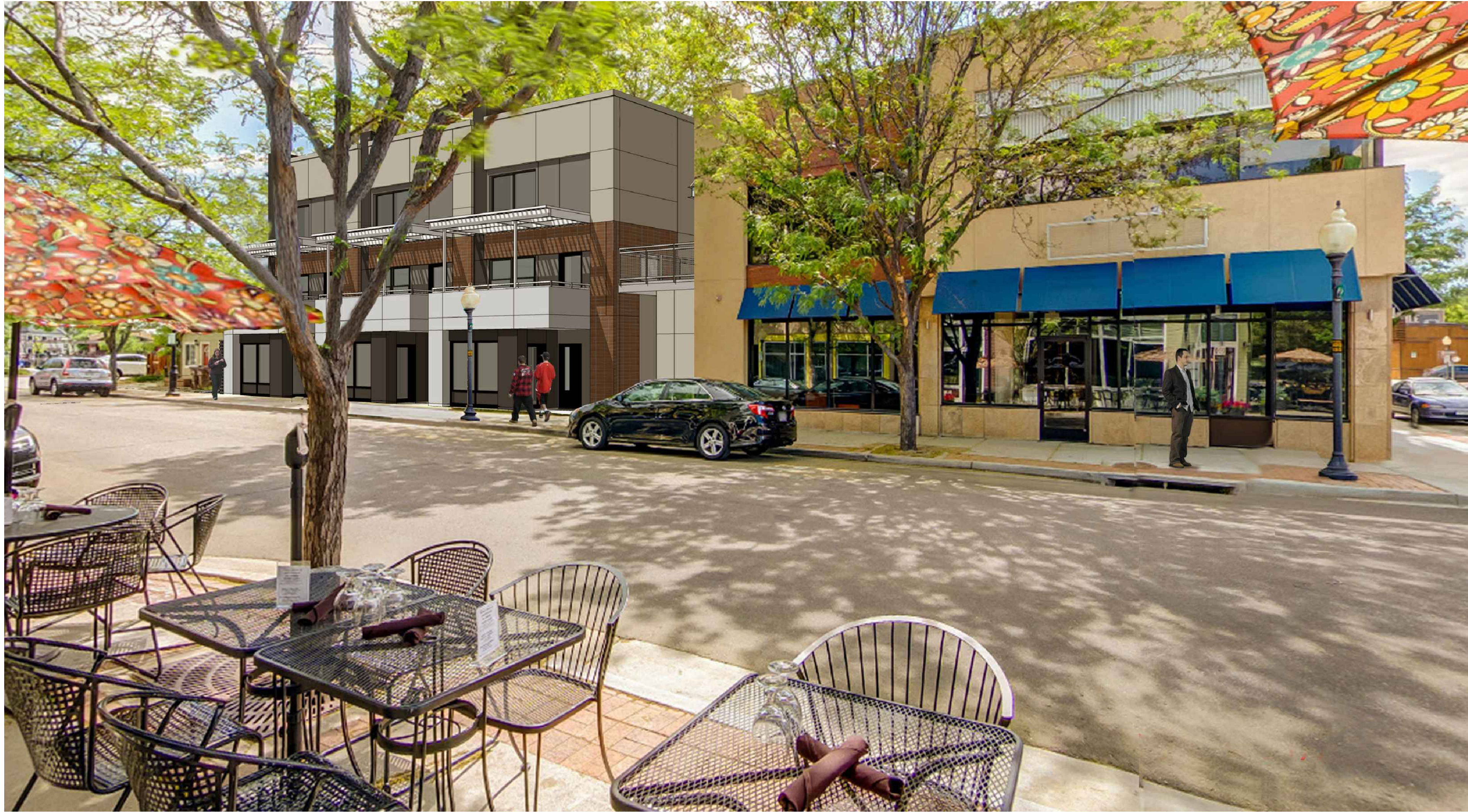
STREET VIEW FROM THE NORTHEAST
