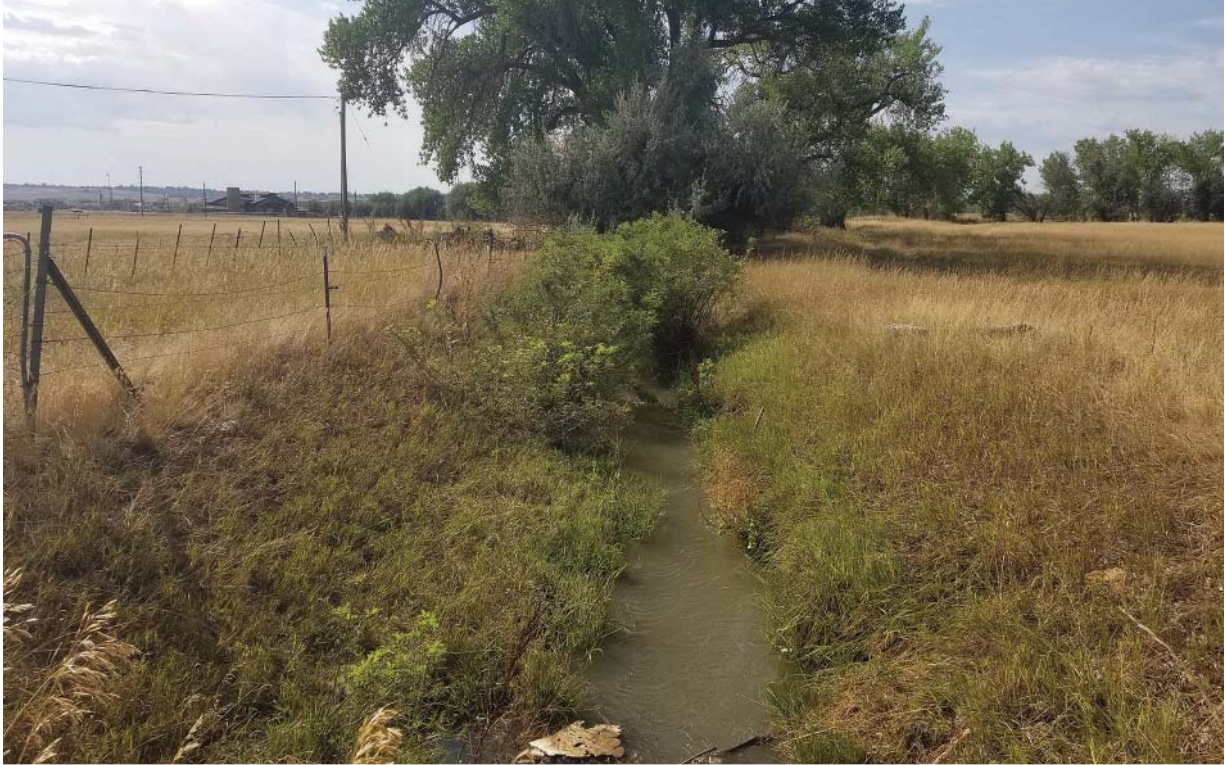
Photo 1 - Overview of Goodhue Ditch. View is to the southeast.
