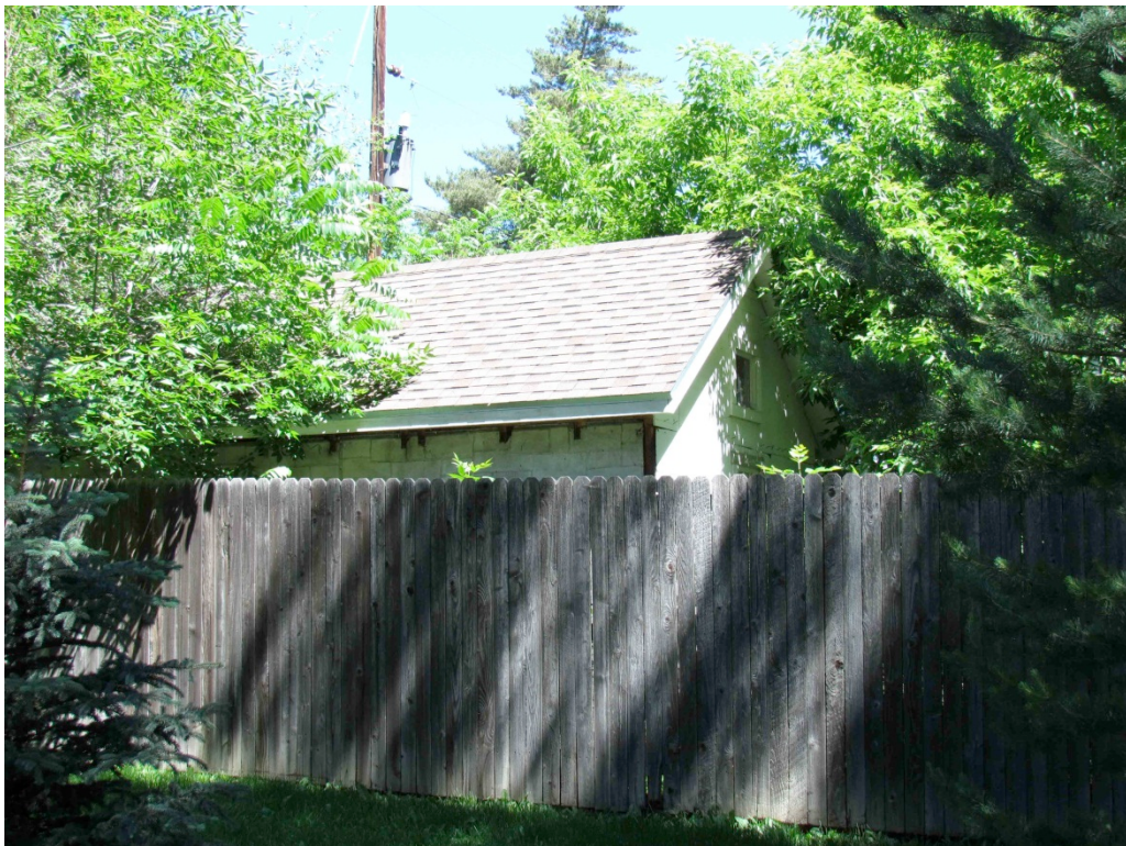
5BL11305_833Jefferson_04 outbuilding southwest
