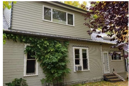
Variety of windows on the south side
