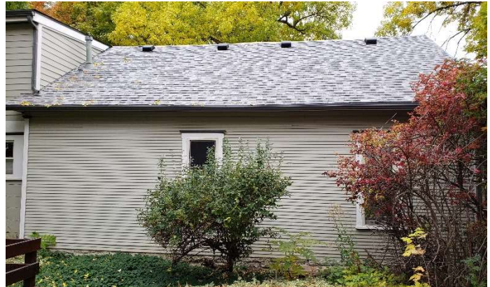
North side asphalt composite shingle roof and mushroom vents near the ridge
