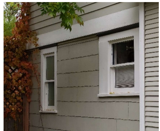
North side windows in kitchen and bath
