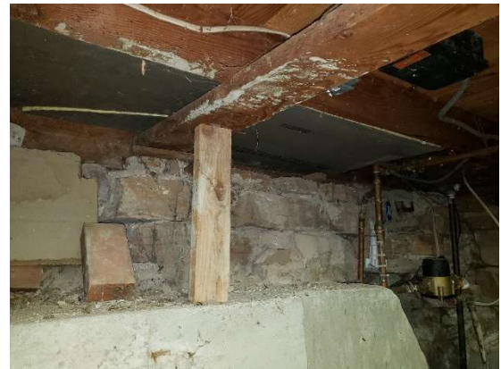
Flat 2x6 beam & 2x4 column
