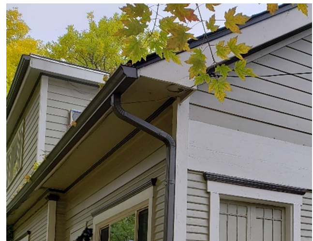
Soffit transition at southeast corner of house
