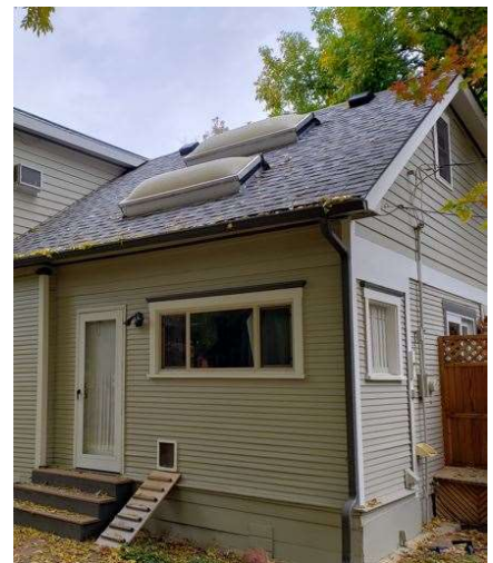
Curb mounted skylights on south side
