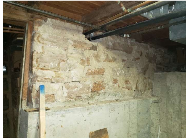
Concrete foundation added beneath original stone foundation. Concrete retaining wall between the basement and crawlspace is seen on the right.
