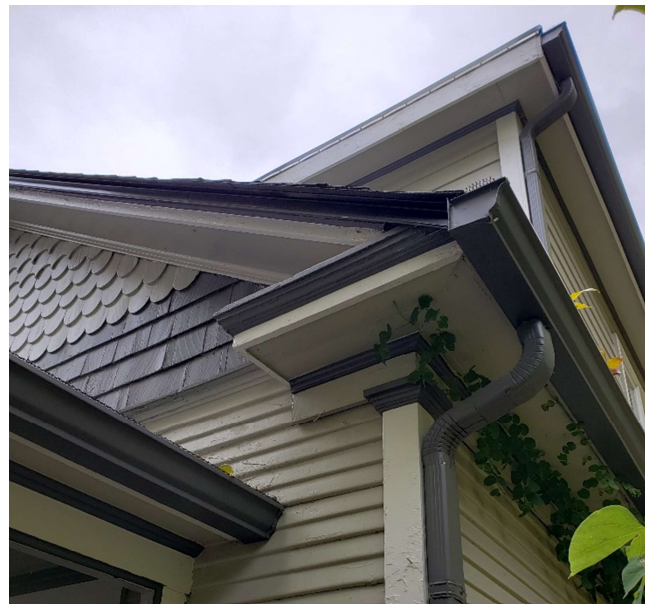
Varieties of soffits & fascia on southwest corner of house
