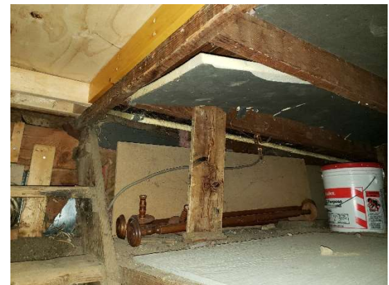
South deck (now enclosed) floor framing & support
