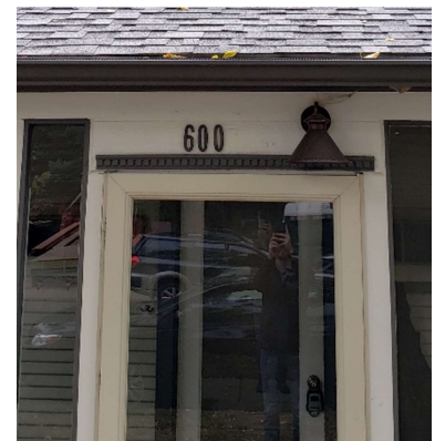
Wall sconce at sunroom door
