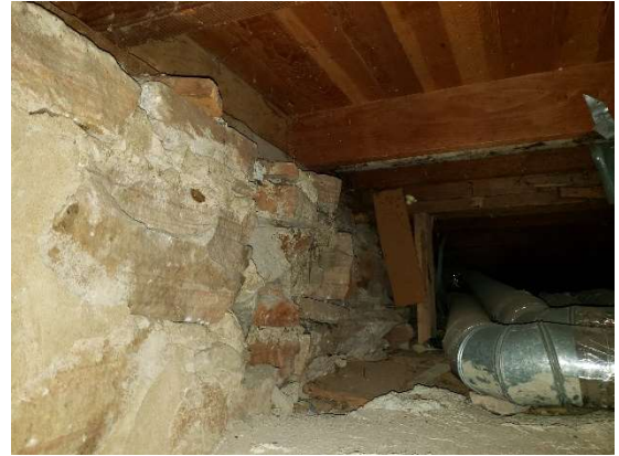
Original floor framing, sheathing, sill plate, and floor bracing
