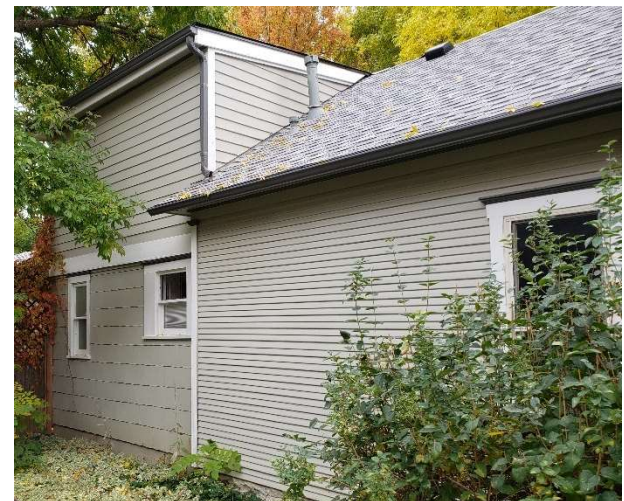
The gable on the north stops at the second floor addition. The second floor has a low sloped shed roof.
