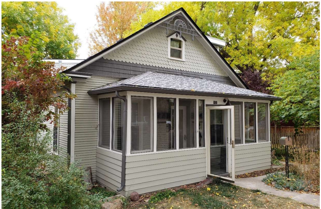
2021 photograph from the northwest
