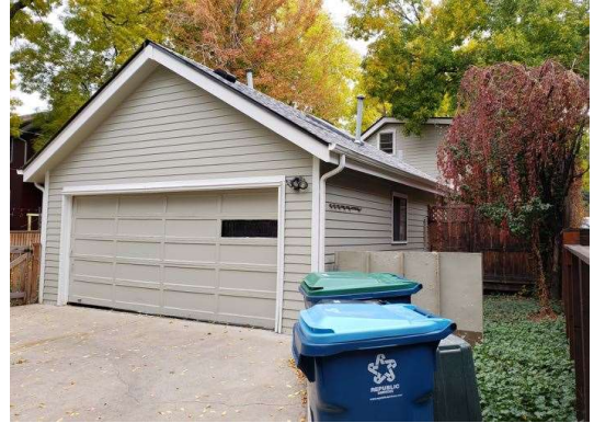
Garage view from the alley
