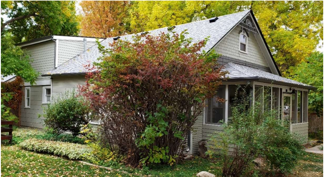
2021 photograph from the northwest
