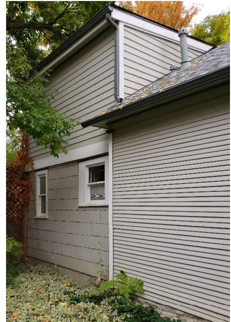
Clapboard siding, lap siding, and composite siding on north side of the house
