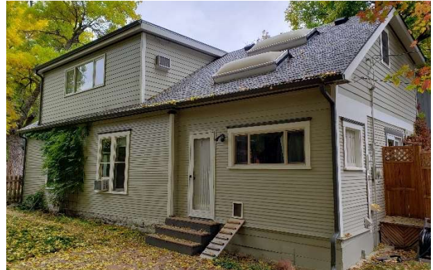
The gable roof form carries from front to back on the south side with the south dormer projecting out. There is a slight change in roof plane aligned with the main floor transition.
