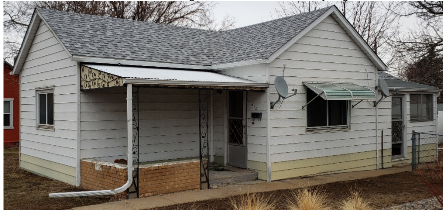
Asphalt composite shingle roof on main house, corrugated metal roof at the covered front porch.
