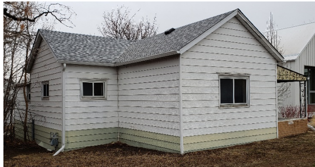
Grading around the building footprint is apparent in how the siding is tapered where it meets grade.
