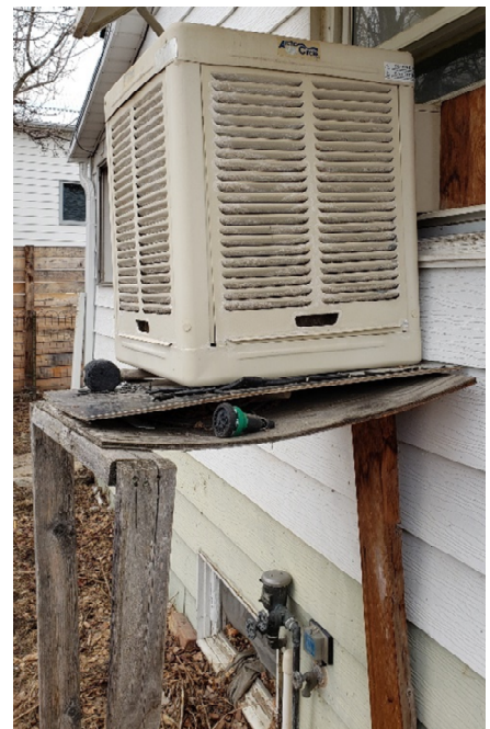
Window mounted air conditioning unit and makeshift support structure located at east facing kitchen window.
