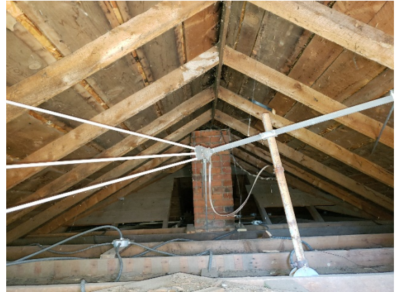
East facing gable roof structure with north-south gable structure beyond. Chimney remnants found in attic space are not present on the main floor nor protruding through the roof.
