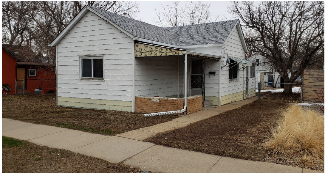
Looking northeast. The house sits on the west end of the lot, close to the ROW without any planting on the west side of the lot.
