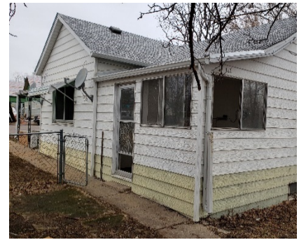
Grading around the building footprint is apparent in how the siding is tapered where it meets grade.
