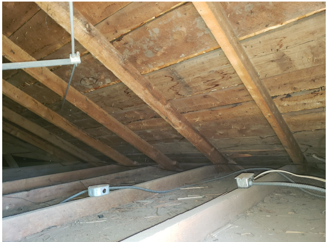
Roof framing as observed from east gable end access.
