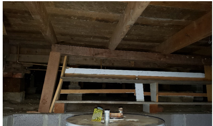
Floor framing, sheathing, & supports
