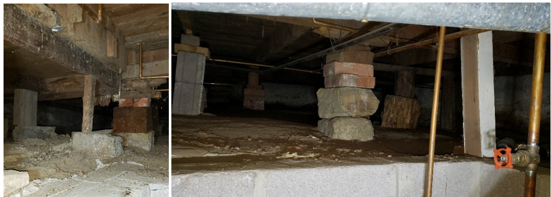
Various flooring structure support-beams & built-up columns
