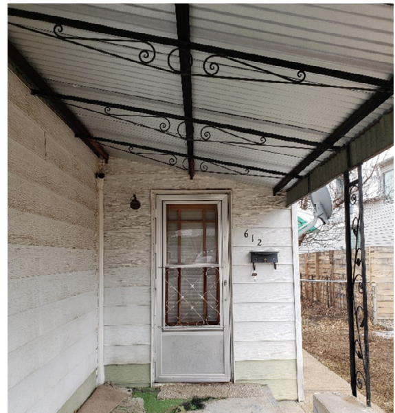
Covered front porch steel structure.
