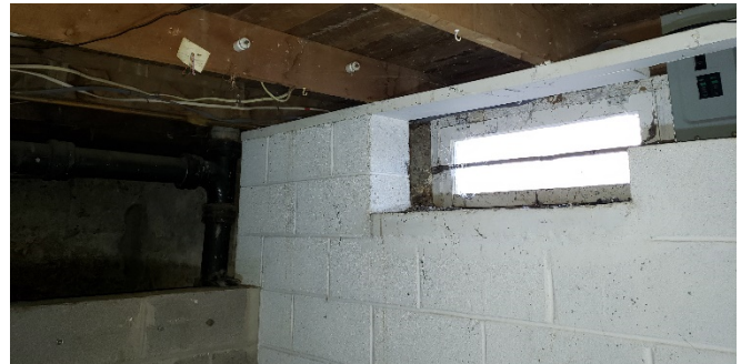
CMU walls in basement. The east wall runs to the bottom of floor joists and is capped with a 2x sill plate.
