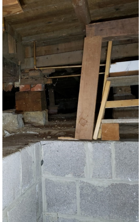
CMU walls between basement and crawlspace.
