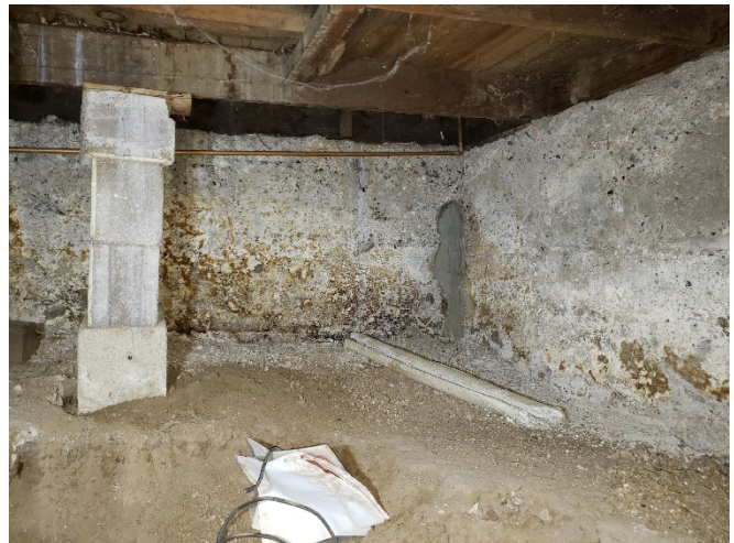
Concrete foundation in northeast corner of crawlspace.
