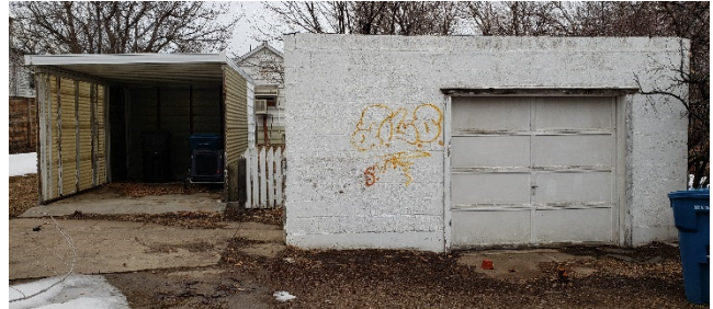
Garage and carport facing the east alley
