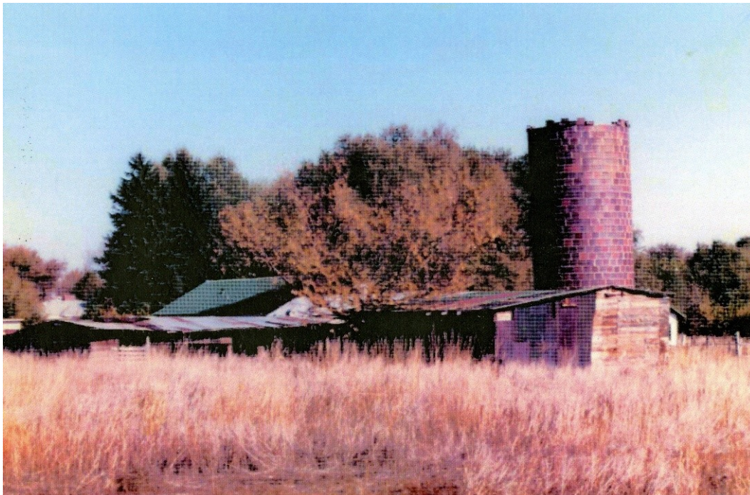
facing northeast (Photograph on file with the Louisville Historical Museum).
