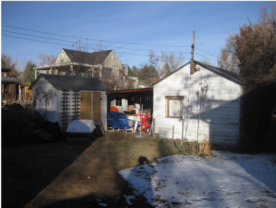
Figure 26. 109 W. Spruce outhouse / coal shed, storage area, shed 3, west and south sides, facing northeast.
