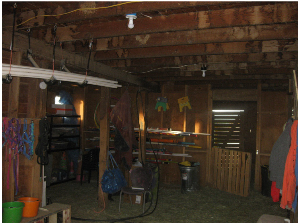
Figure 9. 10433 Dillon barn interior, facing north.
