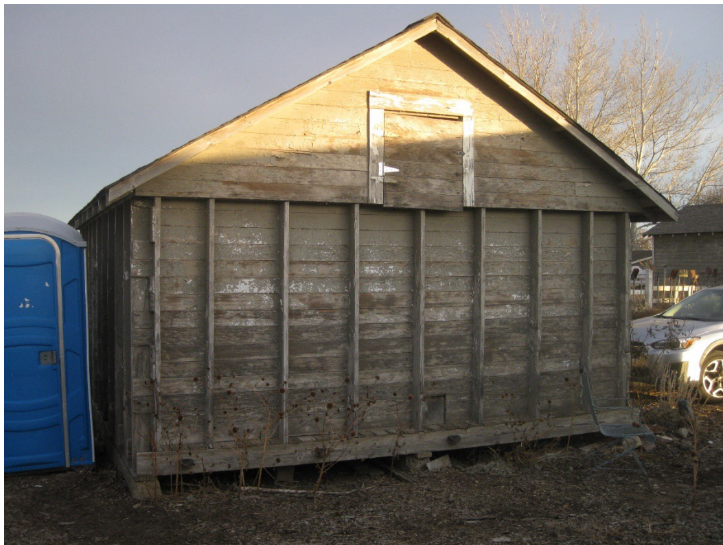
Figure 26. 10433 Dillon granary 2, west side, facing east-southeast.
