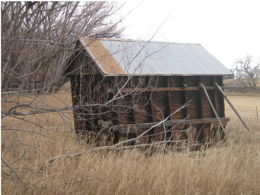
Figure 26. 151 County tack shed, north and west sides, facing southeast.
