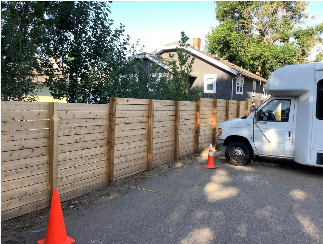
Figure 6. 920 Lincoln, back of house, facing southwest.
