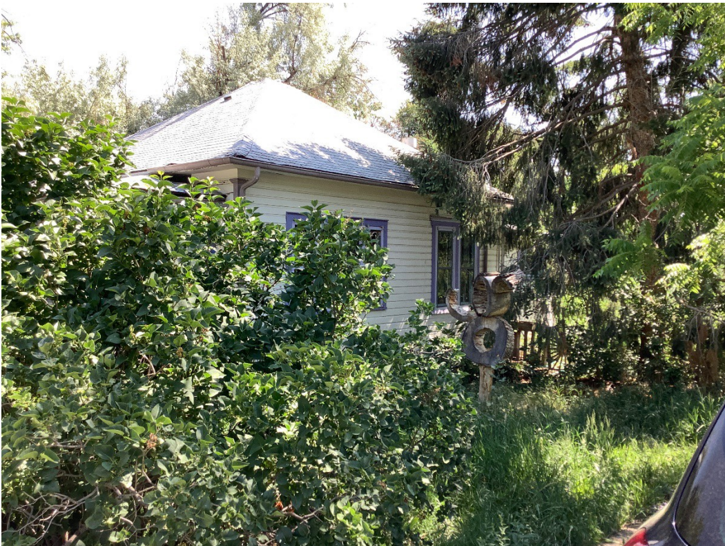
Figure 4. 600 Grant, facing northwest.
