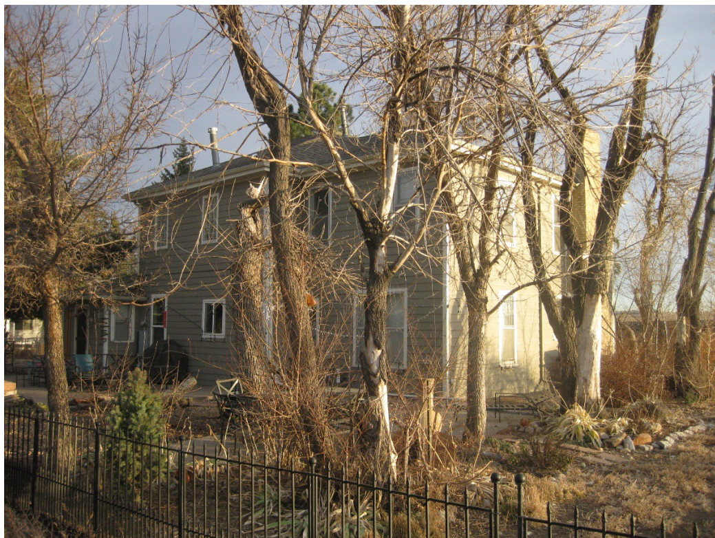
Figure 3. 10433 Dillon house, north and west sides, facing southeast.
