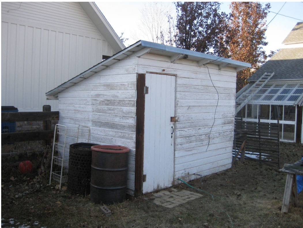
Figure 14. 109 W. Spruce shed 2, south and east sides, facing northwest.
