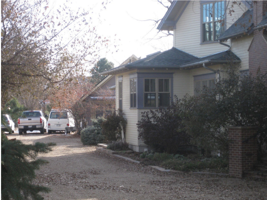
Figure 5. 310 W. Spruce garage, north side, and house, east side, facing south- southwest.
