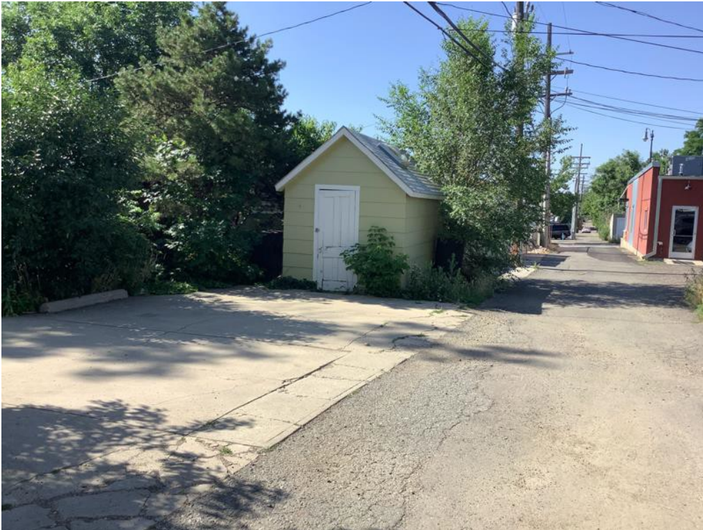
Figure 7. 921 Main, Outbuilding – Shed, facing south-southwest
