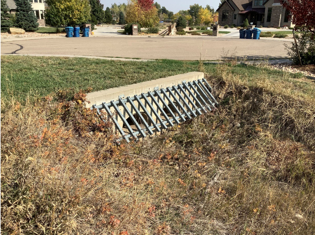
Figure 11. 5BL9577.2 concrete headwall with metal grate, facing north, M. Taylor, 10/8/2020.
