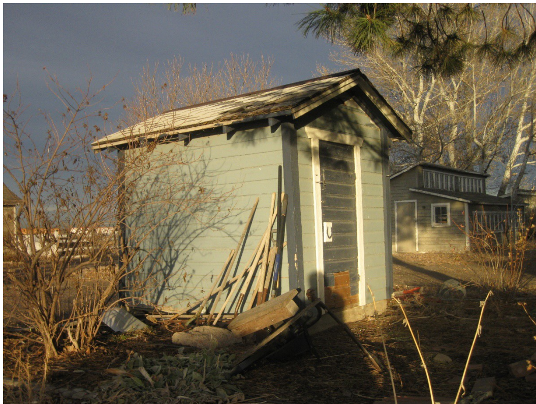
Figure 18. 10433 Dillon small outbuilding, west and south sides, facing northeast.
