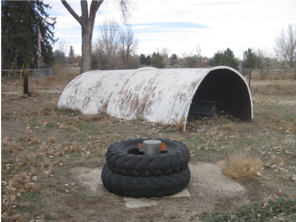
Figure 23. 151 County semi-cylindrical storage, south side, facing north.
