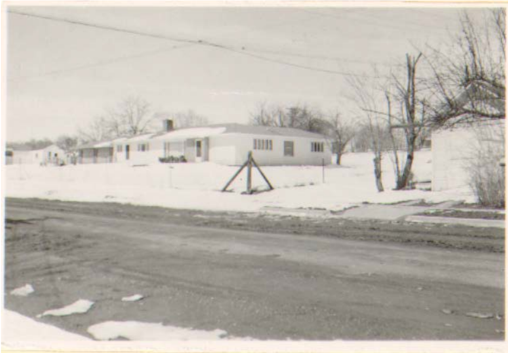
Figure 9. 101 W. Spruce photo from ca. 1964 assessor card, south and east sides, facing northwest (LHM 2017).
