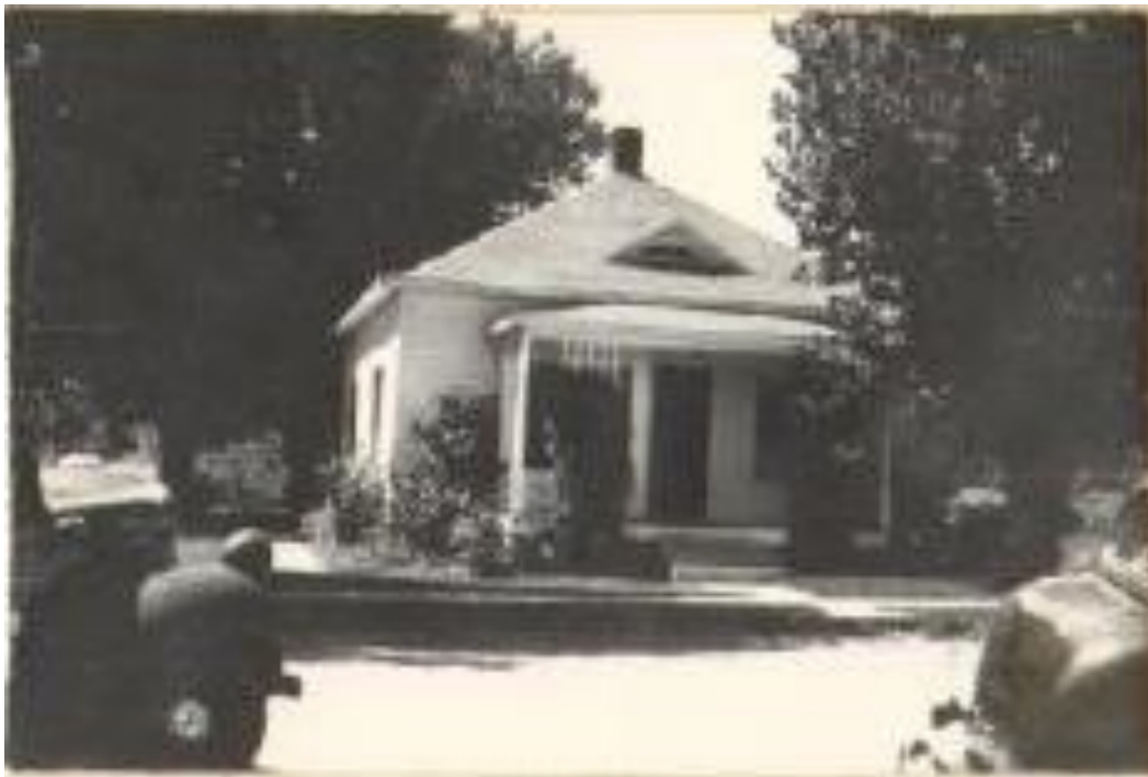
Figure 7. 933 Lincoln photo from 1948 Assessor Card, south and east sides, facing northwest (LHM 2017).
