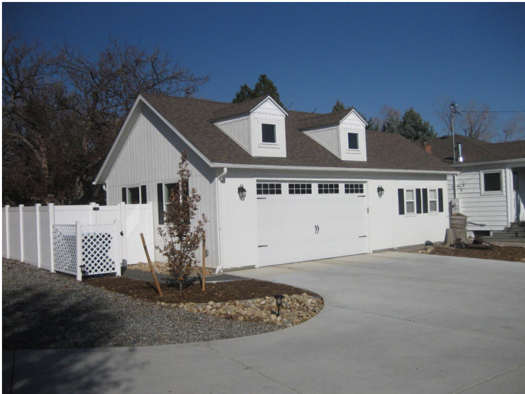
Figure 8. 1515 Main garage, west and south sides, facing northeast.
