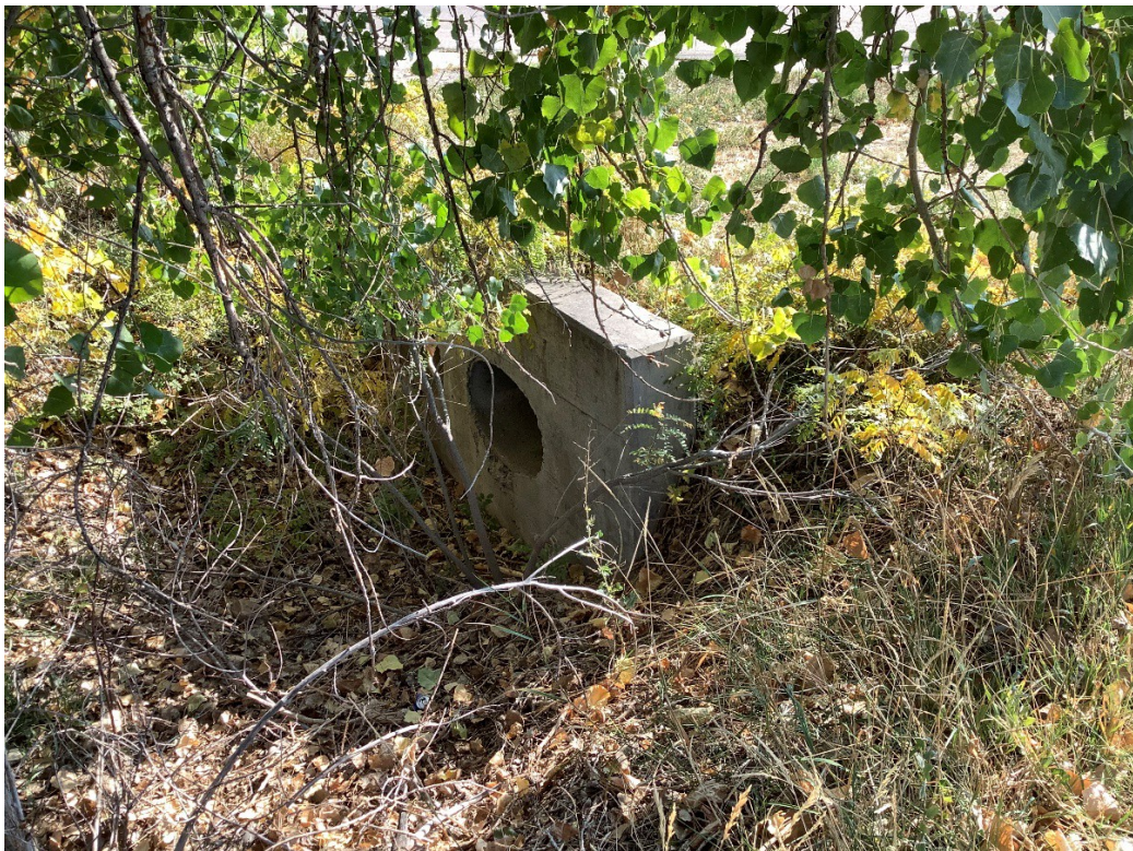
Figure 10. 5BL9577.2 double concrete culvert, facing east, M. Taylor, 10/8/2020.
