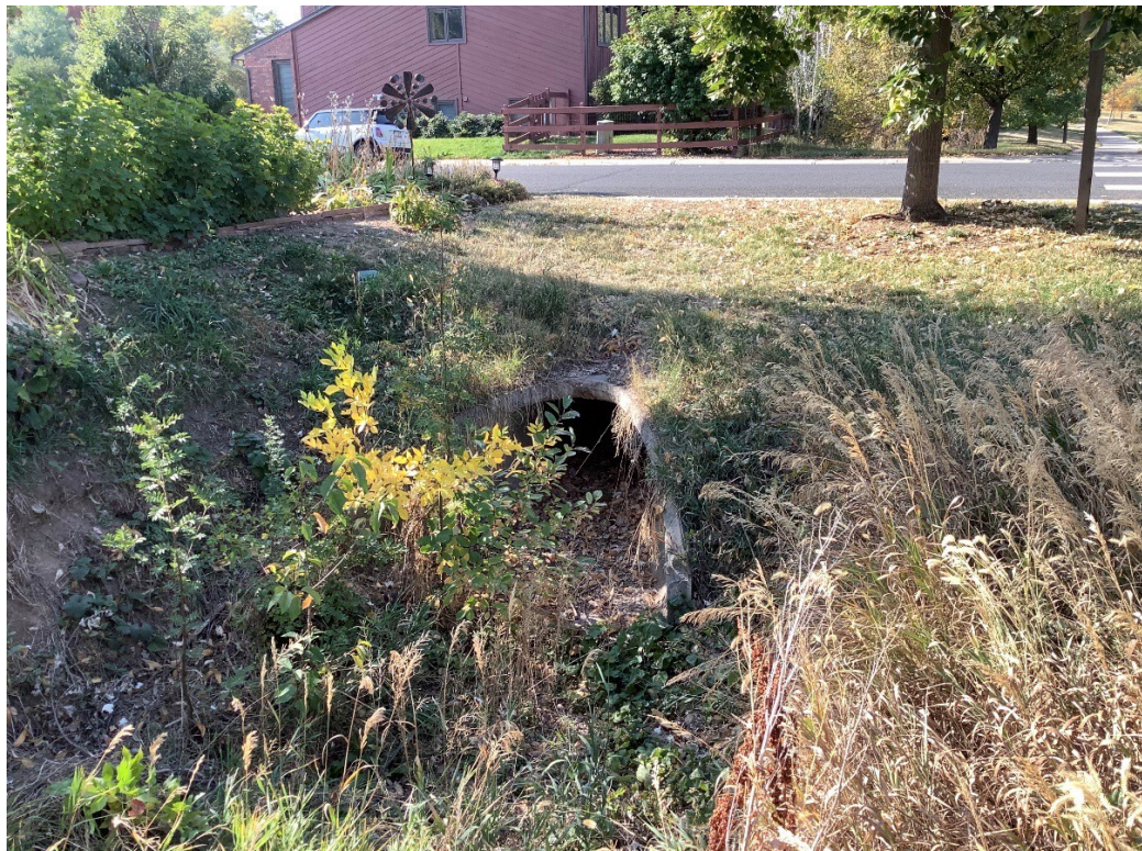
Figure 5. 5BL9577.2 concrete u-culvert, facing south, M.Taylor, 10/8/2020.
