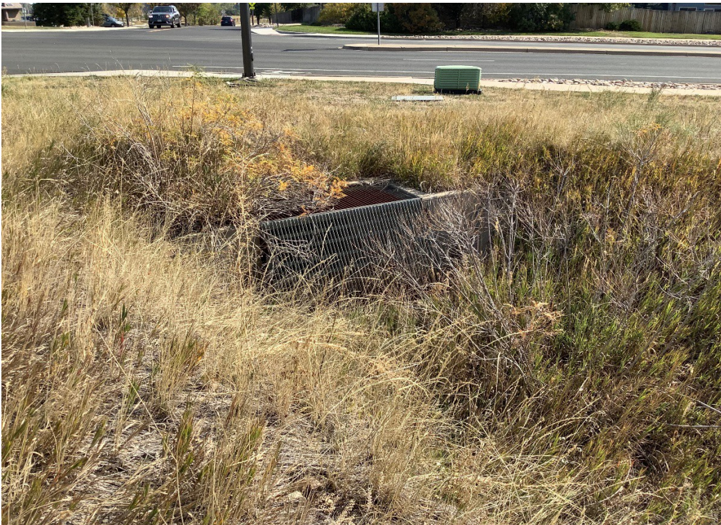
Figure 14. 5BL9577.2 concrete box culvert on west side of McCaslin Boulevard, facing east, M. Taylor 8/12/2020.
