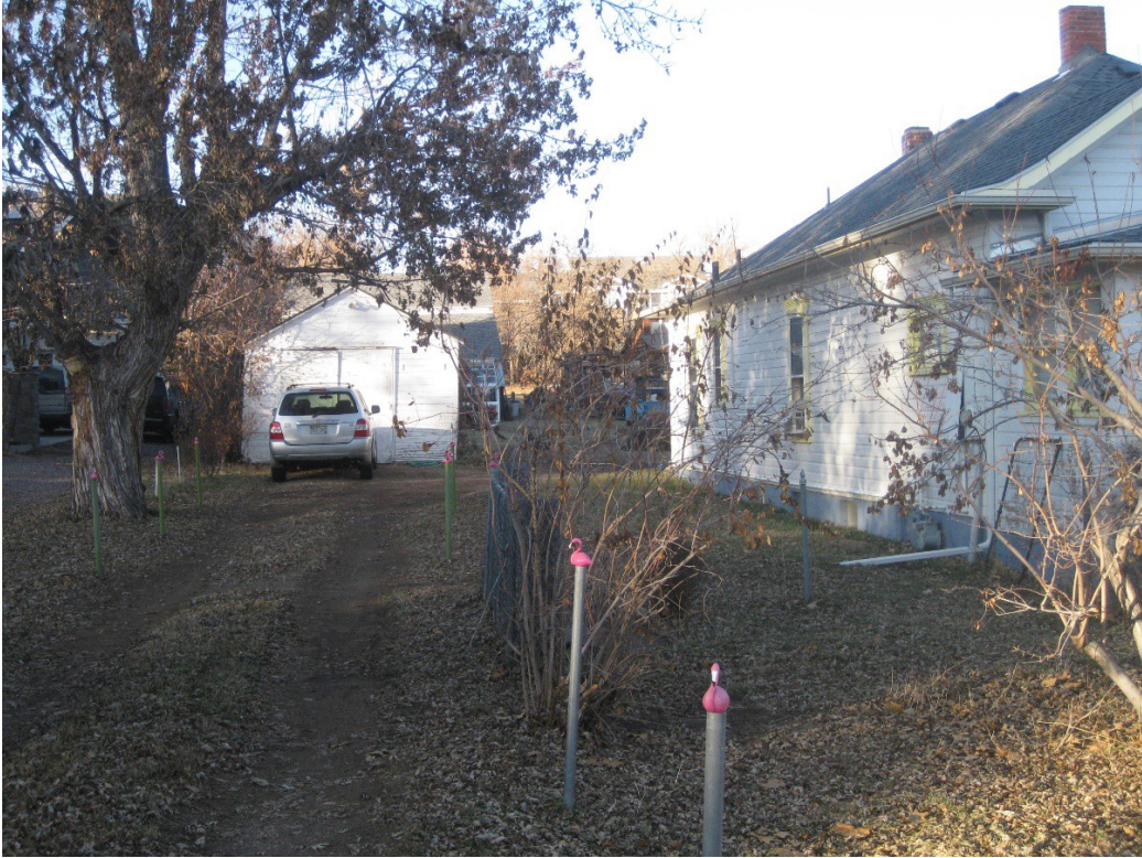
Figure 7. 109 W. Spruce garage and house, south and west sides, facing north.
