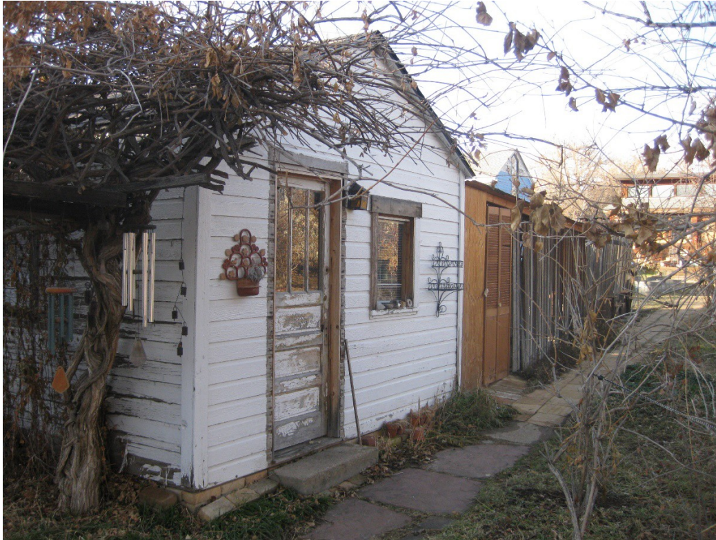
Figure 29. 109 W. Spruce shed 3 and storage area, east and south sides, facing northwest.
