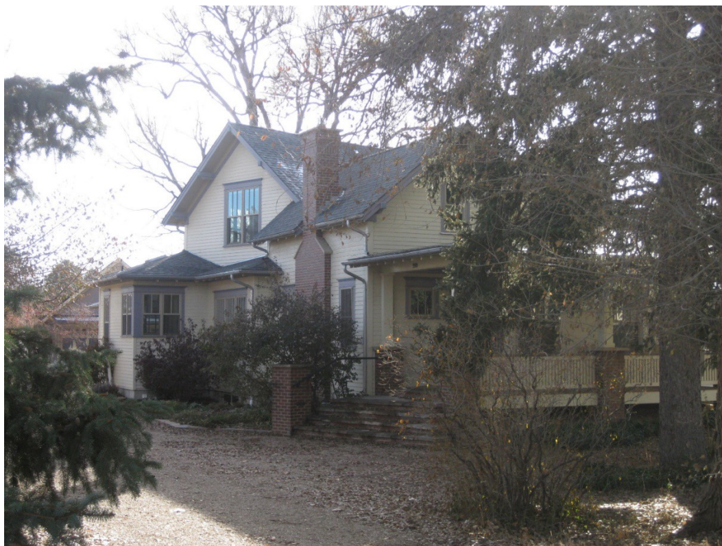
Figure 4. 310 W. Spruce house, east side, facing southwest.
