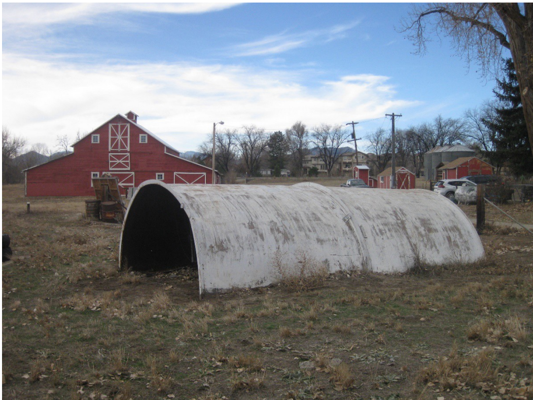
Figure 24. 151 County semi-cylindrical storage, east side, facing west.
