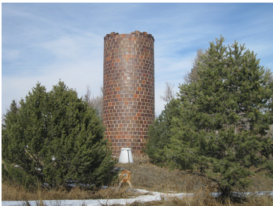
Figure 11. 310 W. Spruce silo, southwest side, facing northeast.
