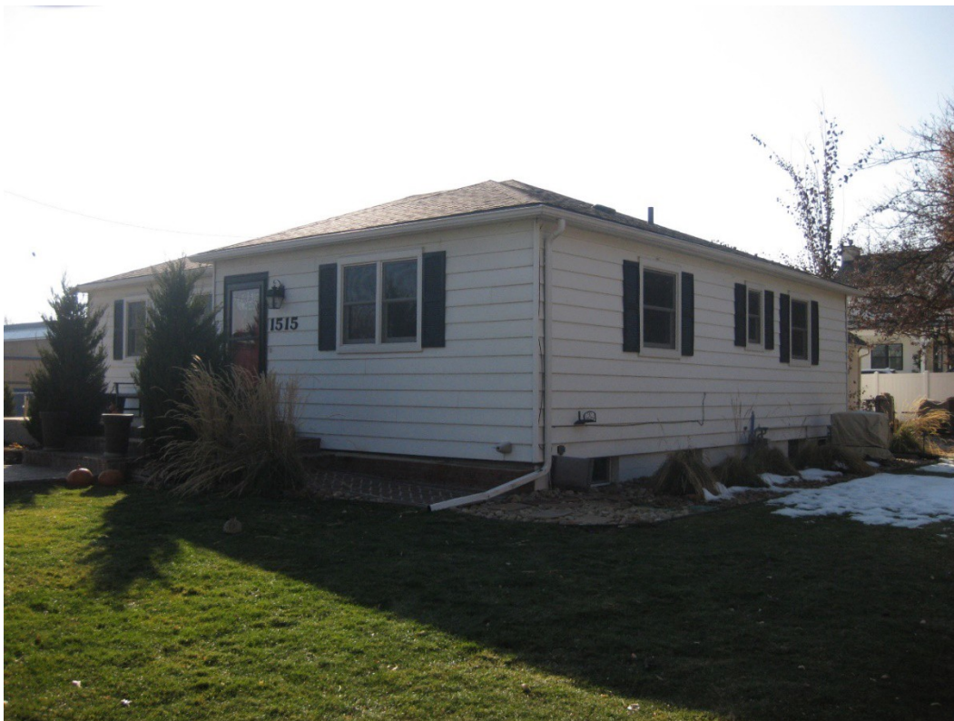
Figure 6. 1515 Main house, east and north sides, facing southwest.
