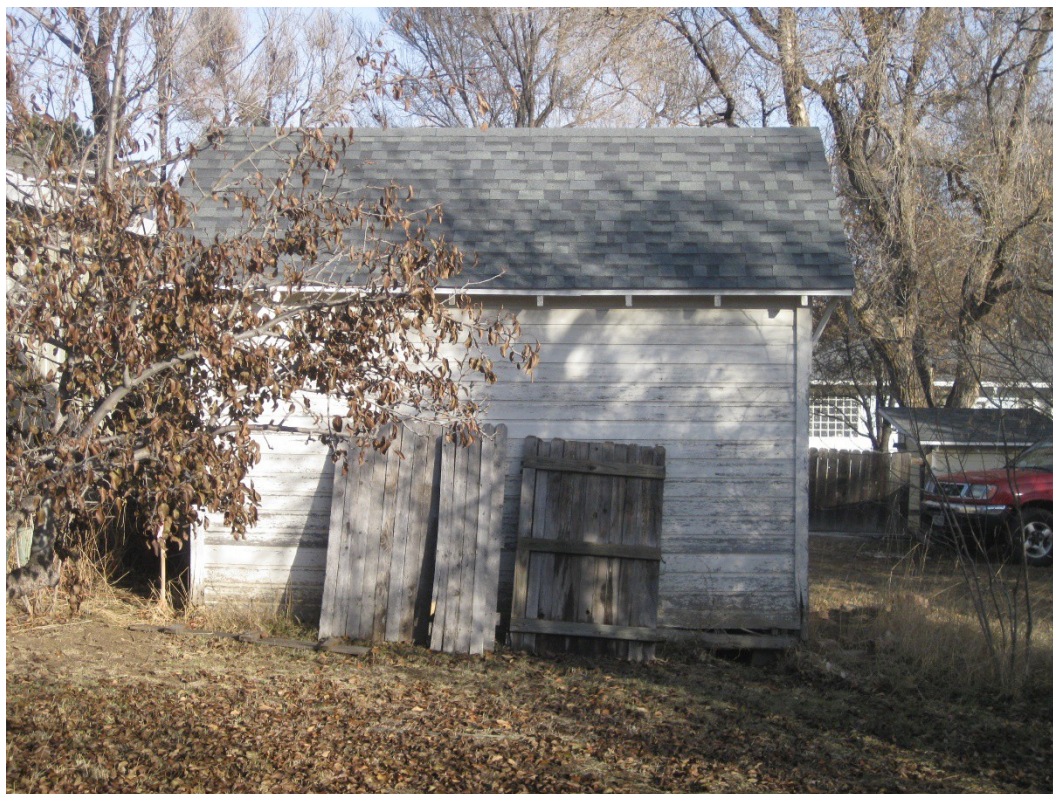
Figure 8. 101 W. Spruce early 1900s house, west side, facing east.
