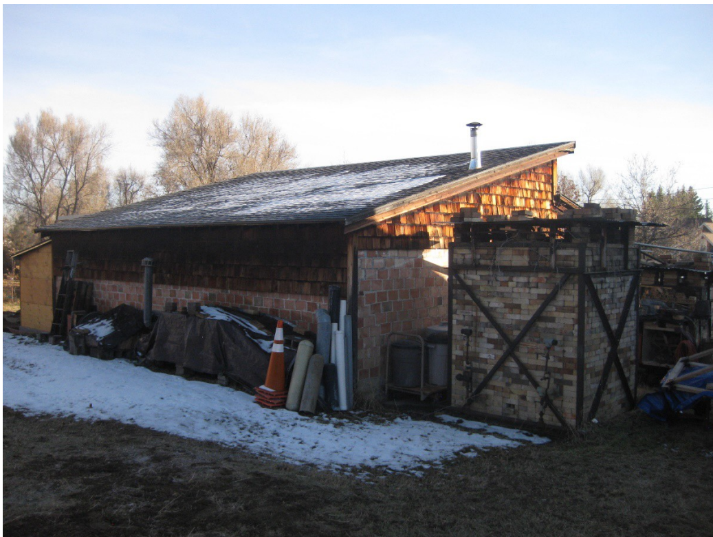
Figure 22. 109 W. Spruce coop and kiln, north and west sides, facing southeast.
