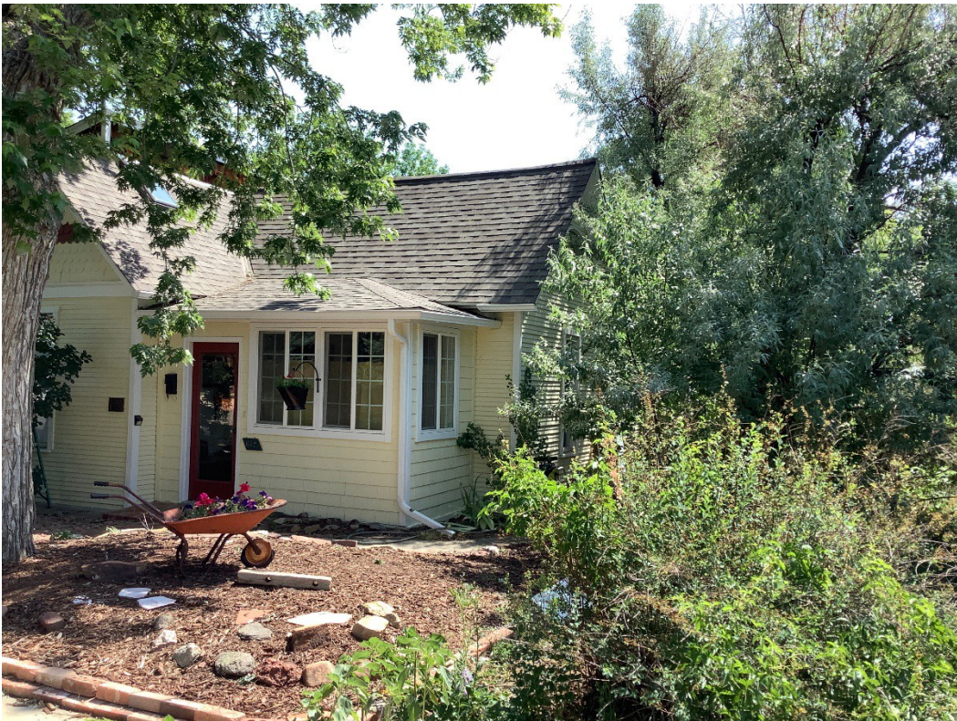
Figure 4. 612 Grant, facing northeast.
