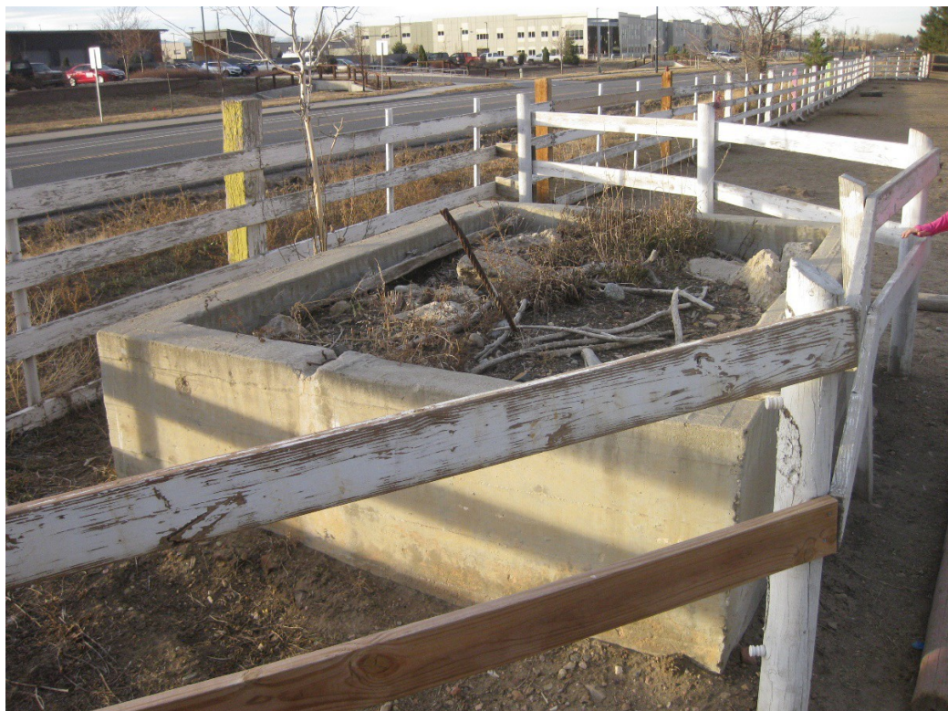
Figure 29. 10433 Dillon trough 1, south side, facing north-northeast.
