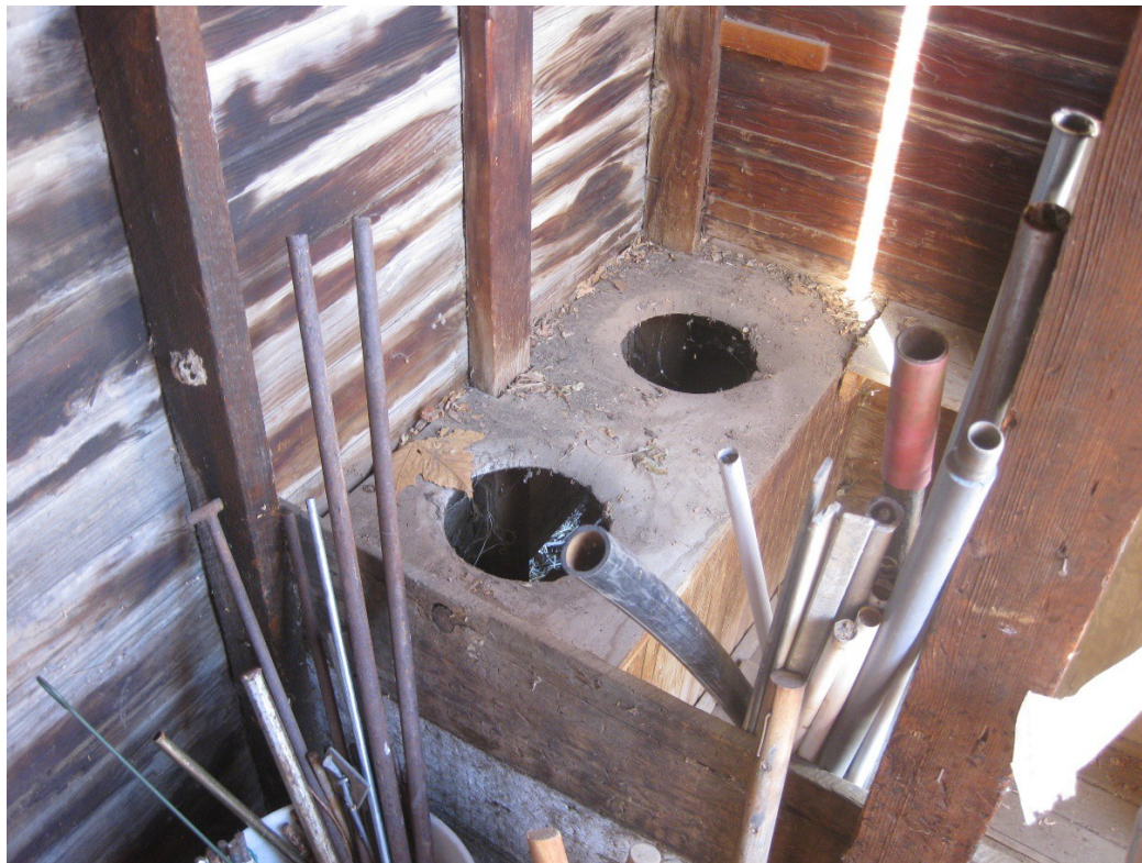
Figure 28. 109 W. Spruce outhouse/coal shed interior, north and east sides, facing northeast.
