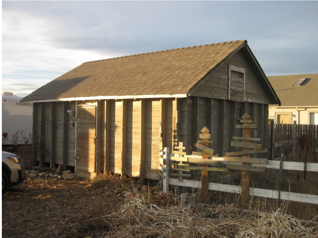
Figure 25. 10433 Dillon granary 2, south and east sides, facing northwest.
