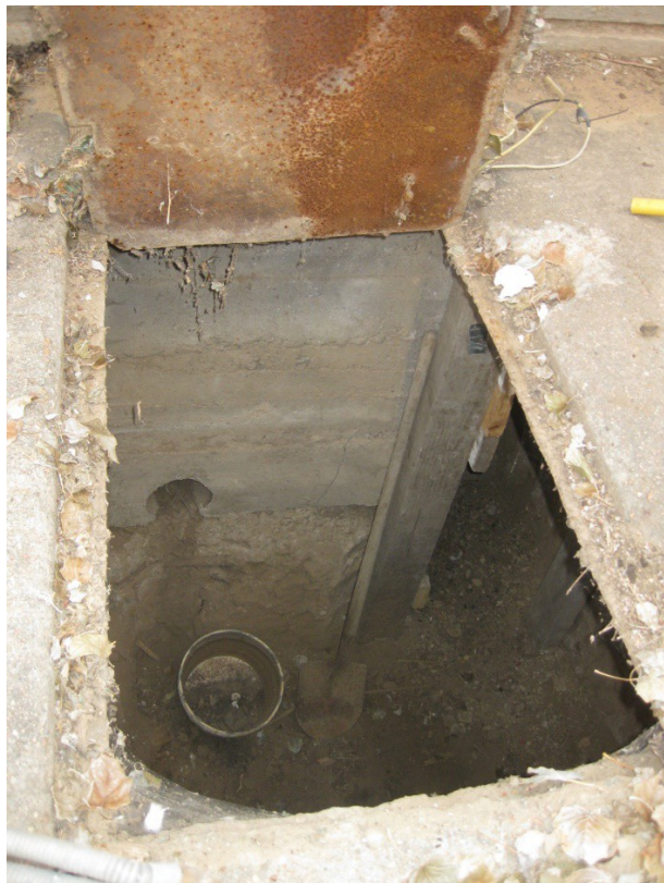
Figure 17. 10433 Dillon hatchery firepit interior, facing southeast.
