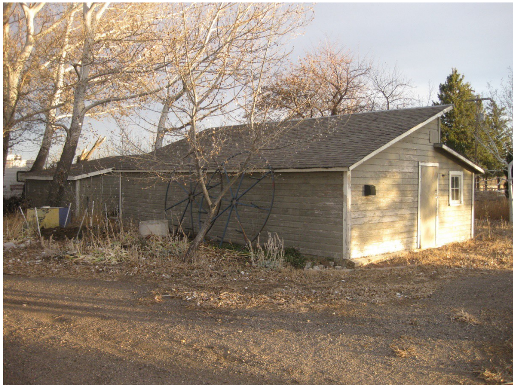
Figure 13. 10433 Dillon hatchery and coop, north and west sides, facing southeast.
