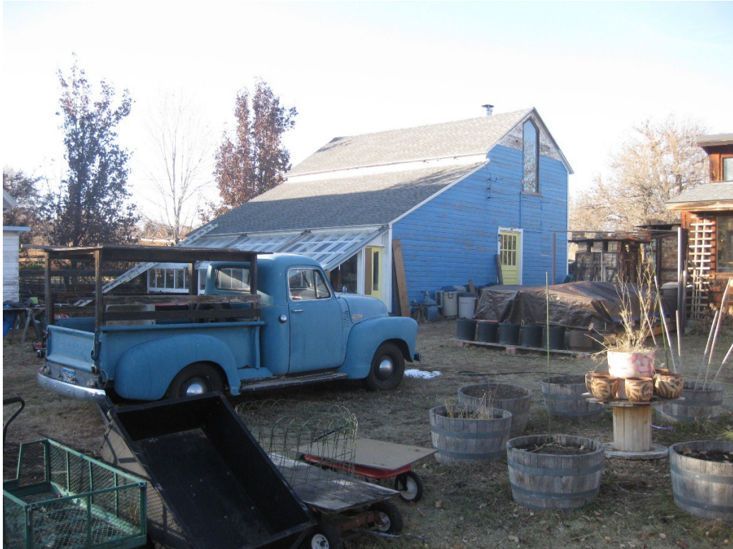
Figure 19. 109 W. Spruce barn, south and east sides, facing northwest.
