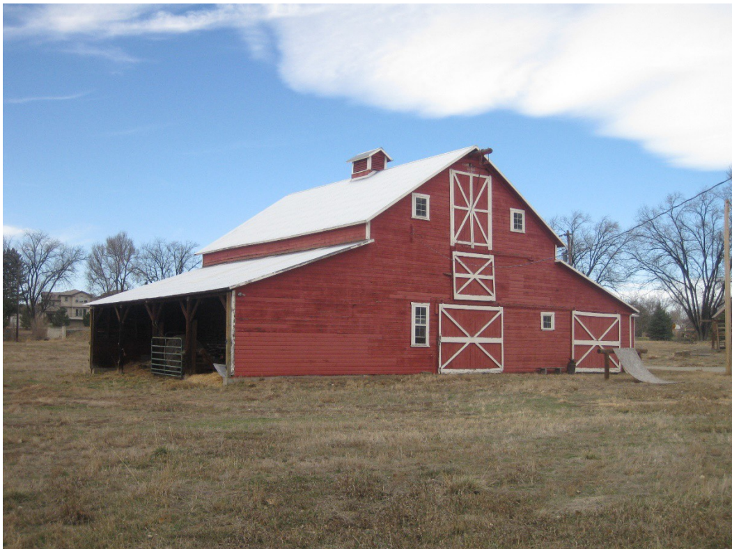
Figure 10. 151 County barn, south and east sides, facing northwest.
