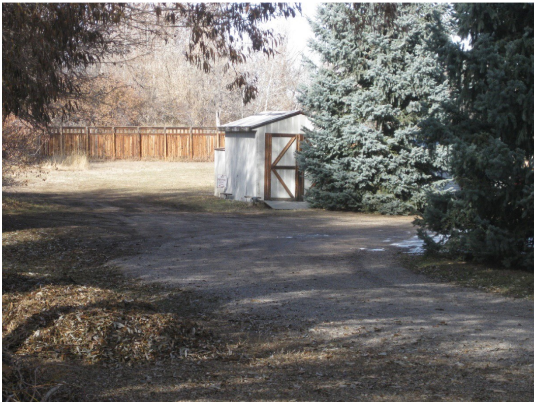
Figure 6. 309 W. Spruce shed 2, west and south sides, facing north-northeast.
