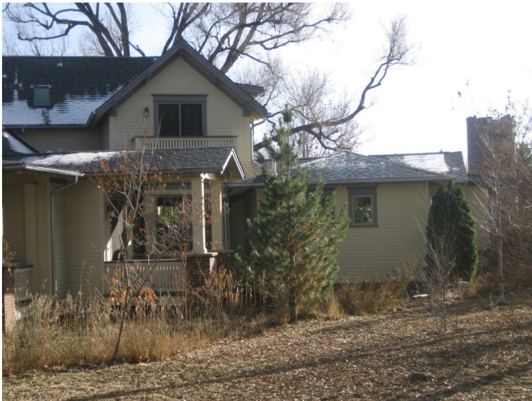
Figure 6. 310 W. Spruce house and silo, north side, facing south.
