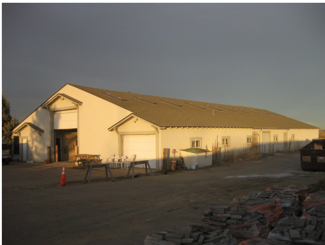
Figure 38. 10433 Dillon dairy barn north of property, west and south sides, facing northeast.
