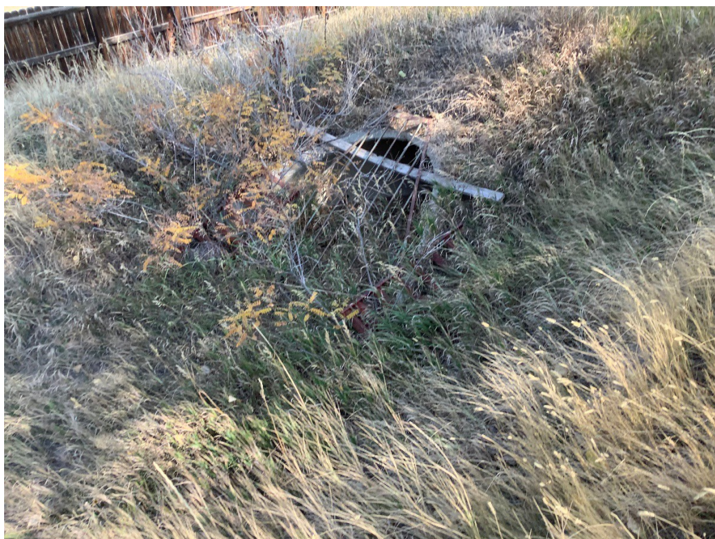
Figure 20. 5BL9577.2 concrete u-culvert, facing northeast, M. Taylor, 10/8/2020.
