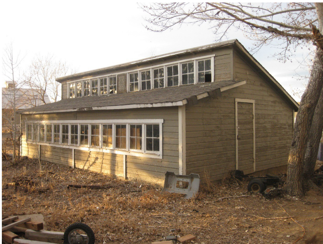
Figure 12. 10433 Dillon coop, south and east sides, facing northwest.
