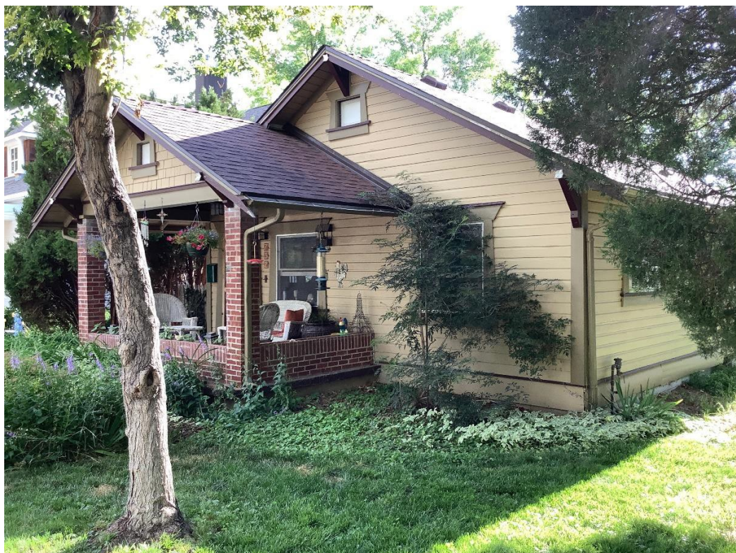
Figure 3. 732 Grant, facing northeast.
