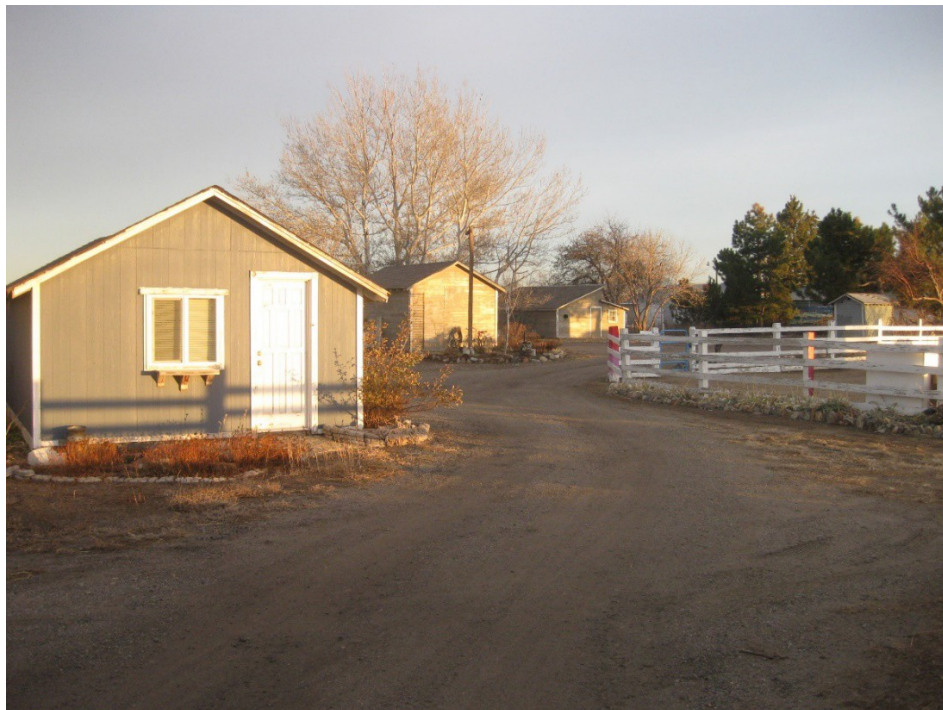
Figure 37. 10433 Dillon heifer barn/office, granary 1, coop, and small outbuilding, north and west sides, facing southeast.
