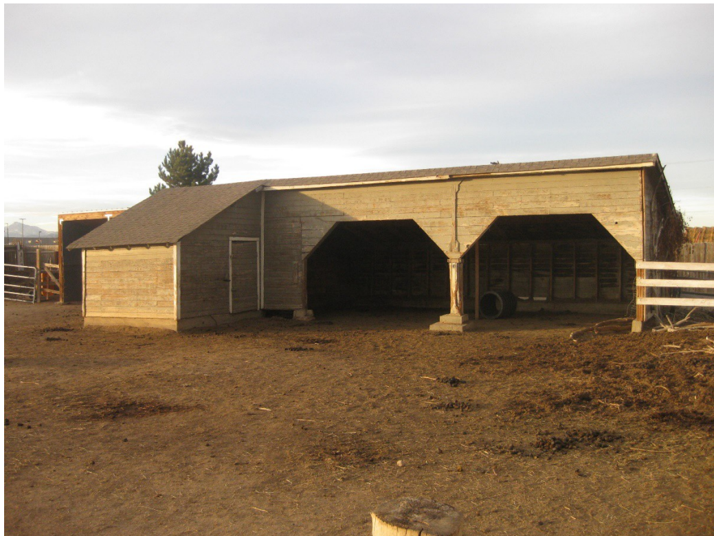
Figure 33. 10433 Dillon stable 2, south and east sides, facing northwest.
