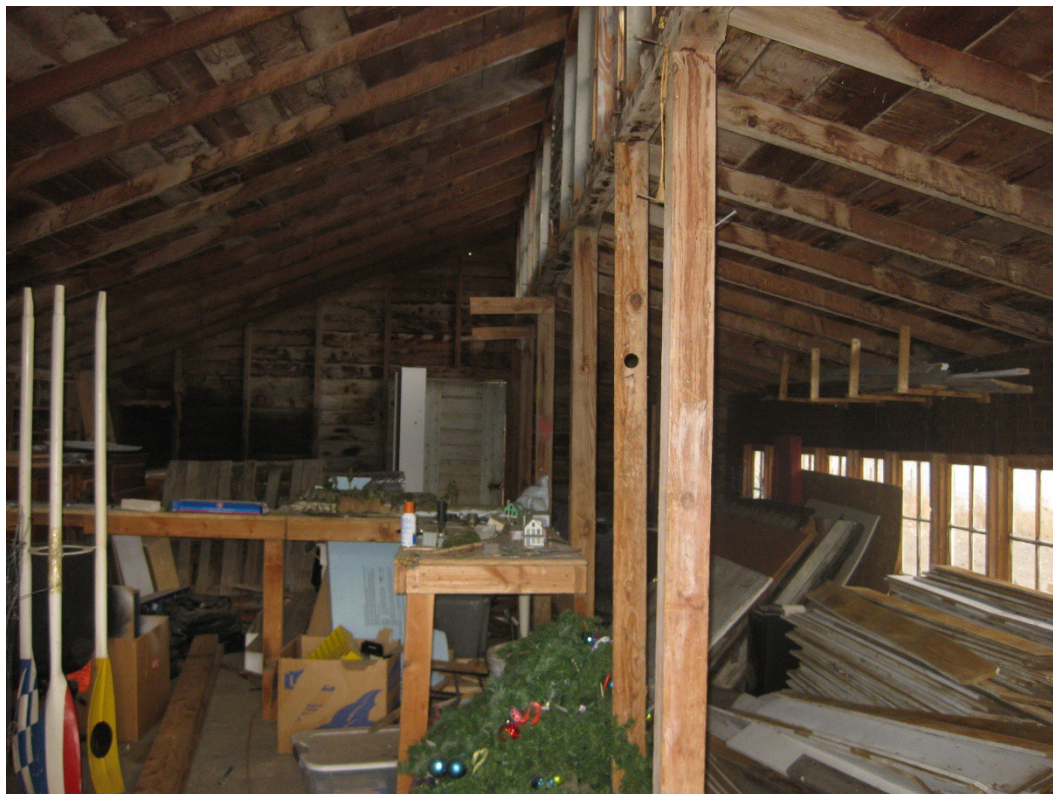
Figure 14. 10433 Dillon coop interior, facing east.
