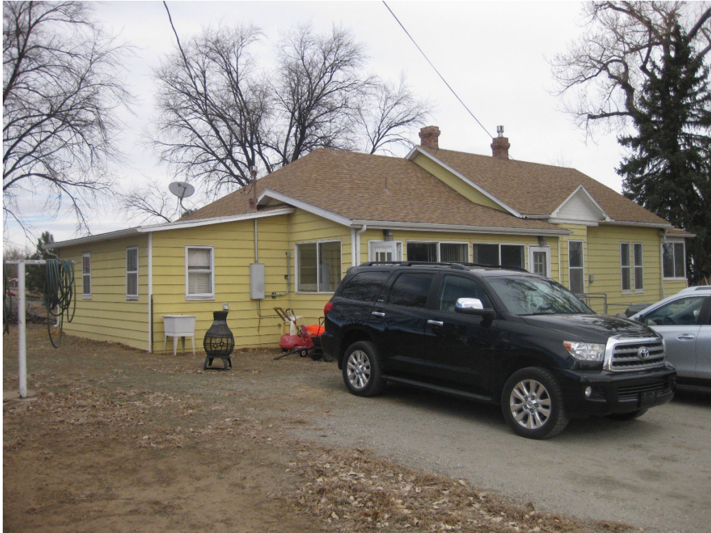
Figure 5. 151 County house, west and south sides, facing northeast.
