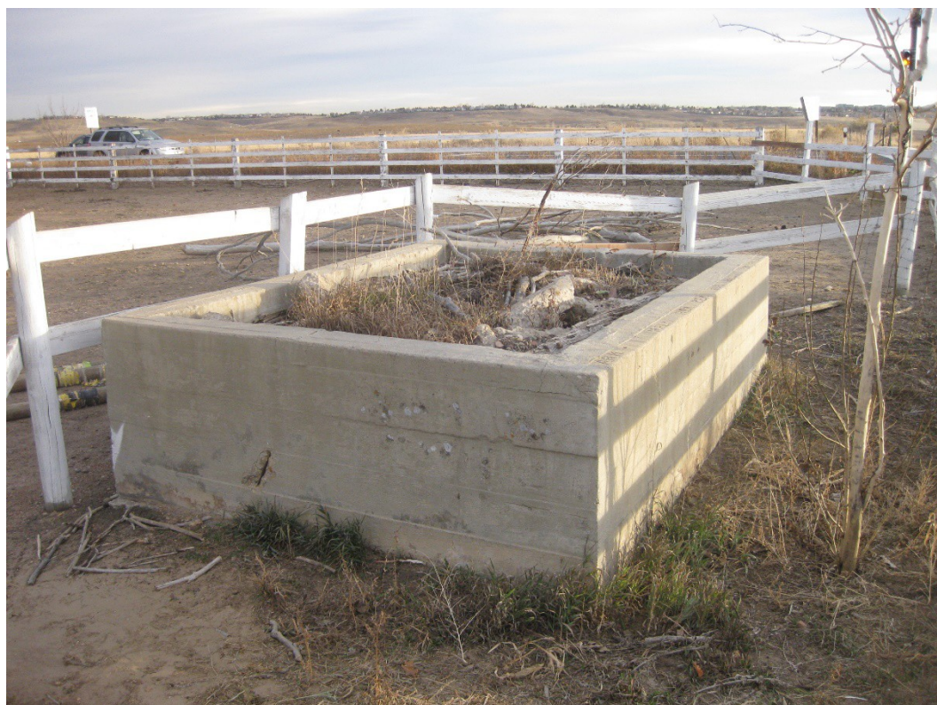
Figure 28. 10433 Dillon trough 1, north and west sides, facing southeast.
