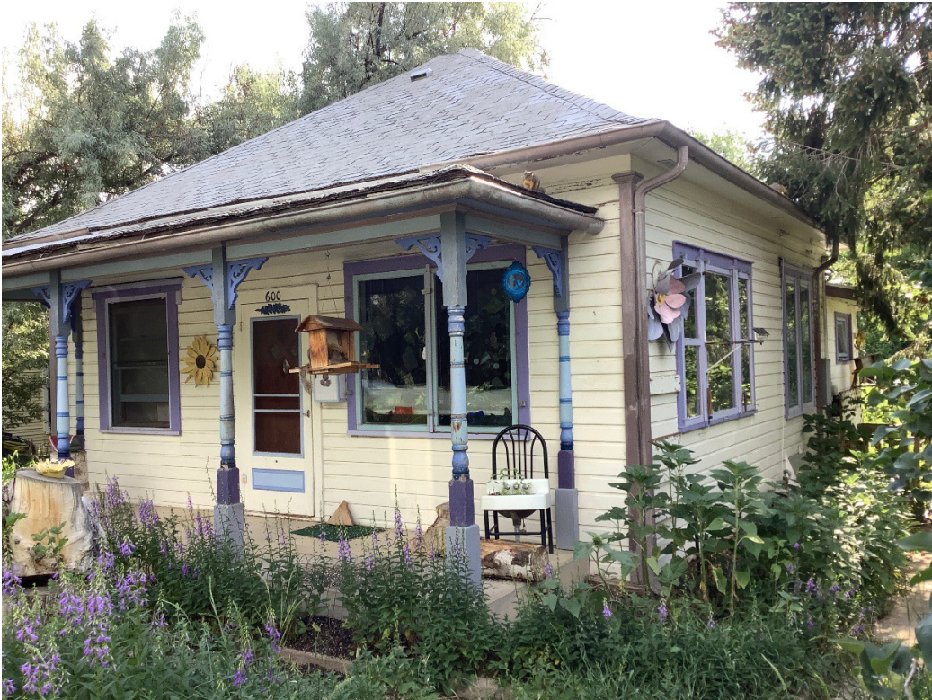
Figure 3. 600 Grant, facing northeast.
