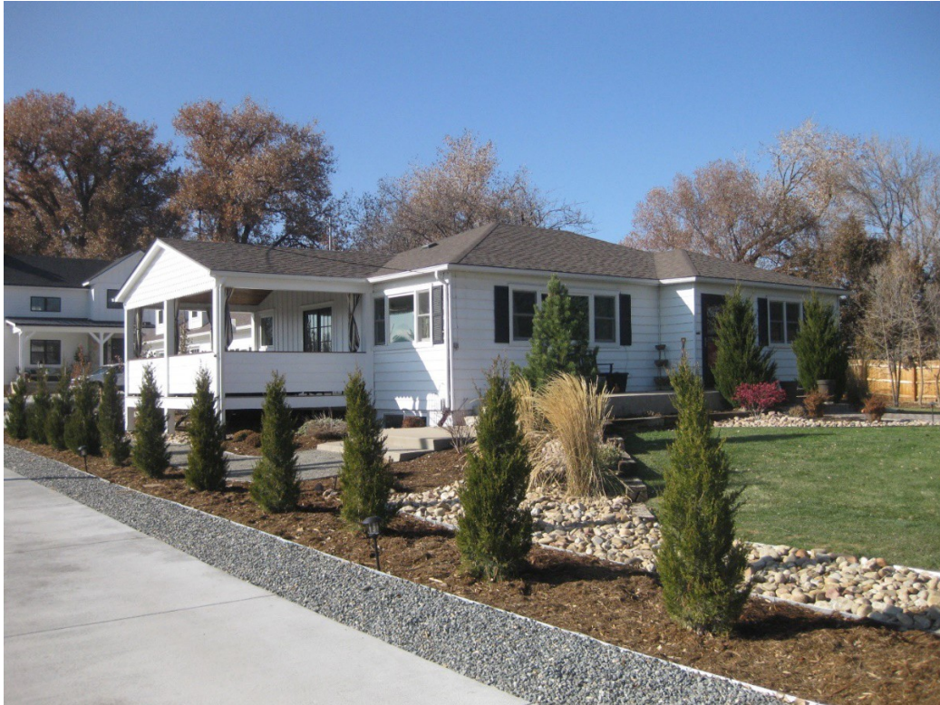
Figure 3. 1515 Main house, south and east sides, facing northwest.
