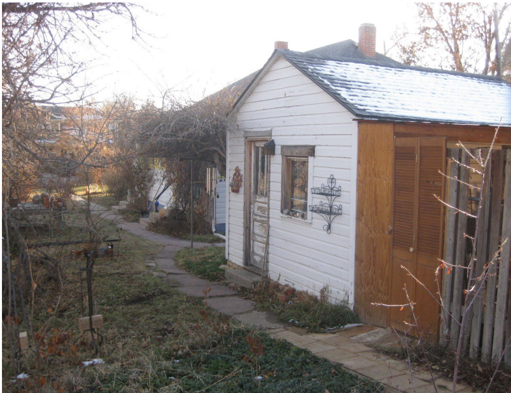
Figure 30. 109 W. Spruce house and shed 3, east sides, facing southwest.
