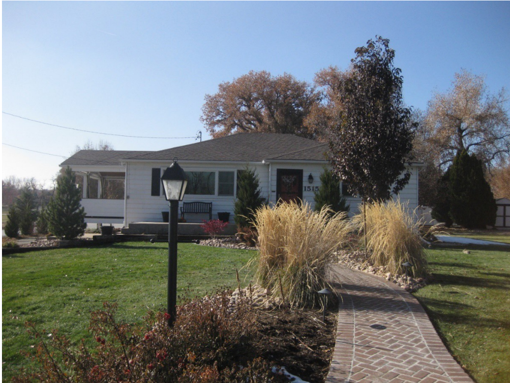
Figure 5. 1515 Main house, east side, facing west.
