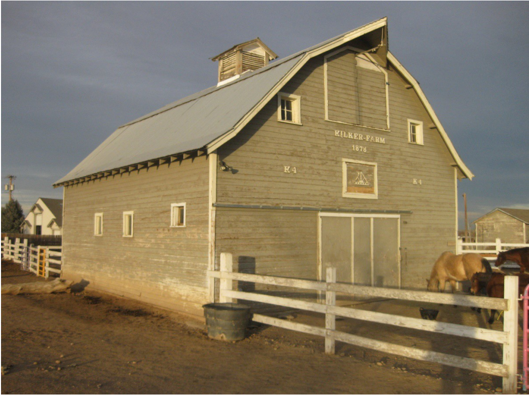
Figure 7. 10433 Dillon barn, west and south sides, facing northeast.
