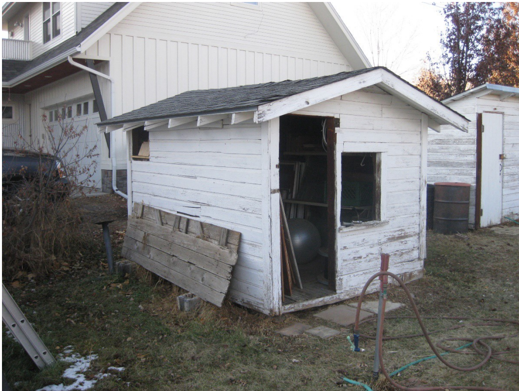
Figure 12. 109 W. Spruce shed 1, south and east sides, facing northwest.
