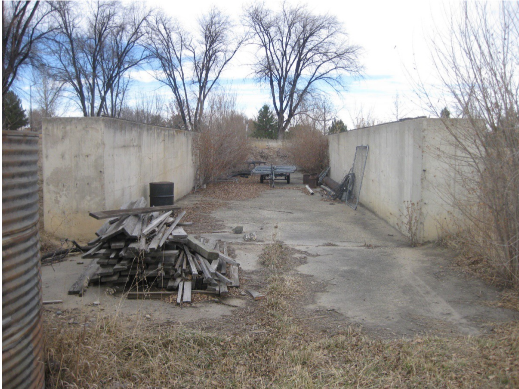
Figure 21. 151 County concrete foundation, south side, facing north.
