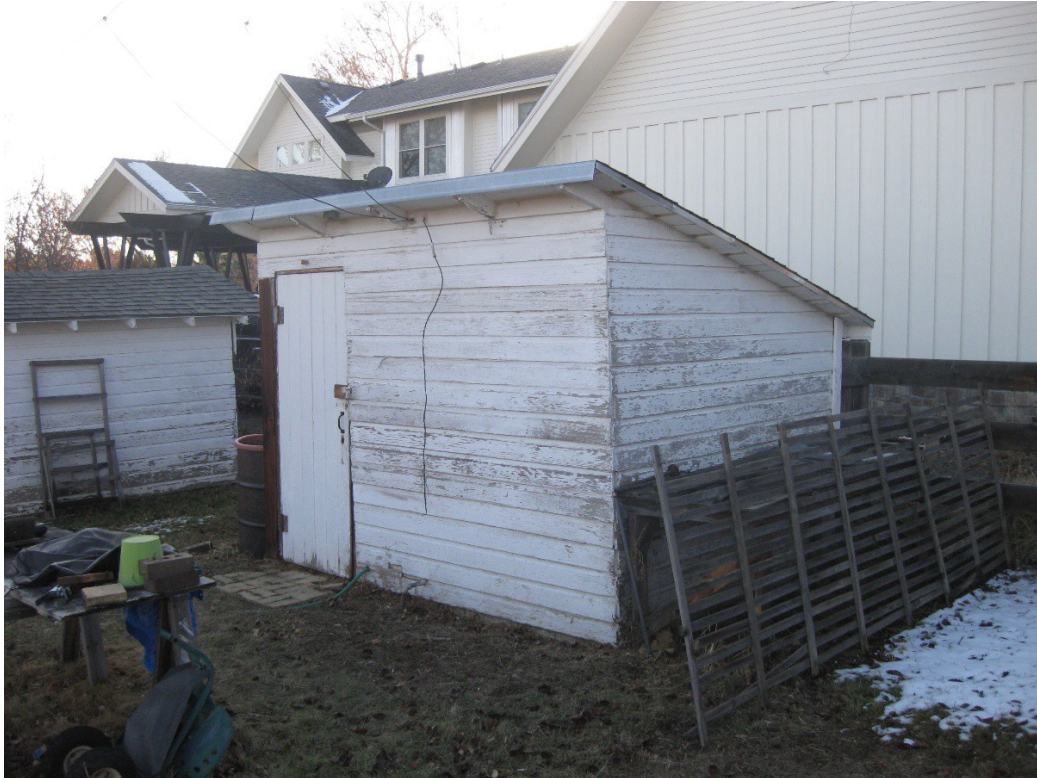
Figure 15. 109 W. Spruce shed 2, east and north sides, facing southwest.
