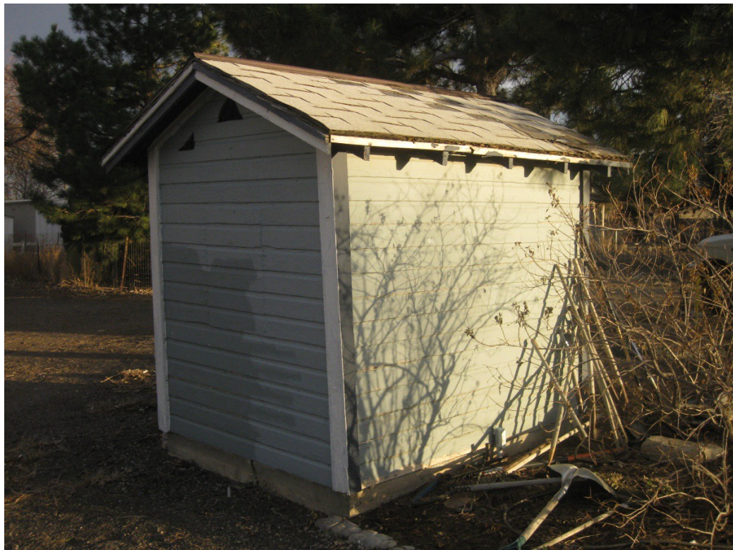
Figure 19. 10433 Dillon small outbuilding, north and west sides, facing southeast.
