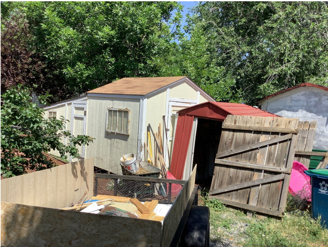
Figure 6. 600 Grant, sheds, facing northwest.
