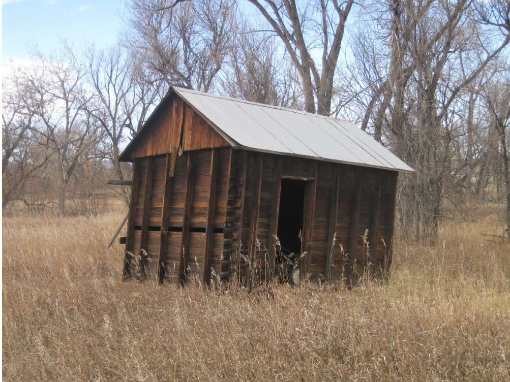
Figure 25. 151 County tack shed, south and east sides, facing northwest.
