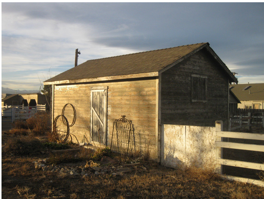
Figure 22. 10433 Dillon granary 1, south and east sides, facing northwest.
