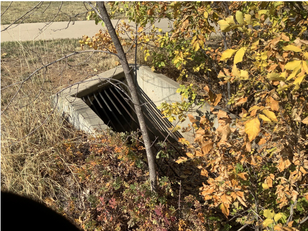
Figure 12. 5BL9577.2 concrete culvert with metal grate, facing west, M. Taylor, 10/8/2020.
