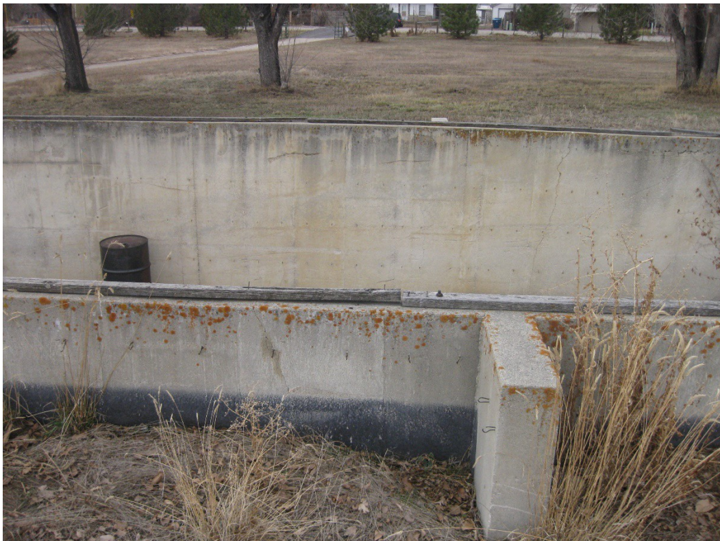
Figure 22. 151 County concrete foundation, east side, facing west.
