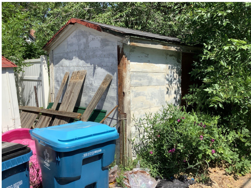
Figure 5. 612 Grant, shed, facing northwest.
