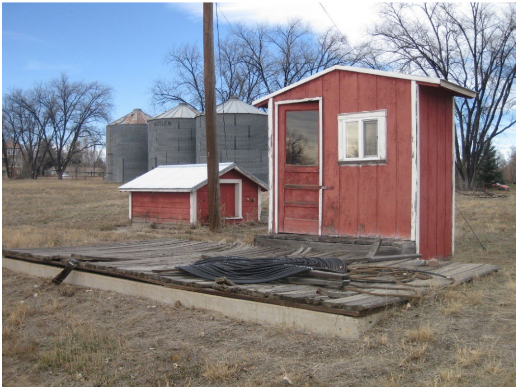
Figure 16. 151 County grain bins 1–3, pump house, and weigh house, south and east sides, facing northwest
