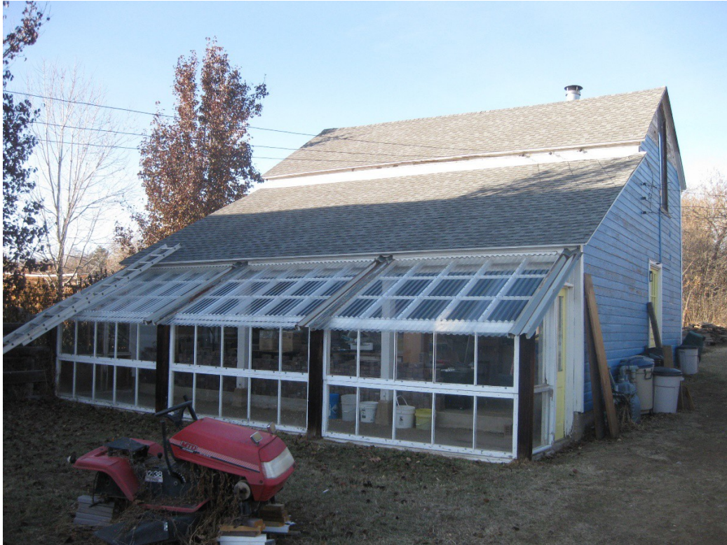
Figure 17. 109 W. Spruce barn, south and east sides, facing northwest.
