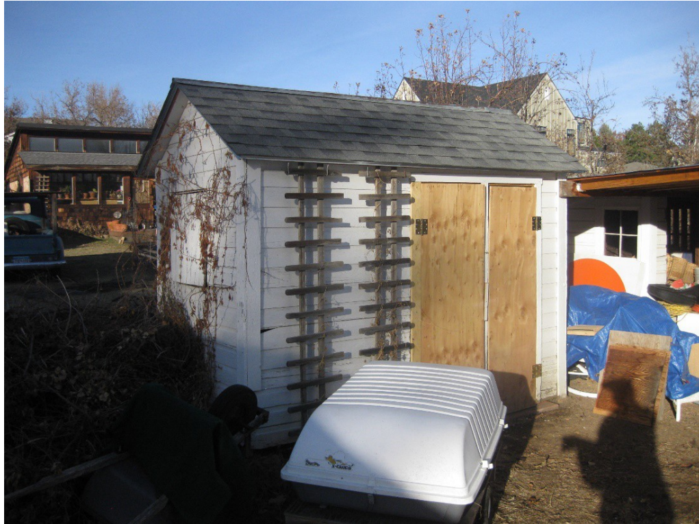
Figure 27. 109 W. Spruce outhouse / coal shed, west and south sides, facing northeast.
