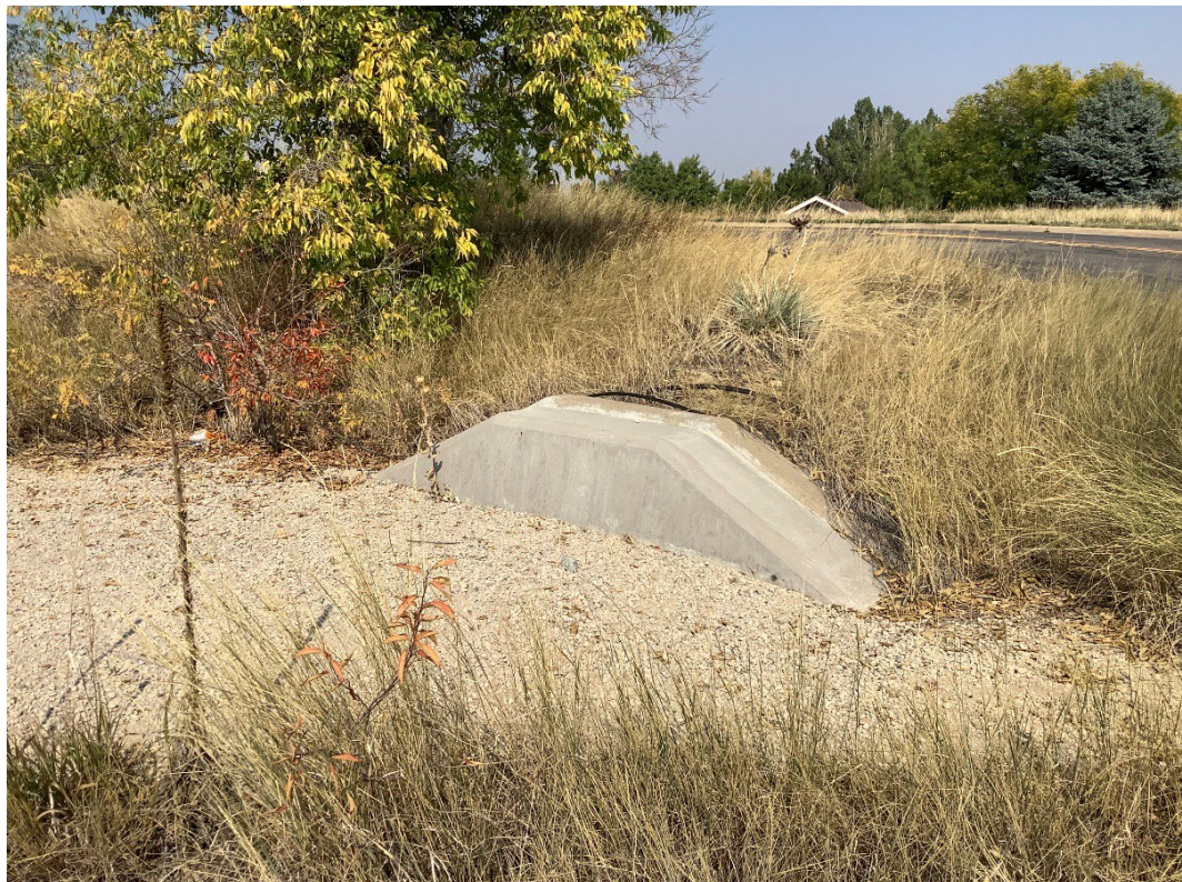
Figure 21. 5BL9577.2 concrete culvert, gravel filled, facing north, M. Taylor, 10/8/2020.
