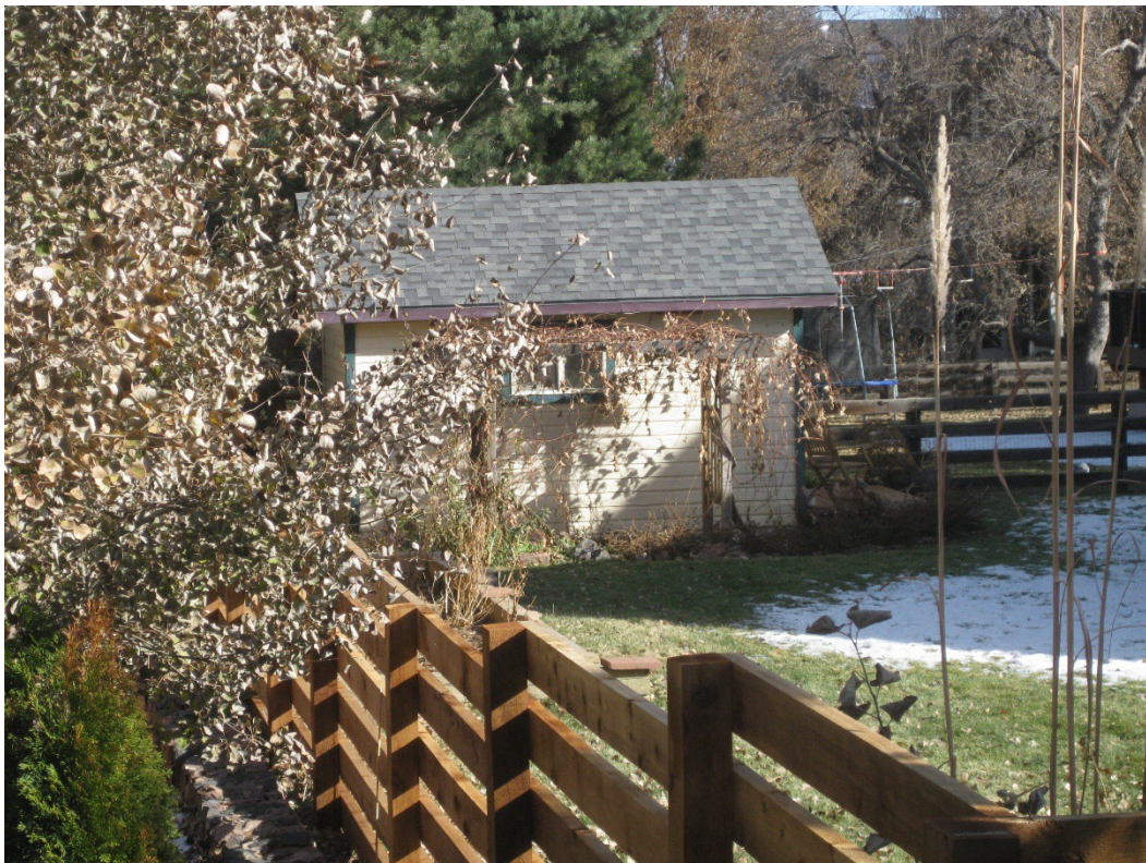
Figure 6. 501 W. Spruce shed, west side, facing east-southeast.
