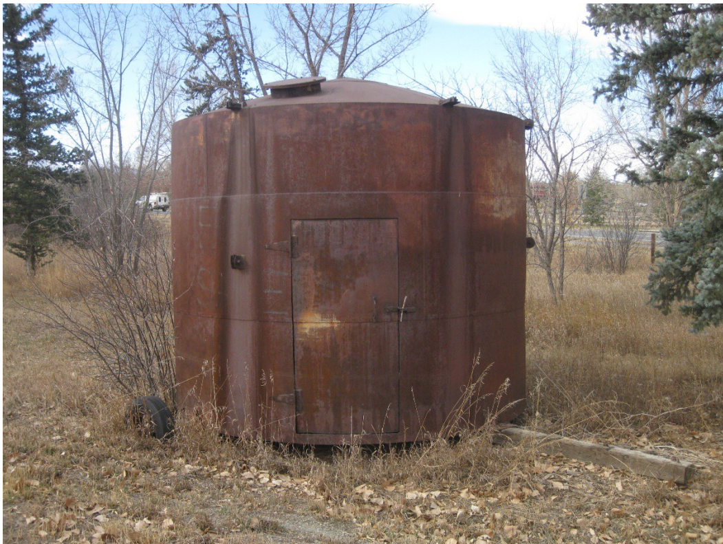
Figure 28. 151 County tank, south and east sides, facing northwest.
