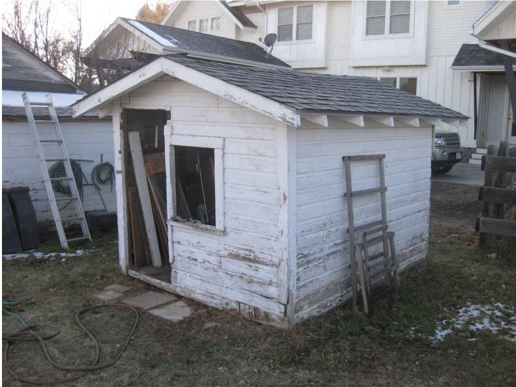
Figure 13. 109 W. Spruce shed 1, east and north sides, facing southwest.
