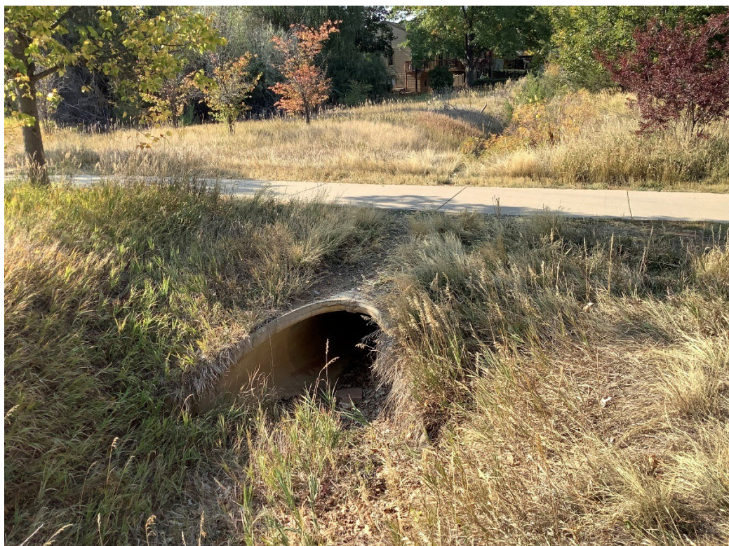
Figure 4. 5BL9577.2 concrete u-culvert, facing south, M. Taylor, 10/8/2020.
