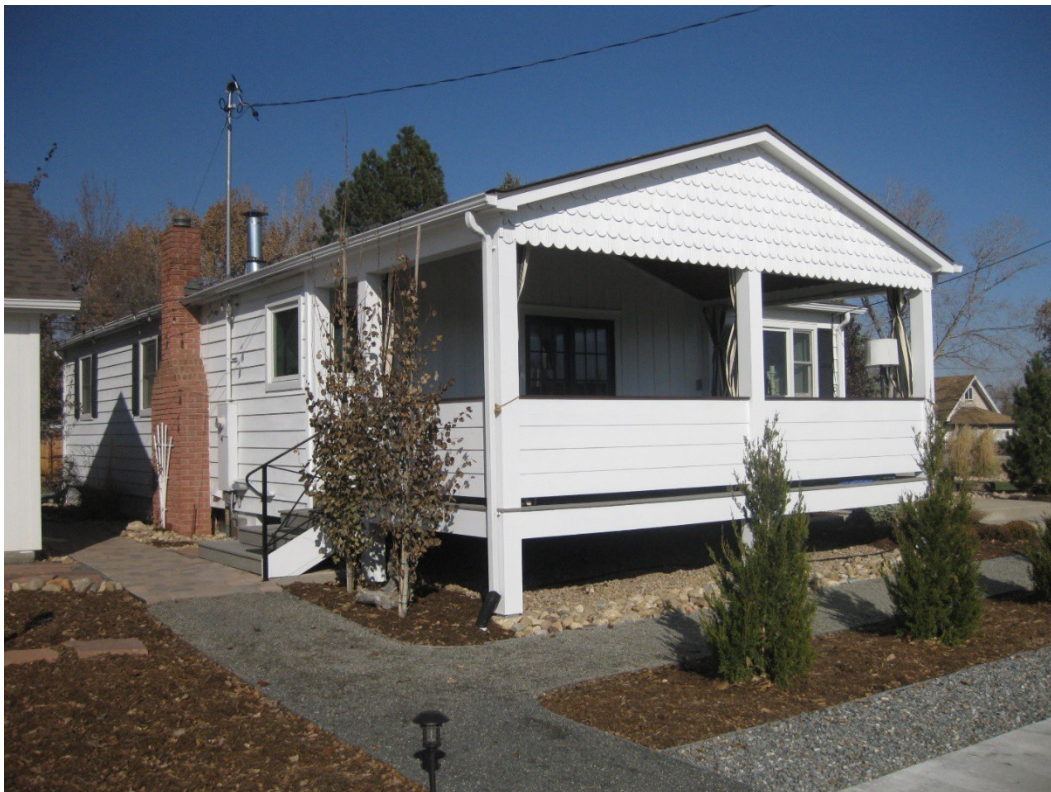
Figure 4. 1515 Main house, west and south sides, facing northeast.
