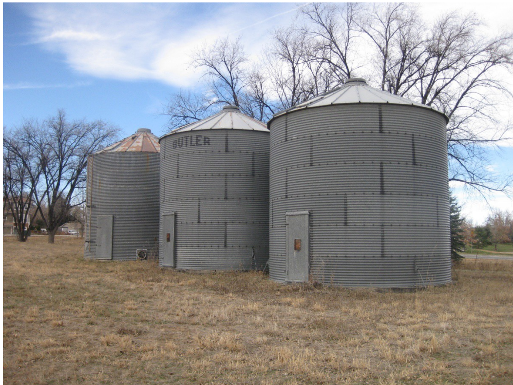
Figure 18. 151 County grain bins 1–3, south and east sides, facing northwest.
