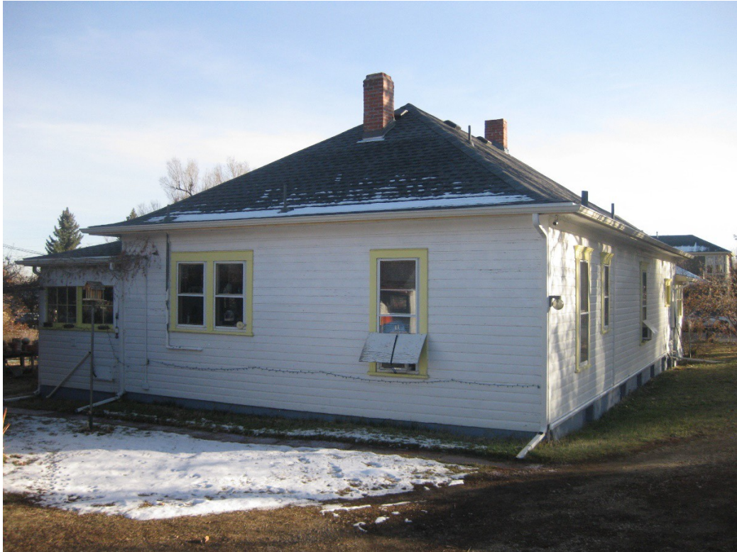
Figure 5. 109 W. Spruce house, north and west sides, facing south-southeast.
