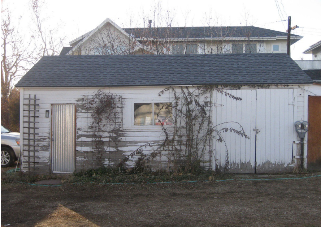
Figure 9. 109 W. Spruce garage, east side, facing west.
