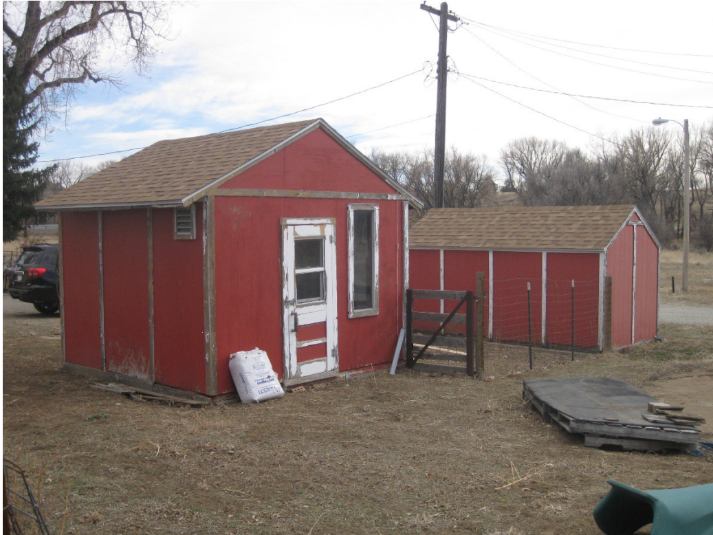
Figure 15. 151 County shed 2 and shed 1, north and west sides, facing southeast.
