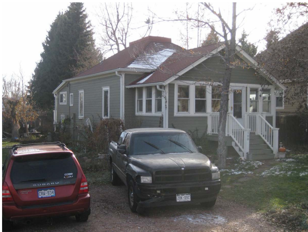
Figure 5. 100 W Spruce Street house, east and north sides, facing southwest.
