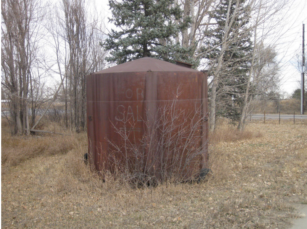
Figure 27. 151 County tank, south and west sides, facing northeast.
