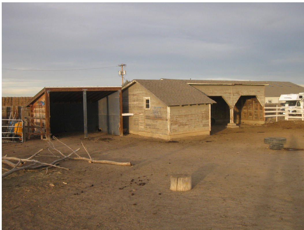
Figure 32. 10433 Dillon stable 1 and stable 2, west and south sides, facing northeast.
