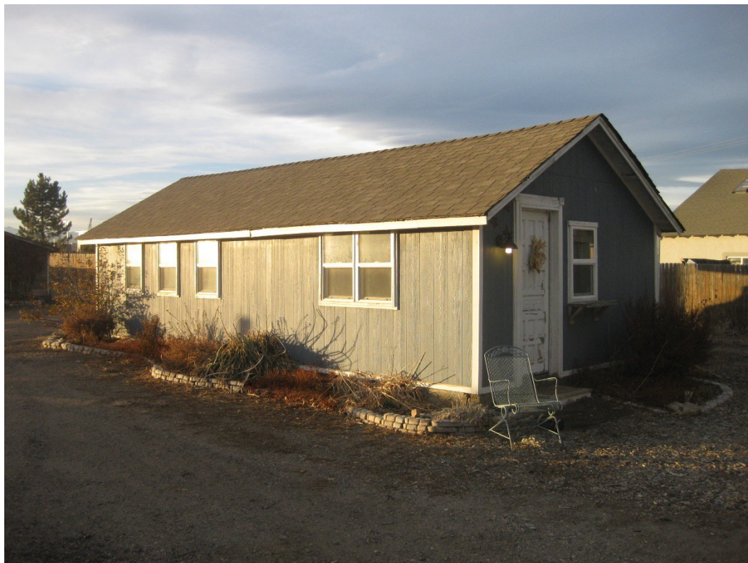
Figure 36. 10433 Dillon heifer barn/office, south and east sides, facing northwest.
