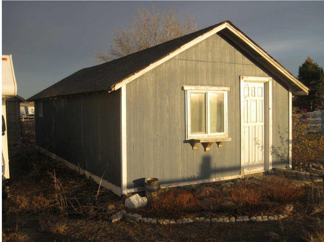
Figure 35. 10433 Dillon heifer barn/office, north and west sides, facing southeast.
