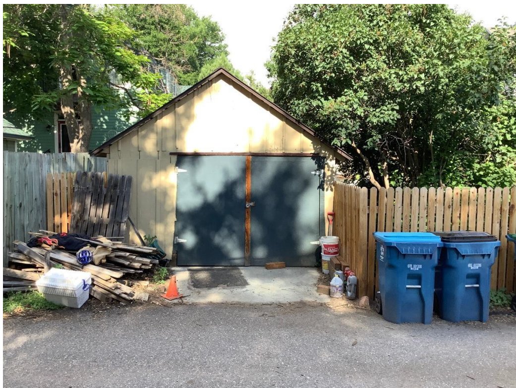
Figure 5. 732 Grant, garage, facing west.
