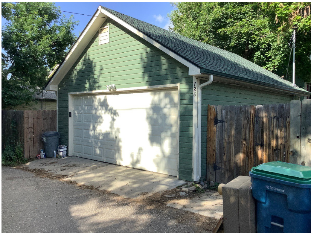
Figure 5. 728 Grant, garage, facing southwest.
