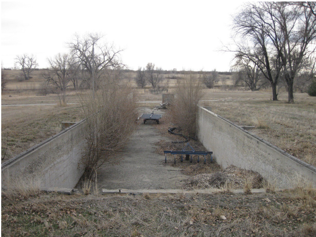
Figure 20. 151 County concrete foundation, north side, facing south.
