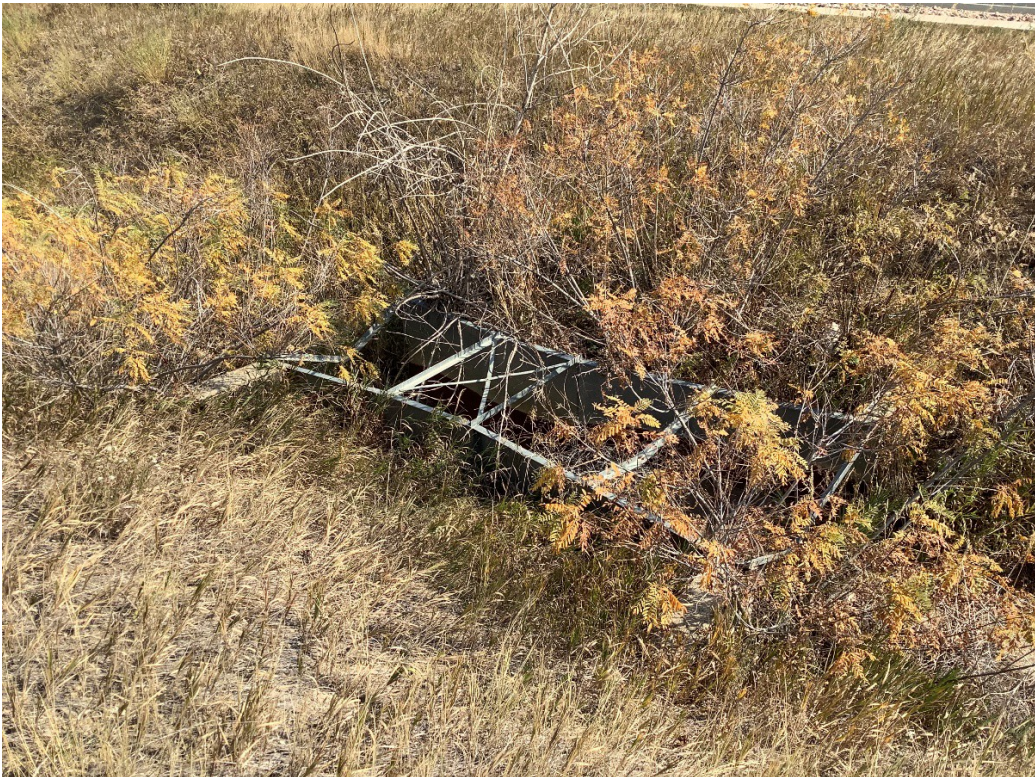
Figure 16. 5BL9577.2 feature 3, facing west, M. Taylor, 10/8/2020.
