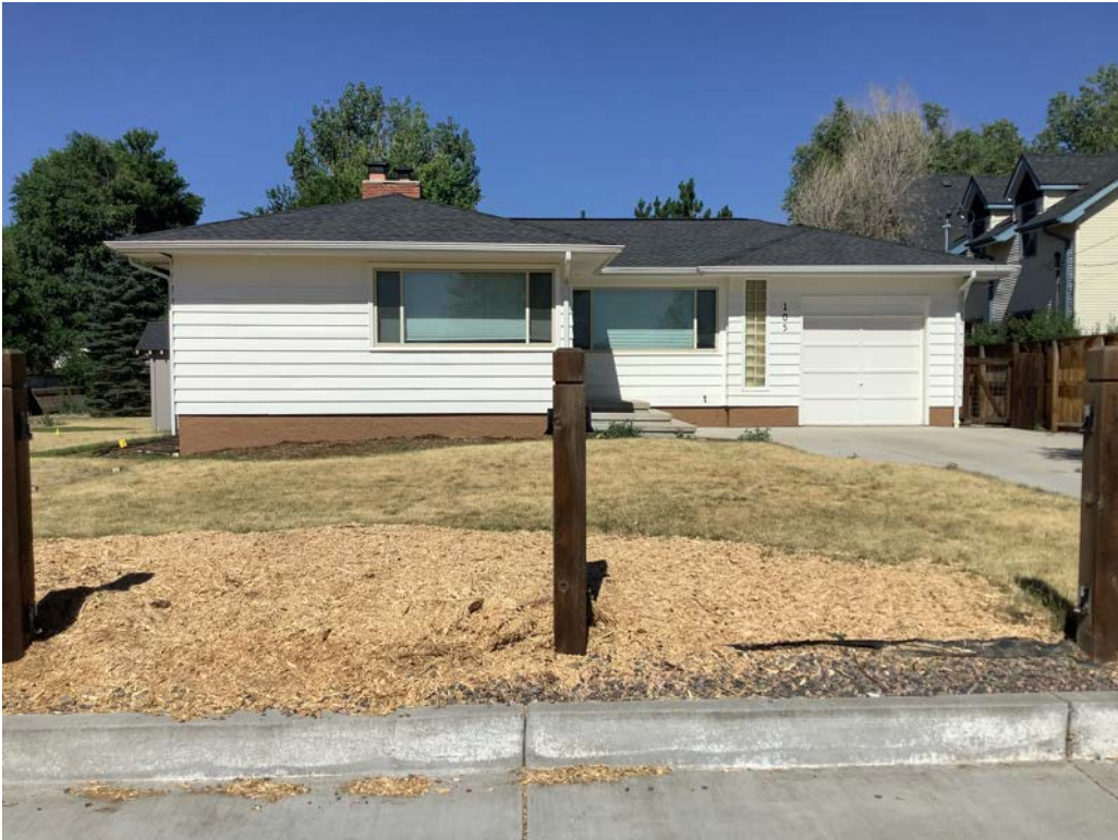
Figure 3. 105 Roosevelt, facing west.
