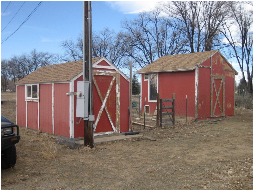
Figure 14. 151 County shed 1 and shed 2, south and east sides, facing northwest.
