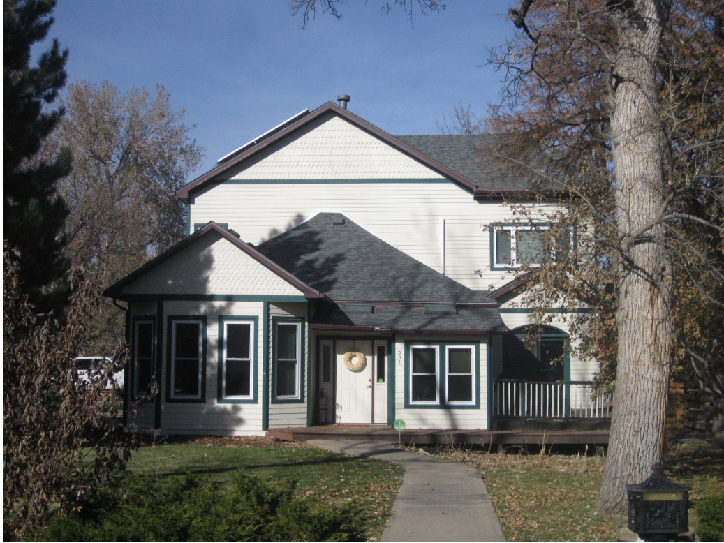
Figure 3. 501 W. Spruce house, south side, facing north.
