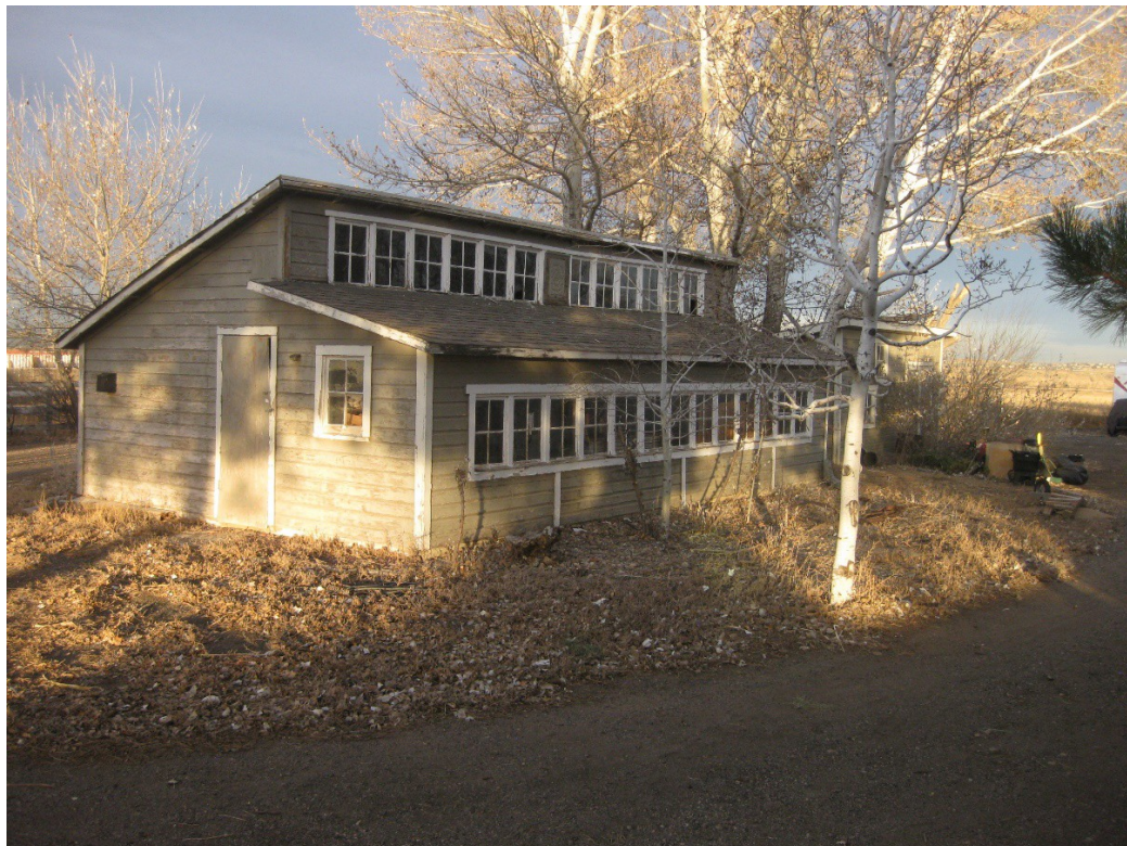
Figure 11. 10433 Dillon coop, west and south sides, facing northeast.
