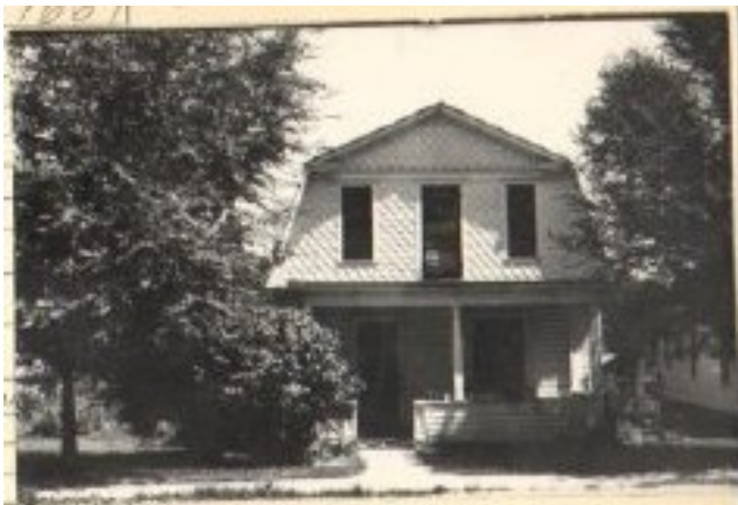
Figure 7. 728 Grant_A1 photo from 1948 Assessor Card, west side, facing east.
