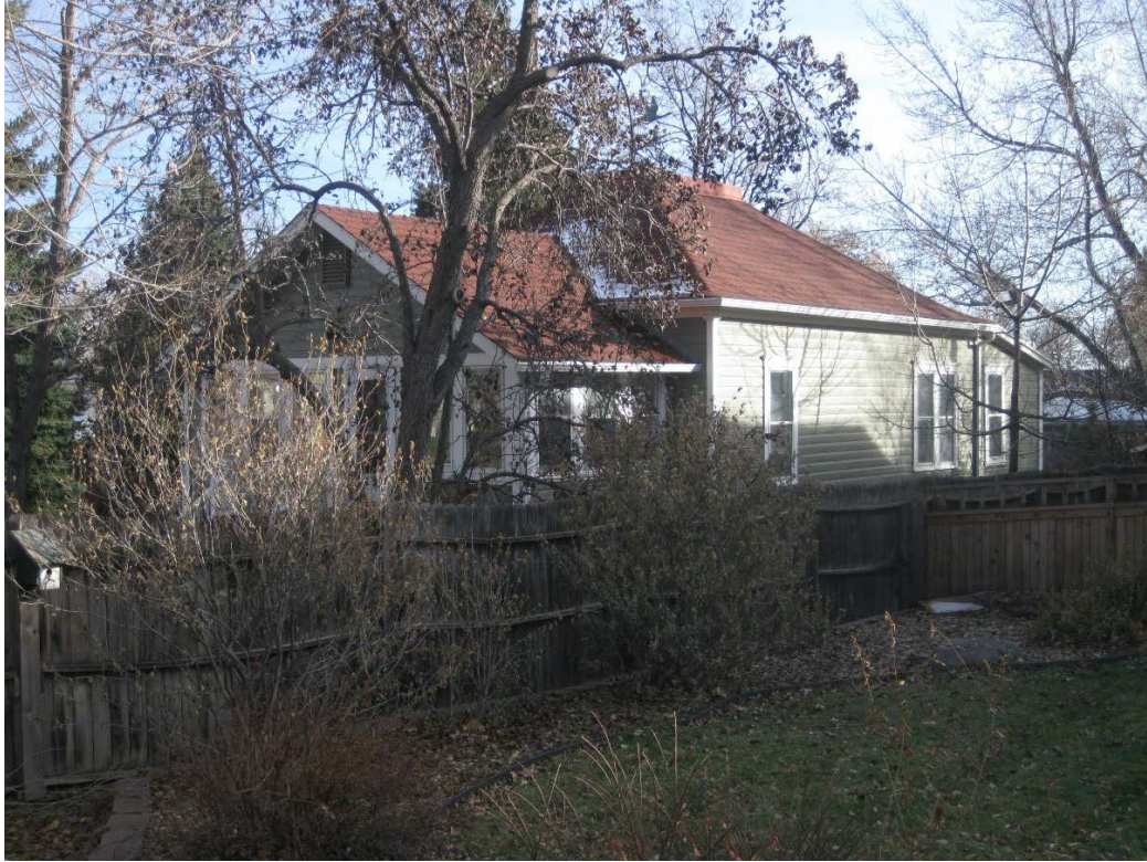
Figure 3. 100 W Spruce Street house, north and west sides, facing southeast.
