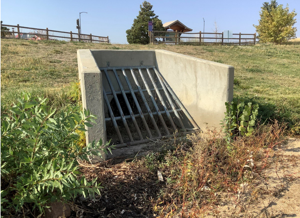
Figure 13. 5BL9577.2 concrete culvert with metal grate, exit point from Harper Lake, facing southwest, M. Taylor, 10/8/2020.
