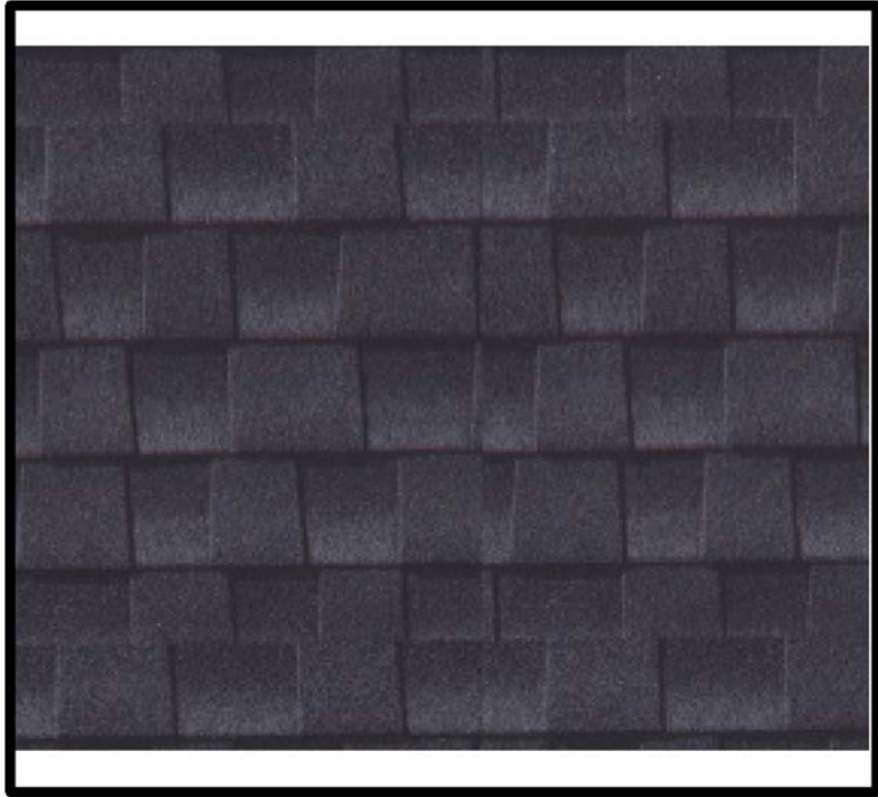
ASPHALT SHINGLE ROOF
