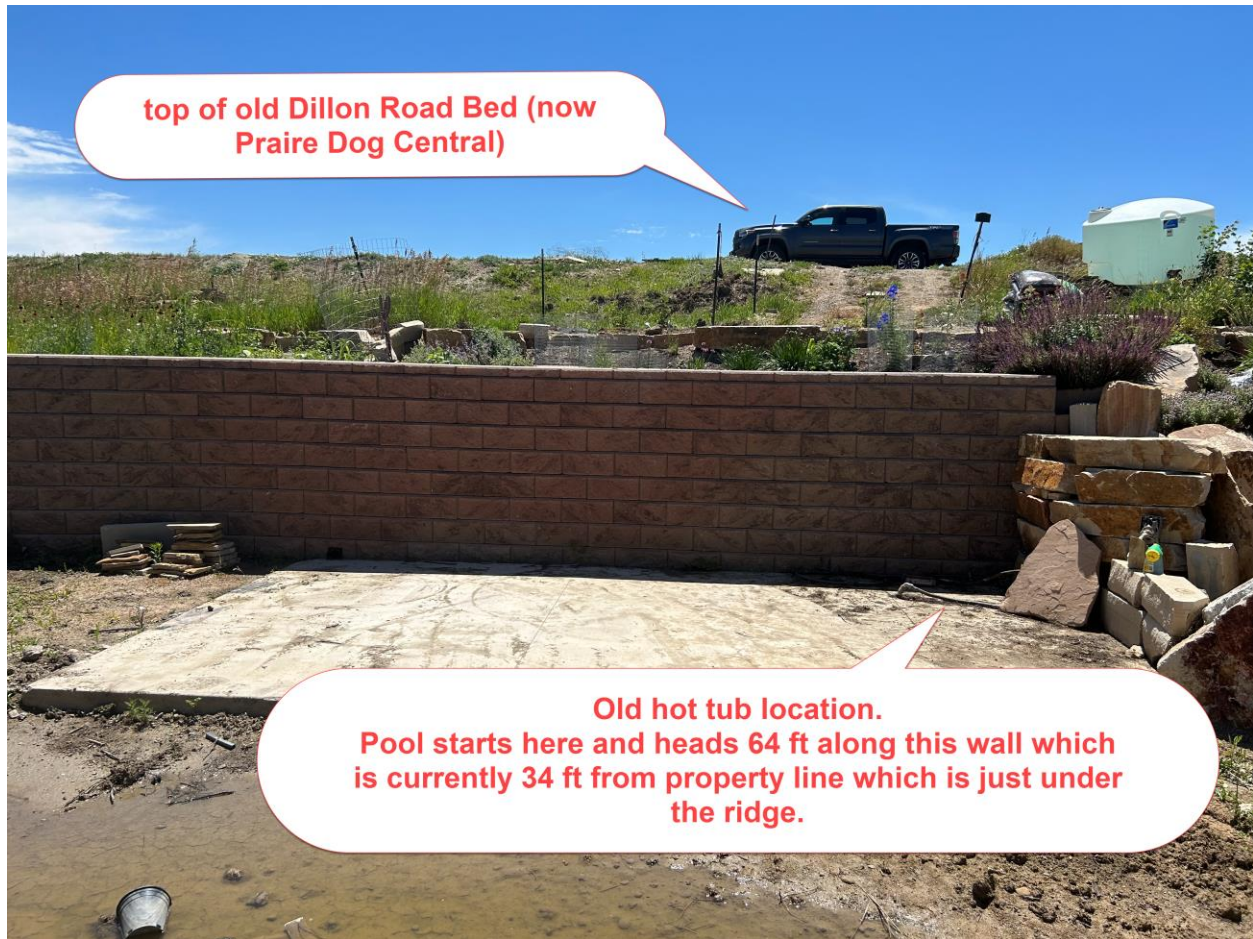
Figure 2 - Existing Retaining wall where hot tub used to be located.
