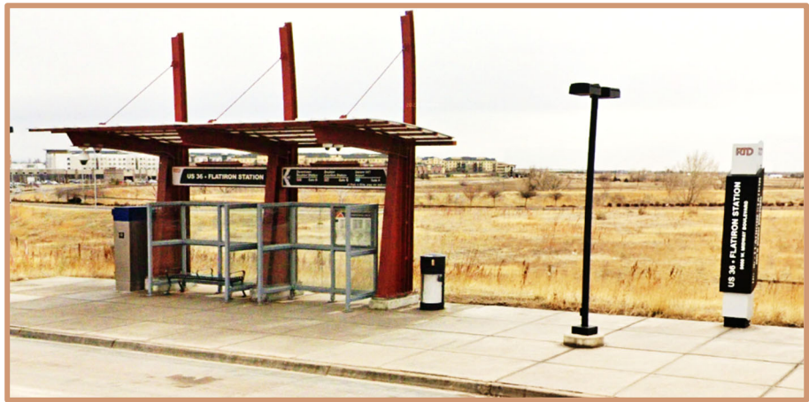
Photo 1: US 36 and East Flatiron Station
