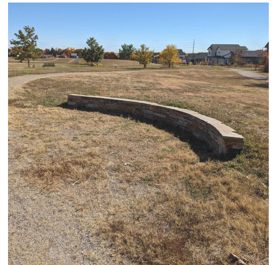
Existing Stone Wall
