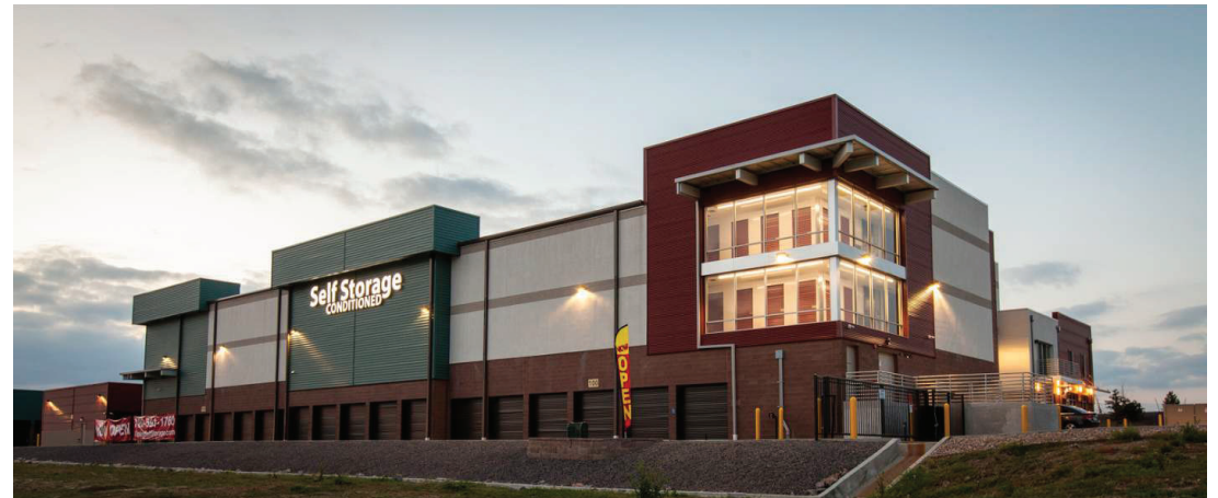
SAMPLE STORAGE FACILITIES
