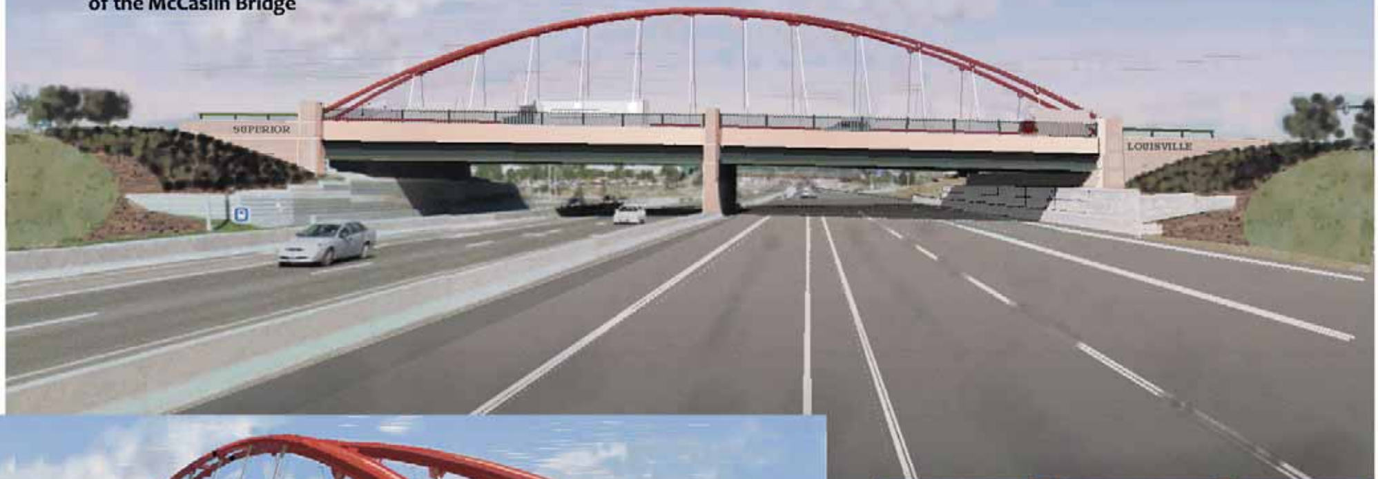
US 36 Northbound View of the McCaslin Bridge
