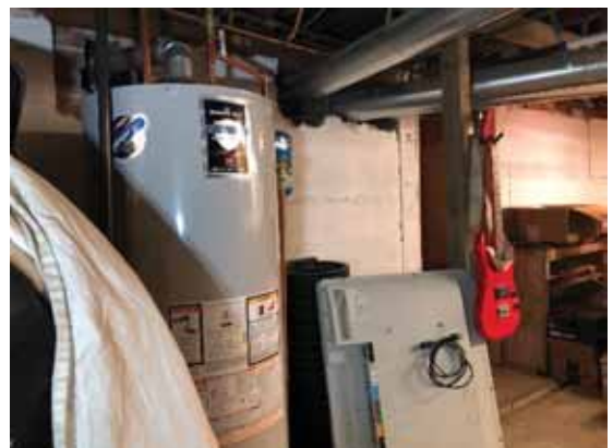
Central foundation wall with openings for ductwork.
