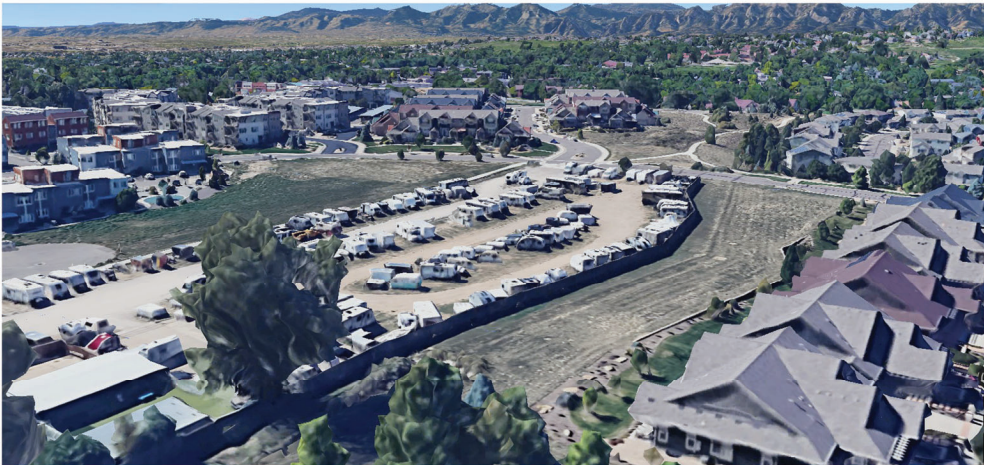
VIEW FROM THE NORTHEAST
