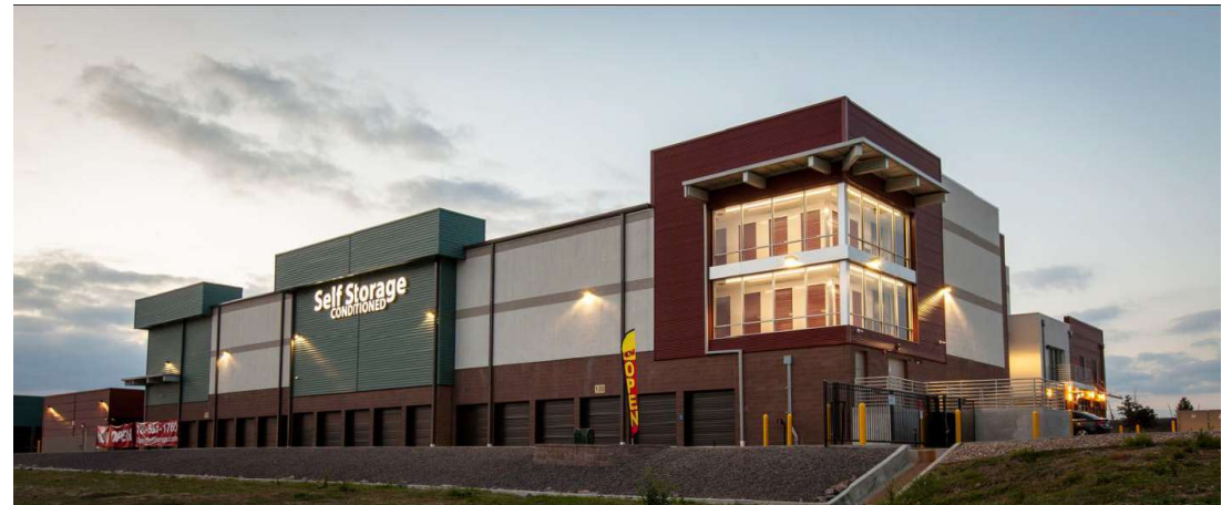
SAMPLE STORAGE FACILITIES
