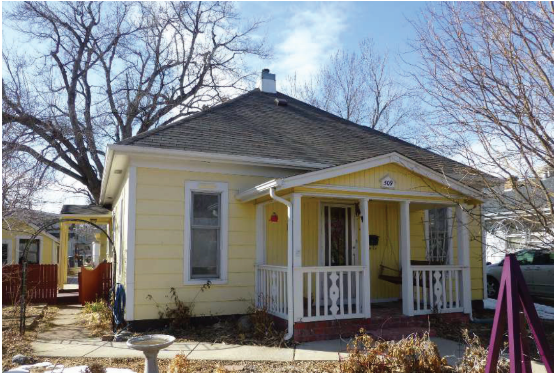
Fiber board siding and T-111 siding
