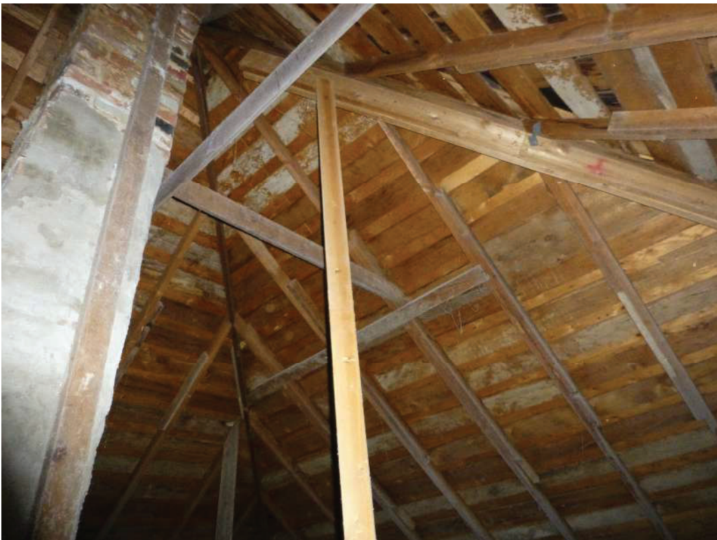
Reinforce roof rafters
