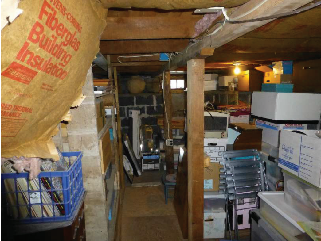
Replace beams supporting first floor structure
