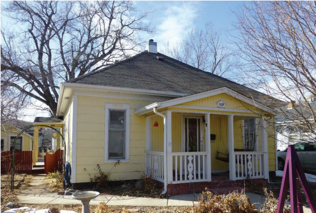
Fiber board siding and T-111 siding
