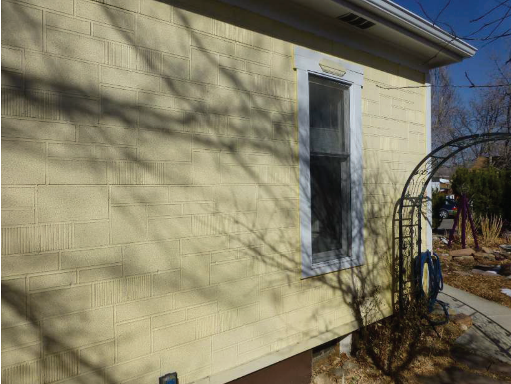
Asphalt siding (painted)
