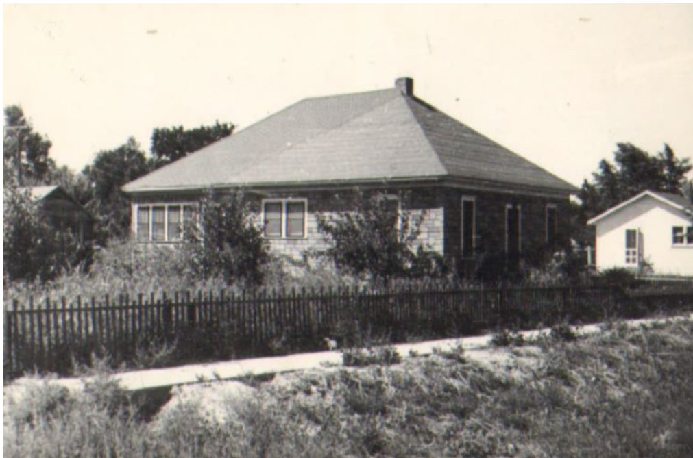
Photo of 509 LaFarge Avenue from the 1948 Assessor's Card.
