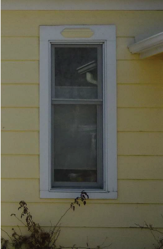
Aluminum-clad replacement windows
