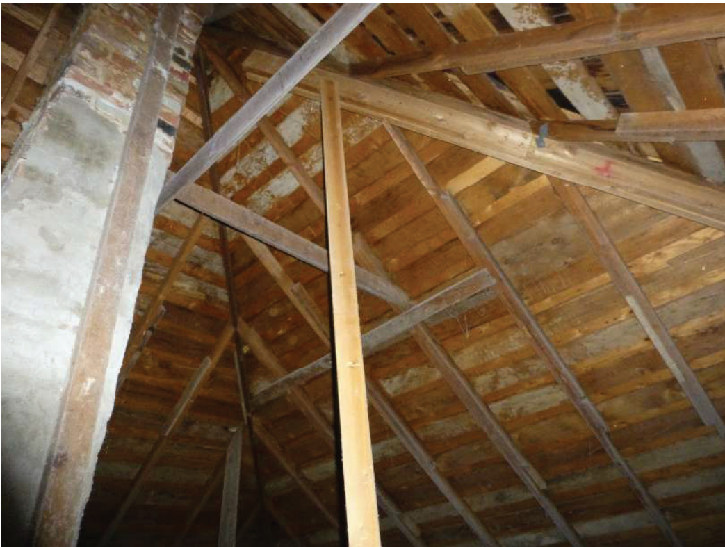
Reinforce roof rafters
