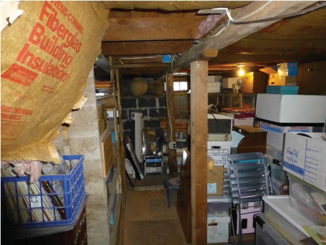
Replace beams supporting first floor structure
