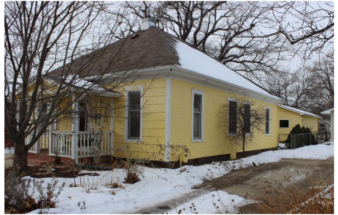
View from northeast corner
