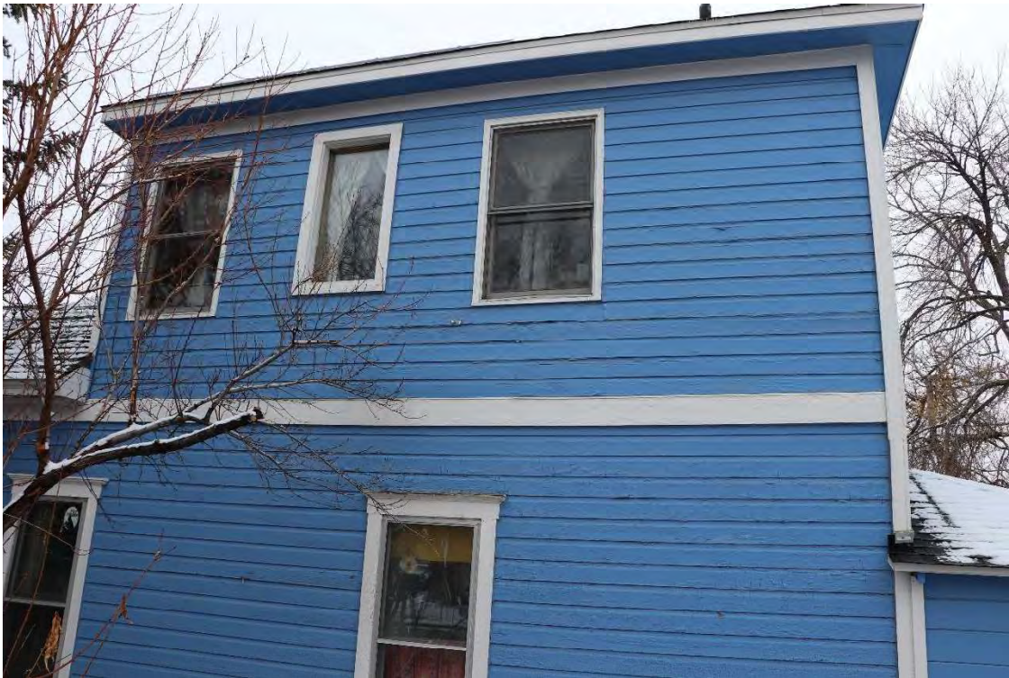
Image 11: Grant Street elevation. The white belt course separates the upper addition from the original first floor. Note the similar but distinct wood siding and window casing on each section
