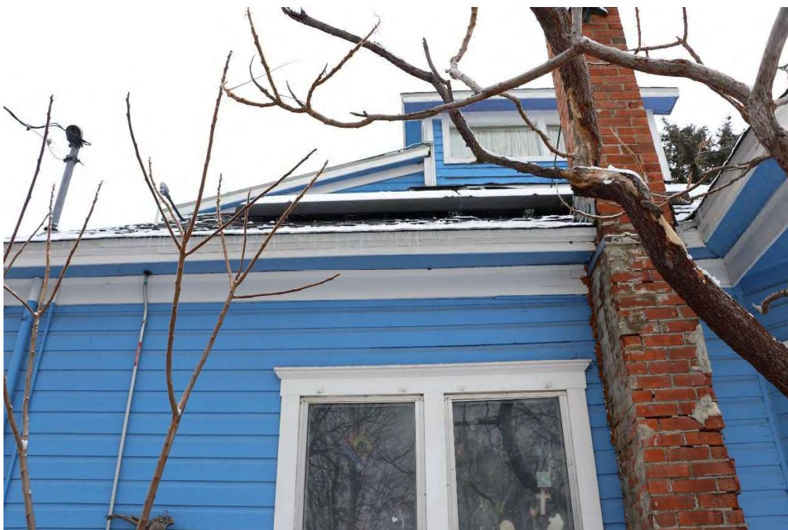
Image 42: Electrical Service and Panels. Service connection visible on left above roofline. Solar panels are flat to the roof to the left of the chimney
