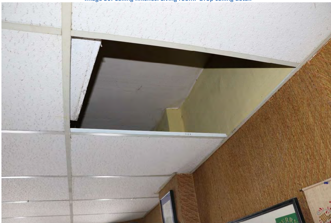
Image 31: Ceiling finishes. Living room. Drop ceiling detail
