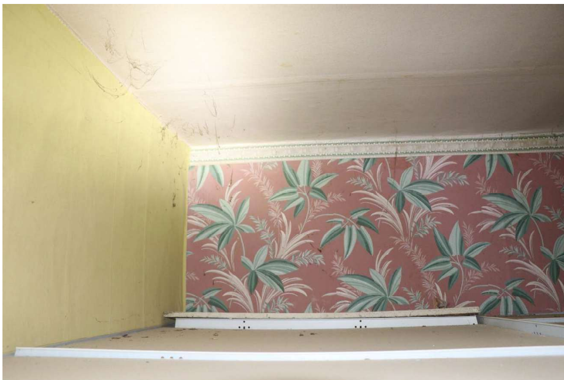
Image 32: Ceiling finishes. Living room. Wallpaper over drop ceiling
