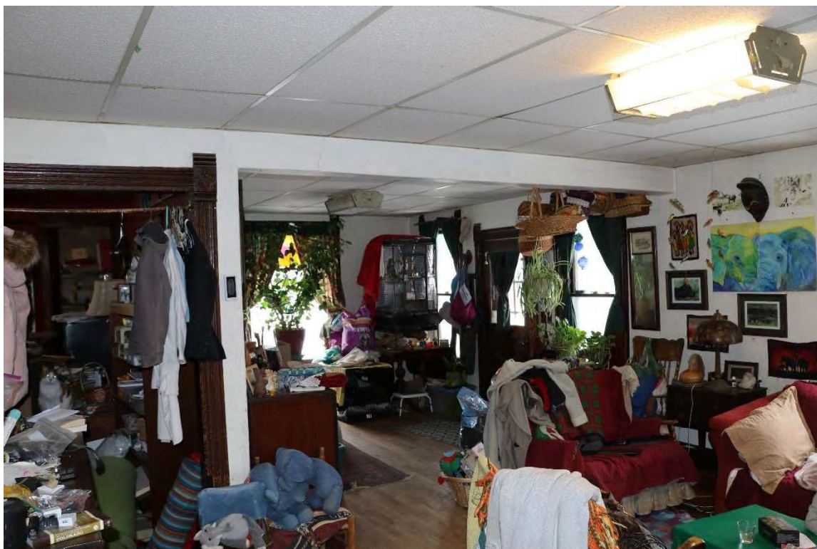
Image 30: Ceiling finishes. Living room. Drop ceiling detail
