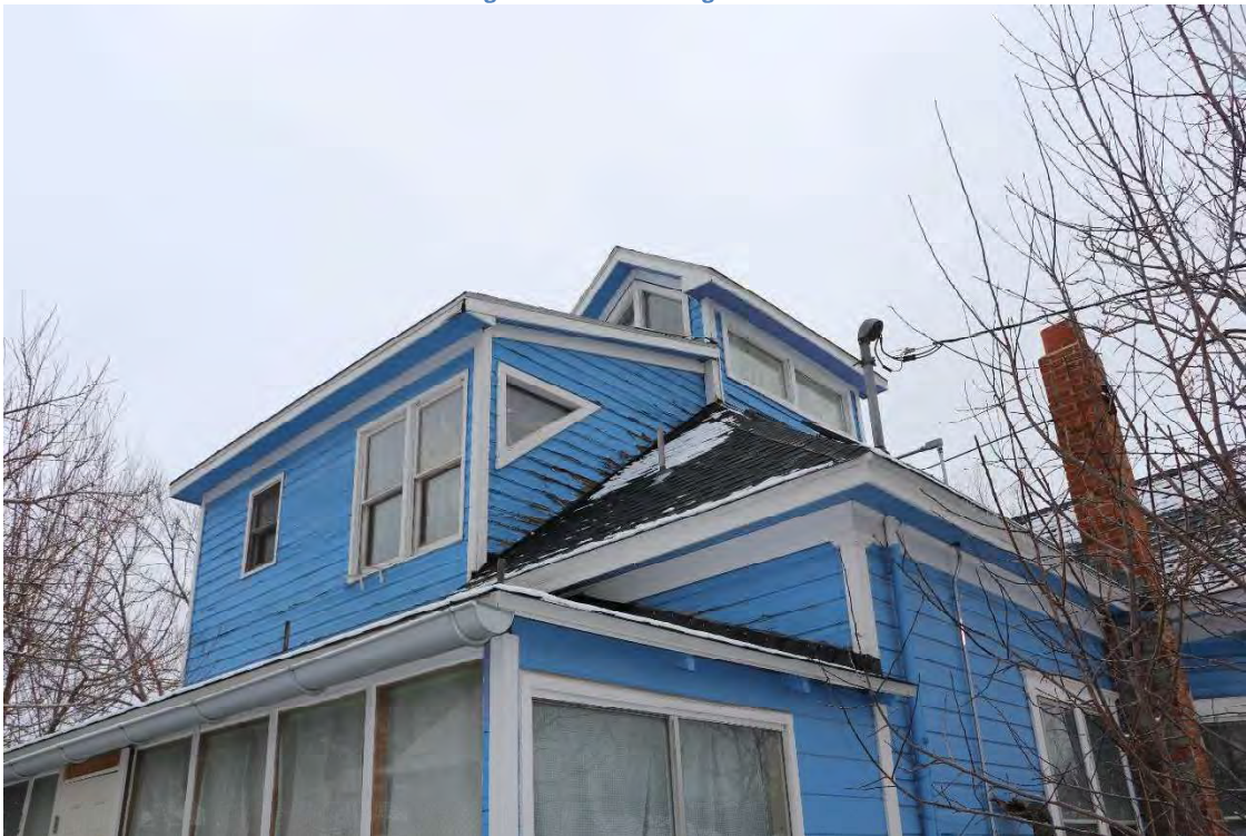
Image 12: South elevation. Original portion of the building is bottom right with corner pilaster. Note the wider siding on the enclosed porch
