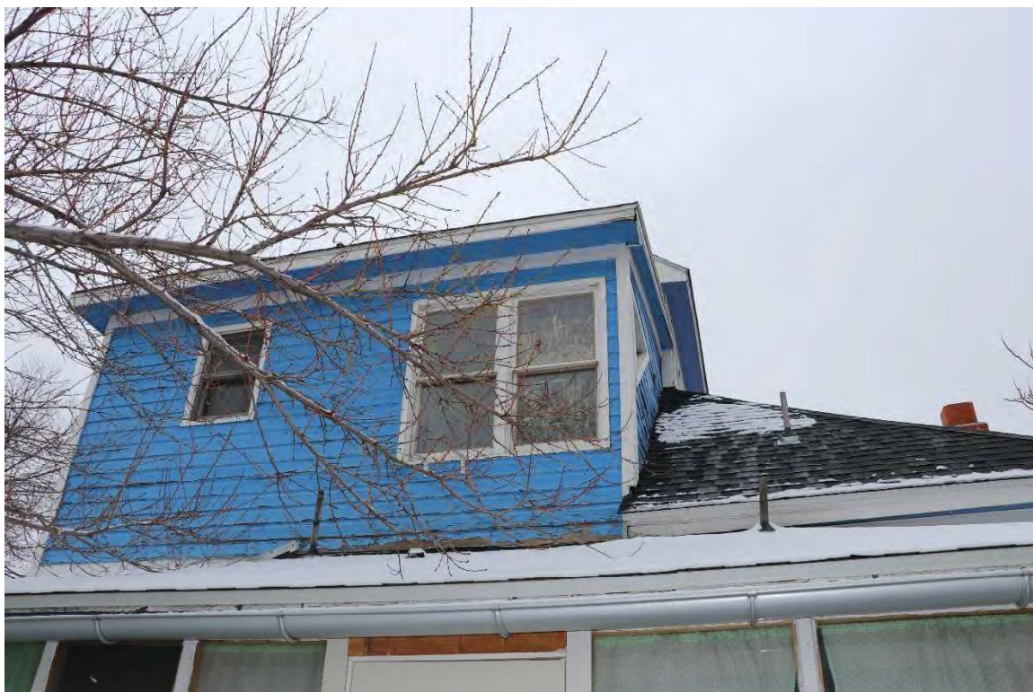
Image 39: Ventilation. Plumbing vents
