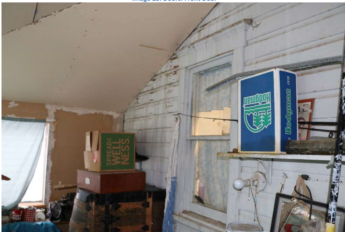
Image 24: Windows. South Elevation Exterior. Inside of enclosed porch
