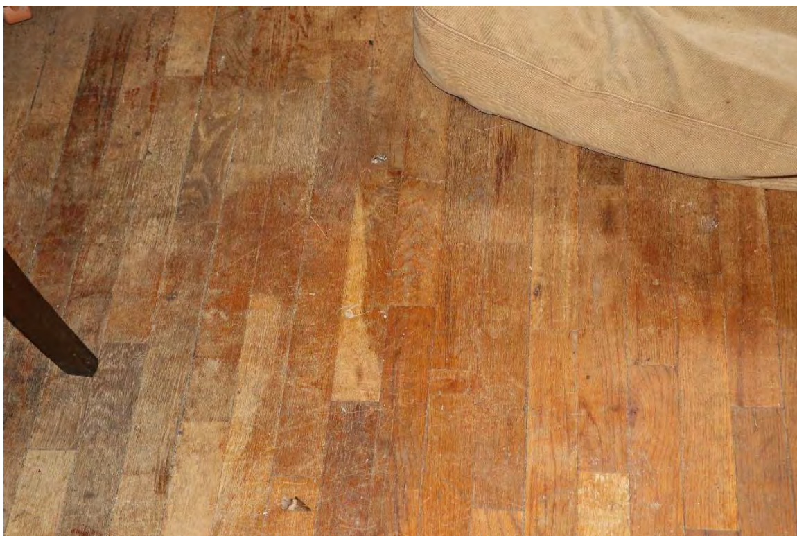
Image 36: Floor finishes. Wood floor. Typical condition
