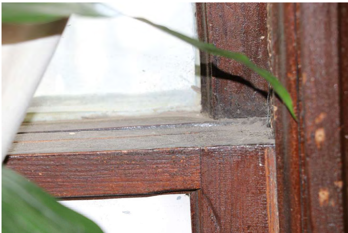
Image 27: Windows. Living Room. Sash detail
