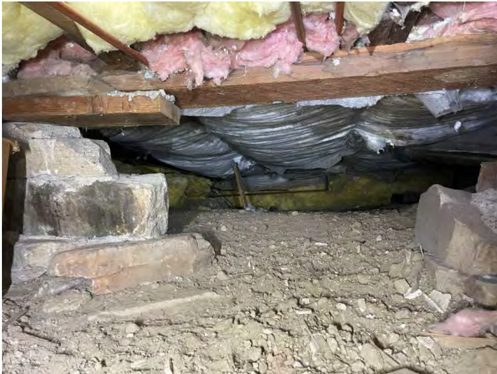
Figure 7: Crawlspace bearing line. Note one (2) 2x oriented flatwise between stone piers
