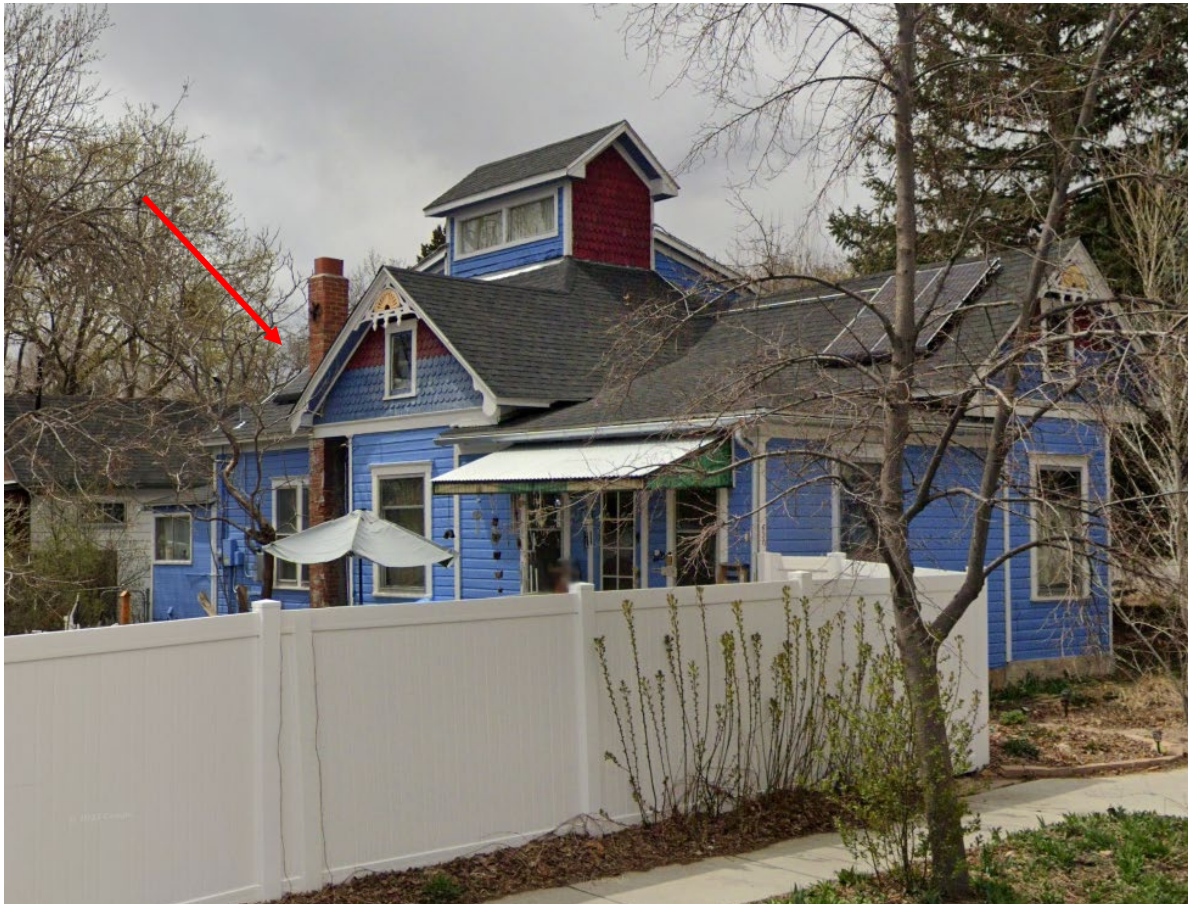
Photo of the chimney's location on the subject building.
