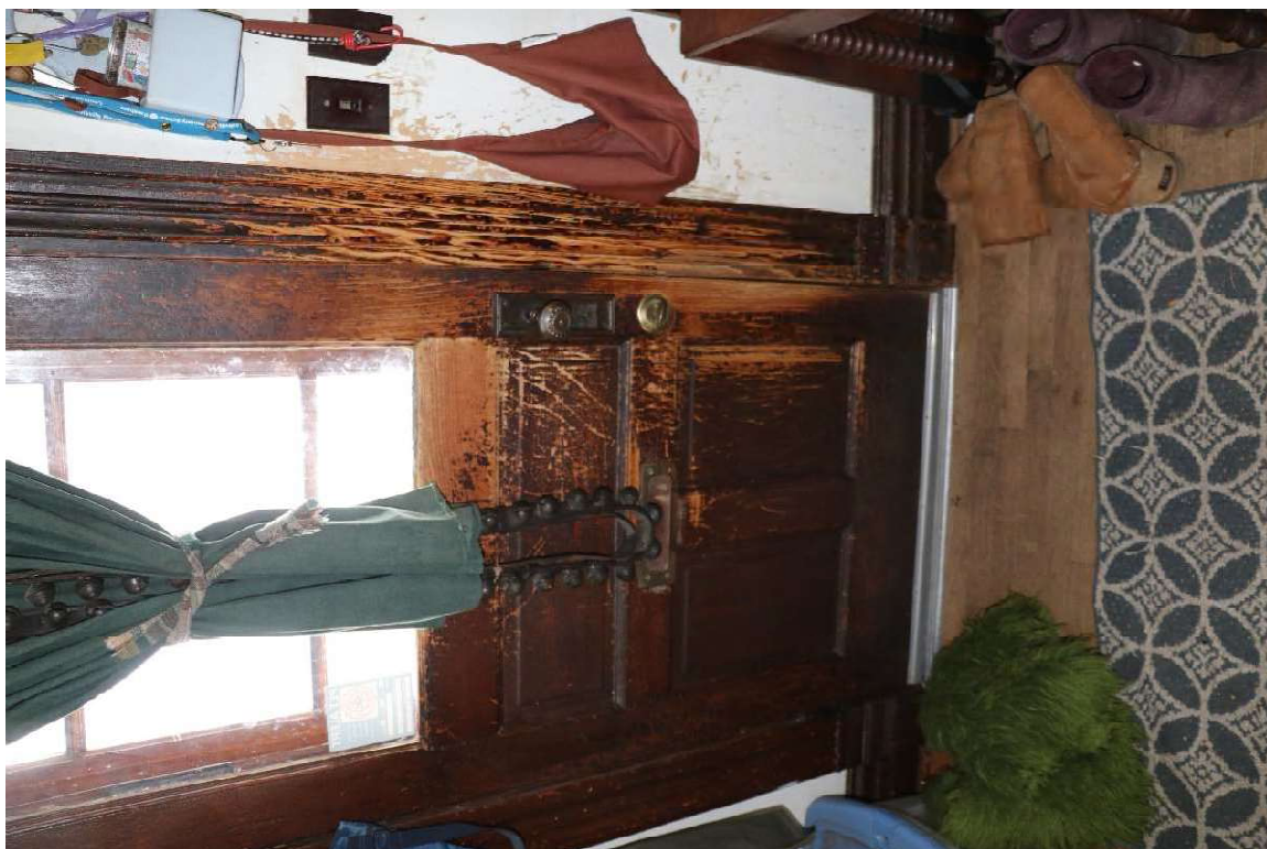
Image 23: Doors. Front Door
