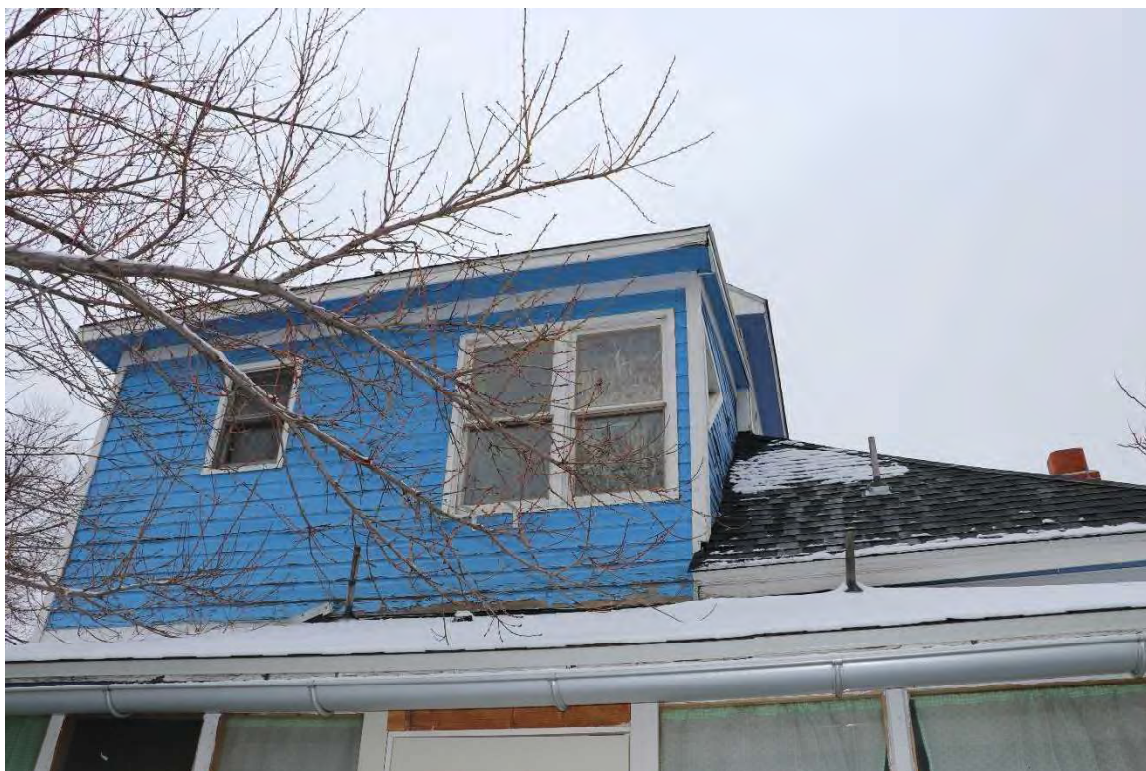
Image 18: Asphalt shingle roofing
