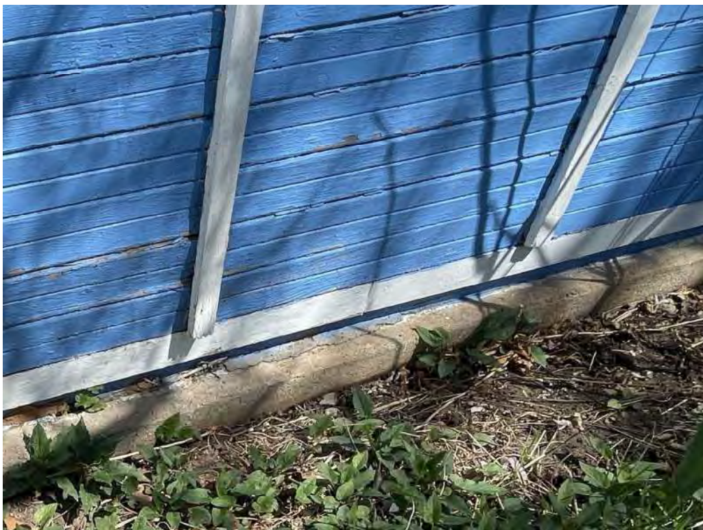
Figure 8: Parge coat over stone masonry foundation and grade proximate to wood framing
