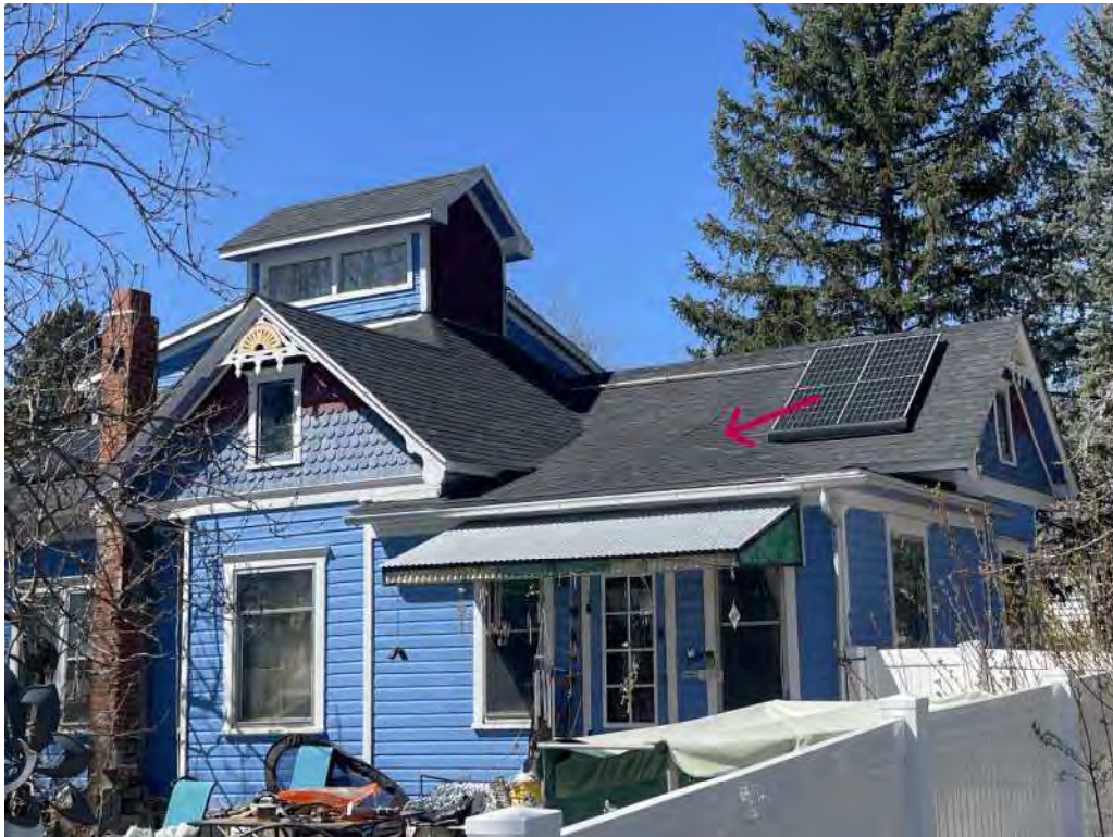
Figure 5: Northeast addition. Note over-framing at roof transition
