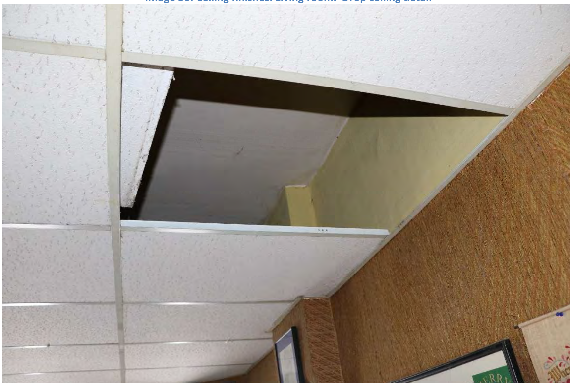
Image 31: Ceiling finishes. Living room. Drop ceiling detail
