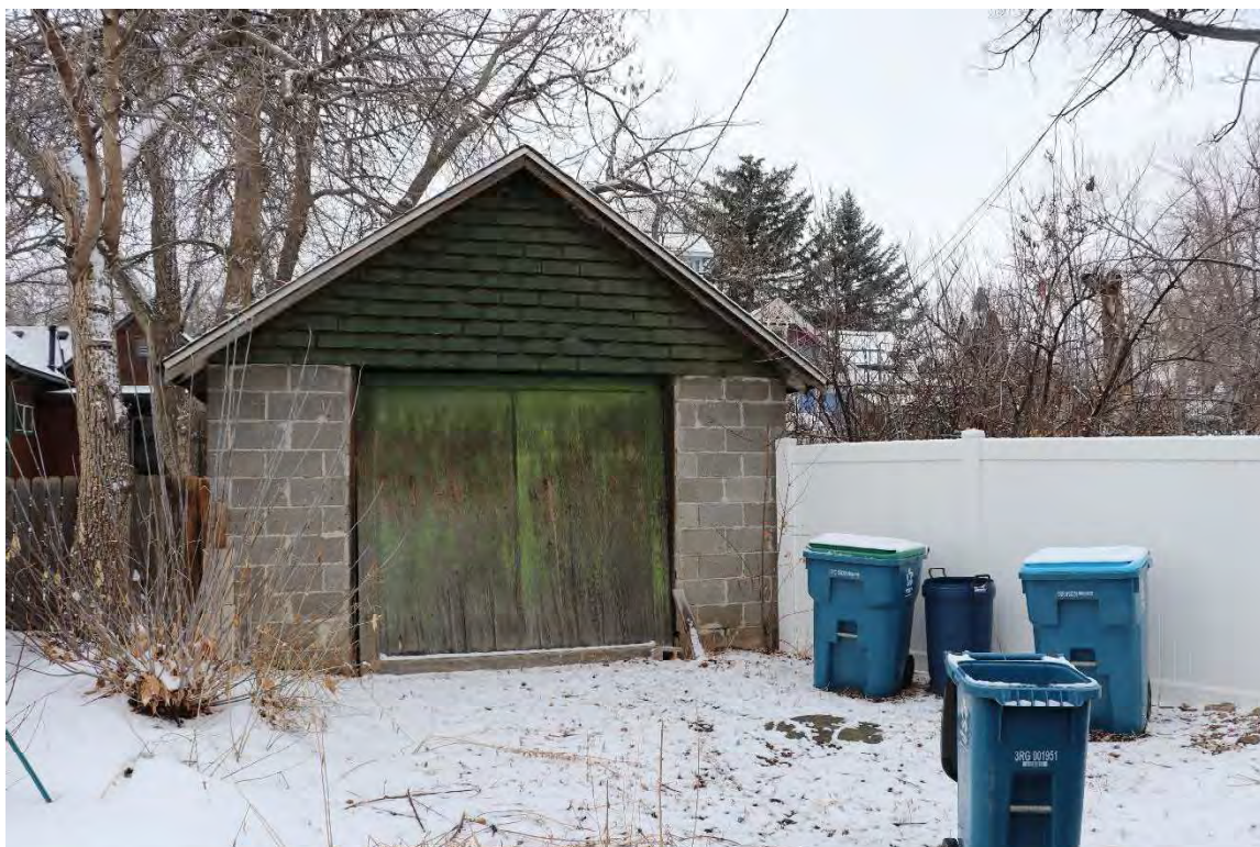
Image 3: Parking. Single car garage along alley
