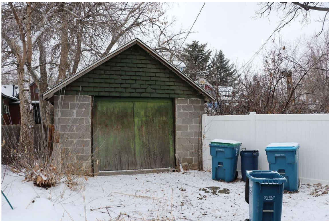
Image 3: Parking. Single car garage along alley
