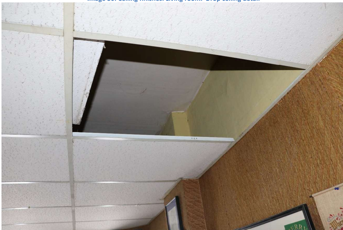
Image 31: Ceiling finishes. Living room. Drop ceiling detail
