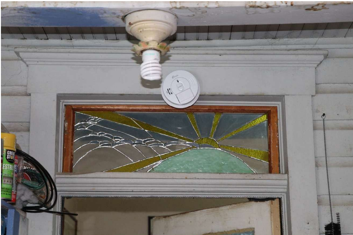
Image 10: Entry porch. Transom and casing detail
