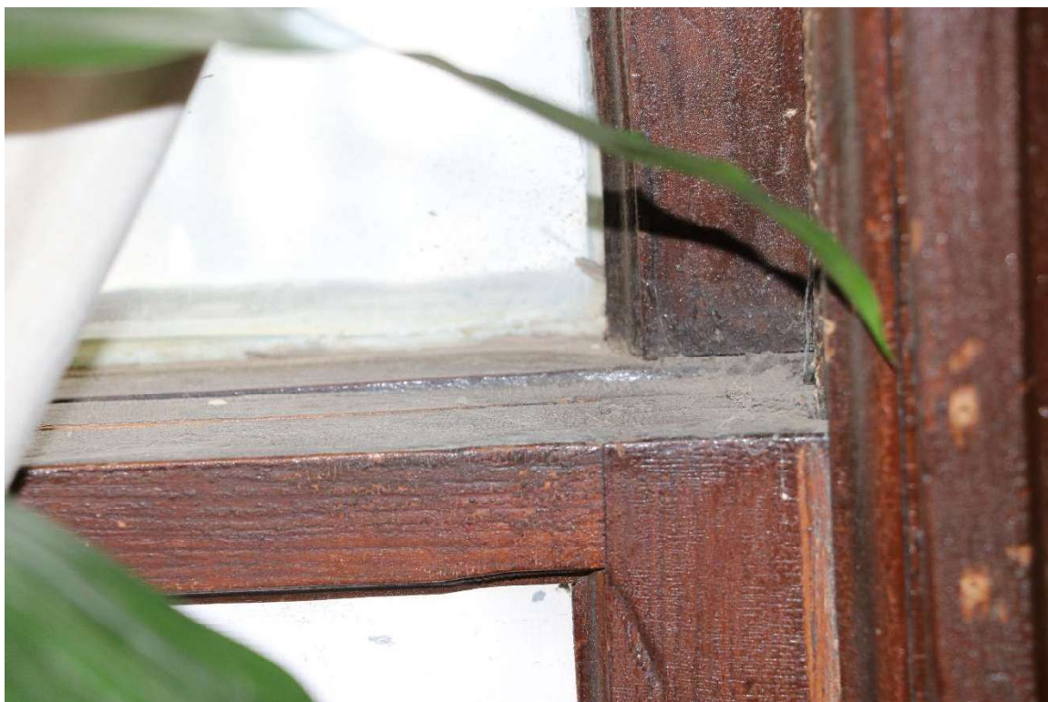
Image 27: Windows. Living Room. Sash detail
