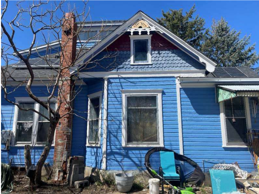
Figure 1: East elevation. Note northeast addition and chimney at roof valley
