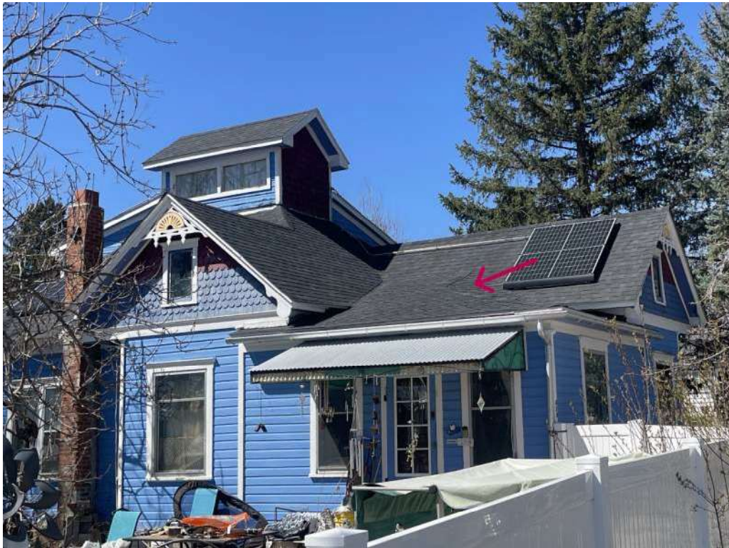
Figure 5: Northeast addition. Note over-framing at roof transition
