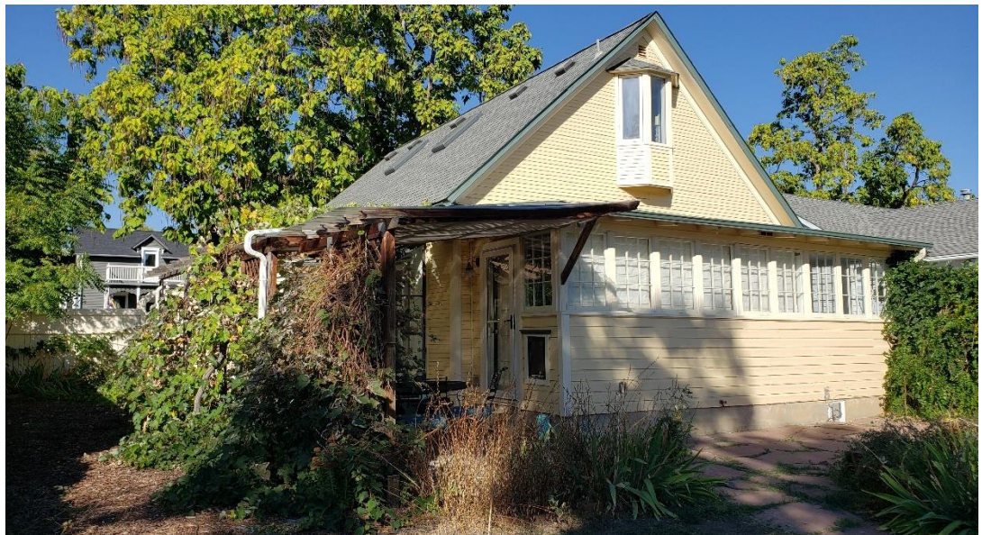
A trellis structure in the southeast corner and a bay window on the upper floor, neither of which are original.
