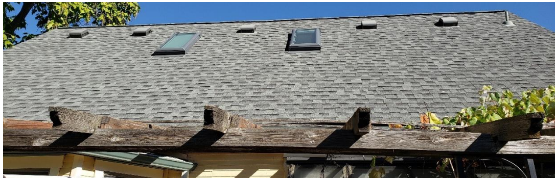
Operable skylights on the south roof aspect.
