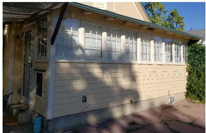
Single-pane 3-over-3 fixed windows at the east addition.
