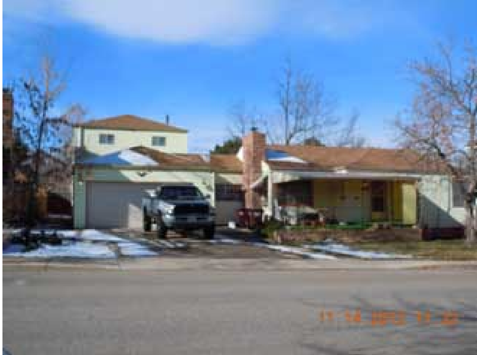
Current Boulder County Assessor photo of 1117 Lincoln.
