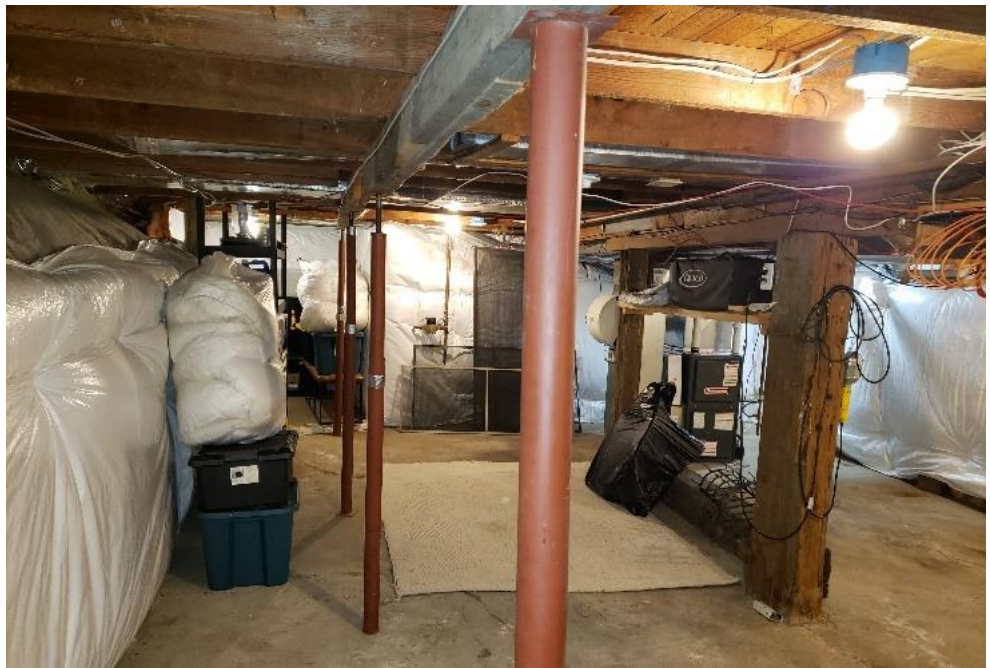
Two beam lines supporting the main floor joists with columns bearing on a concrete slab floor.
