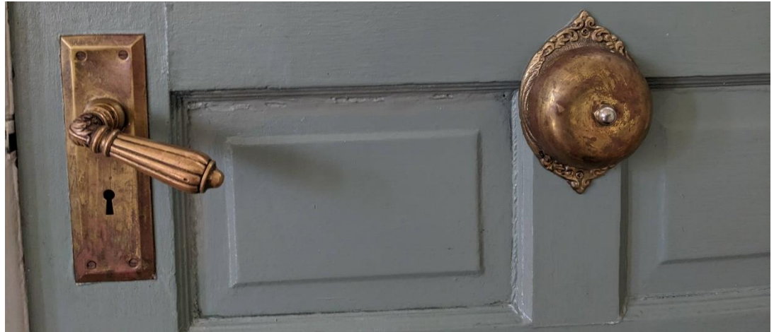
Door handle and doorbell at front door. Both could be original.
