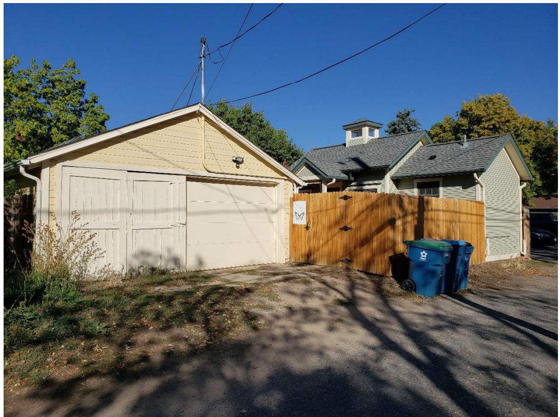
Garage and studio viewed from the alley.
