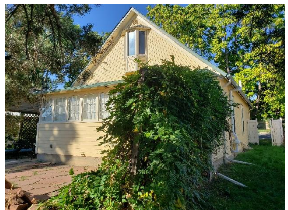
Vines growing on trellis structure.
