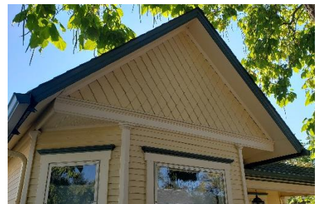
Wood shingle siding in the smaller gable end.
