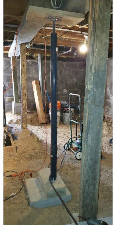
Beam & columns supporting the floor joists.
