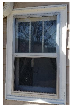
Typical single-hung wood window on north addition.
