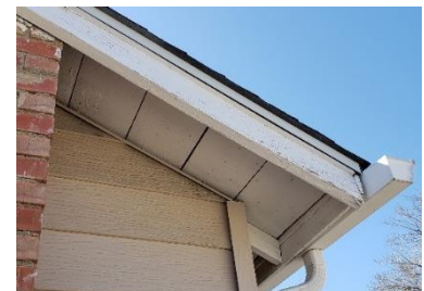
Exposed roof sheathing and rafter tails.
