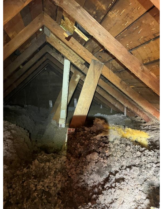
Roof framing members of original gable roof.
