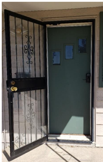
Front door and storm door.
