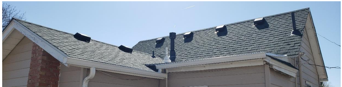
Asphalt composition shingle roof and ridge vents.
