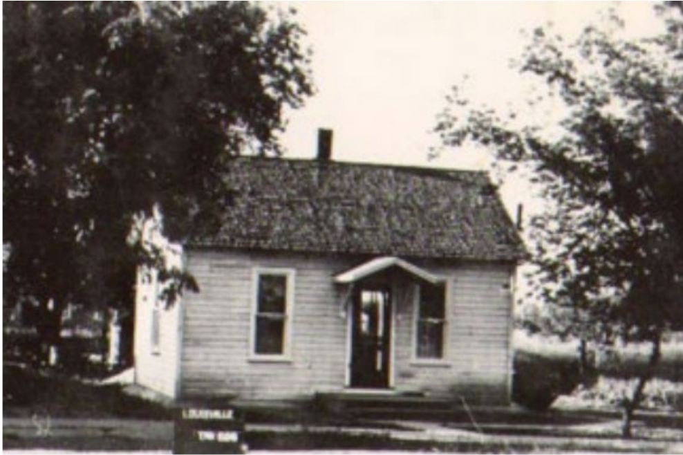
Subject property from the 1948 Assessor's Card.
