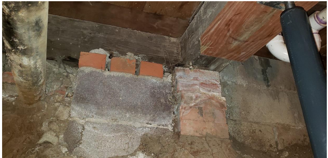
Some brick is used in various location of the foundation wall.
