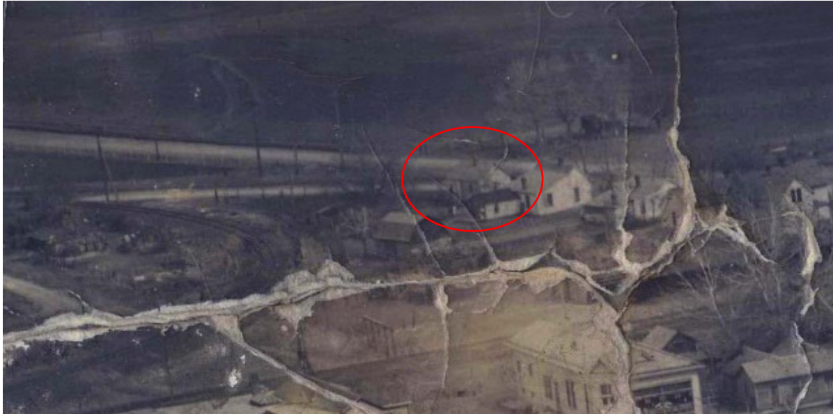
1930s aerial view looking south towards east Pine St. with eastern edge of the wye and 1155 Pine.
