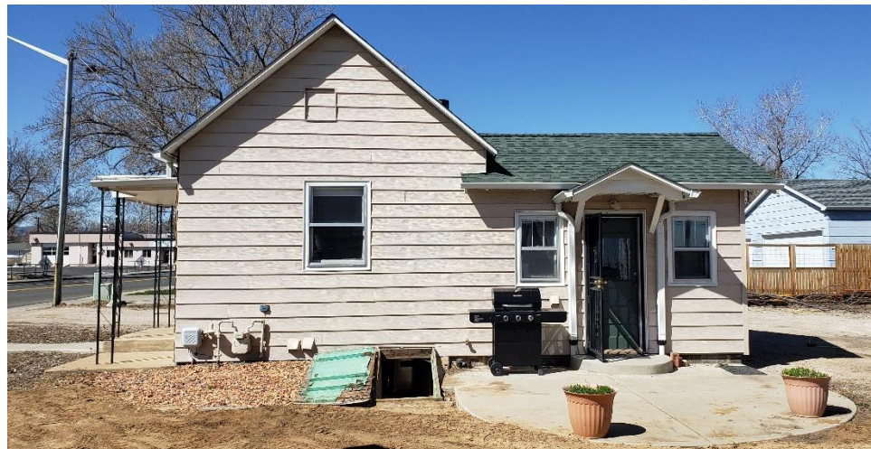
West side of the house showing an uncovered concrete porch, dirt, gravel, and mulch surrounding the house.
