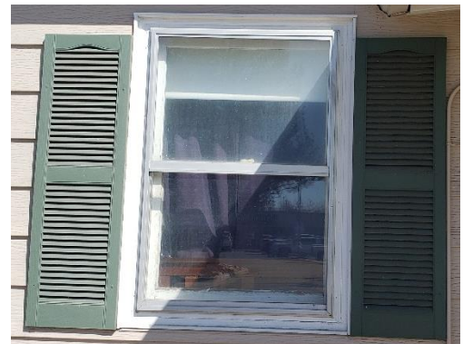
South facing single-hung wood window and vinyl shutters.
