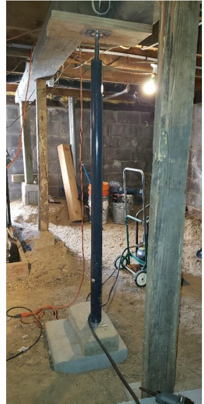
Beam & columns supporting the floor joists.
