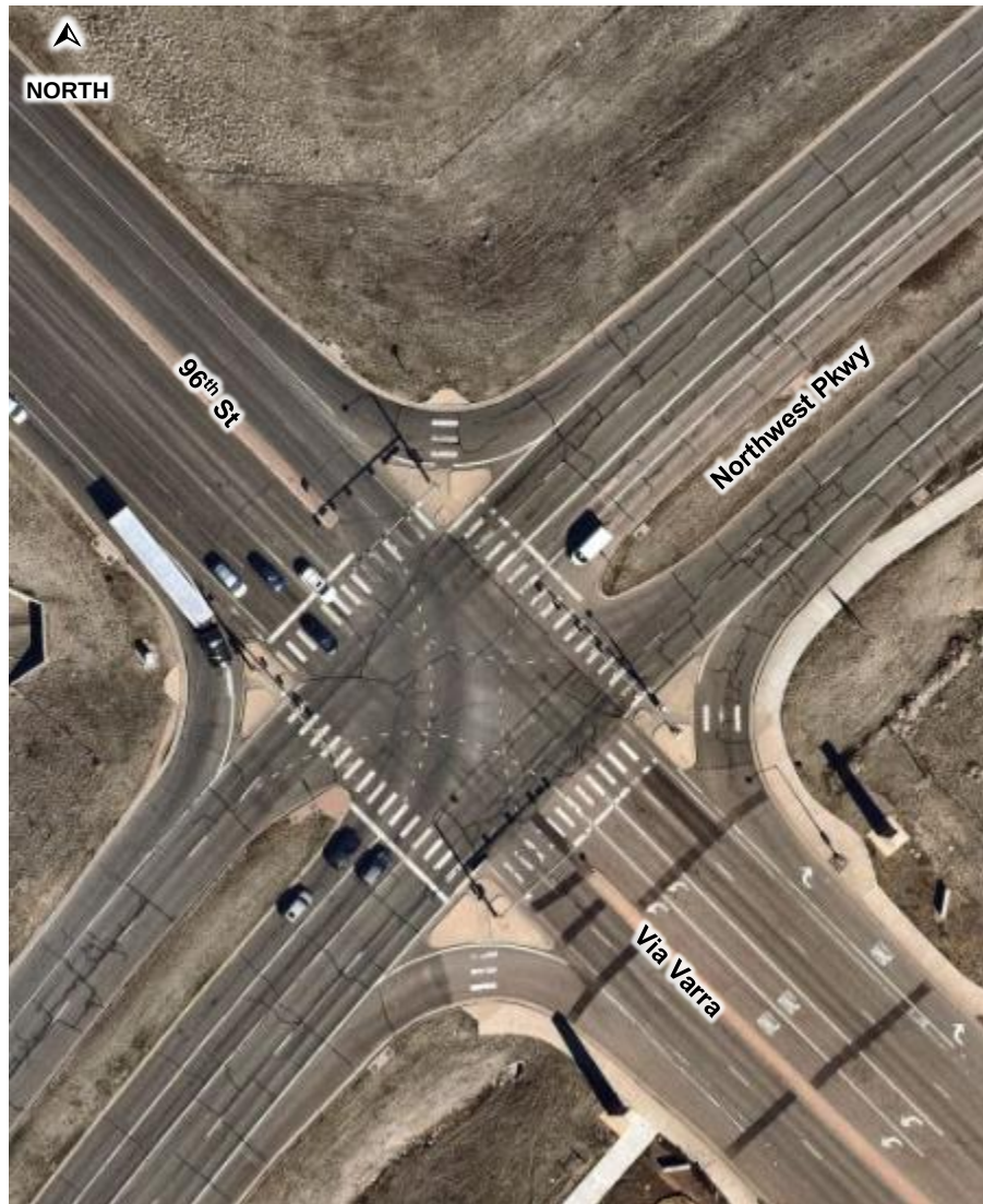
96 th Street/Via Varra & Northwest Parkway (#2)
