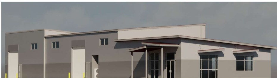
SOUTH BUILDING A - NORTHWEST ELEVATION
