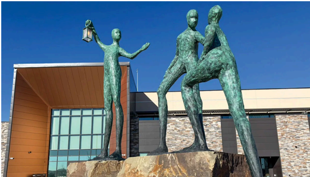
The exterior of the acute care facility at Larimer County's Longview Campus. Courtesy Larimer County Behavioral Health Services
