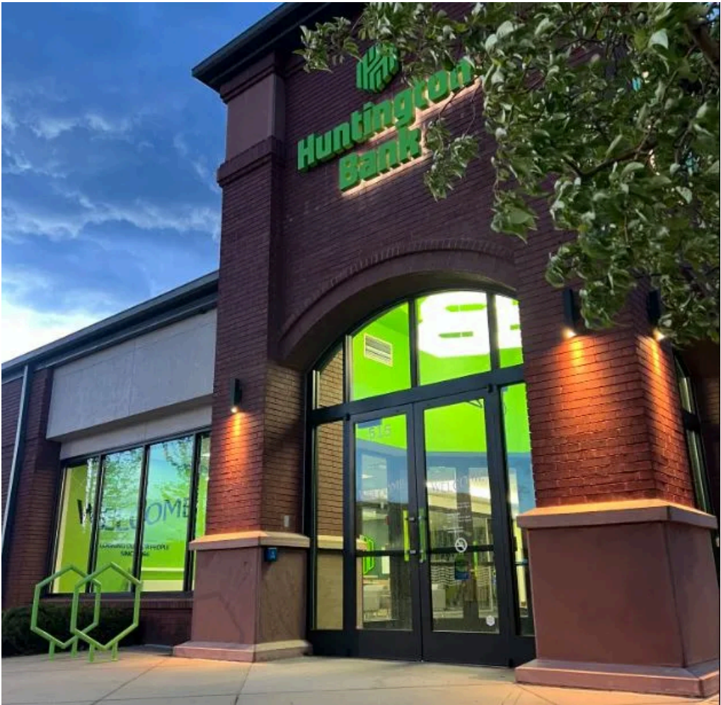
The exterior of the Huntington National Bank branch in Louisville. Courtesy Huntington.
