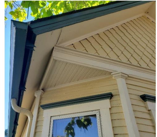
Painted wood 1x soffit & fascia at the eaves and rakes with beadboard soffit at some locations.
