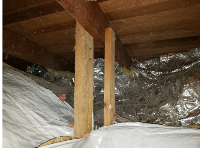
Original floor joists and floor sheathing.
