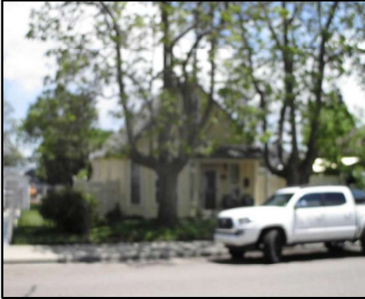
1016 Main St. FRONT VIEW 2
