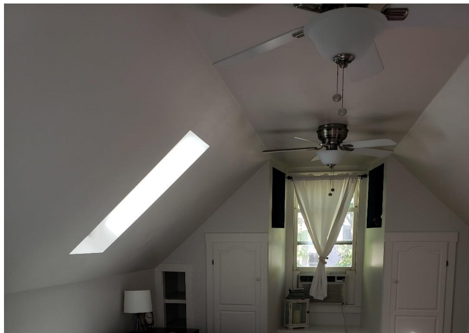
The roof pitch, flat roof, and skylight depth indicate what the roof structure might be.
