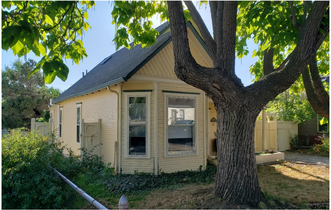
2024 View from the Northwest
