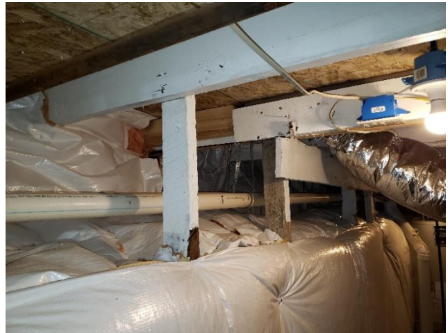
Floor joist supports bearing on a retaining wall.
