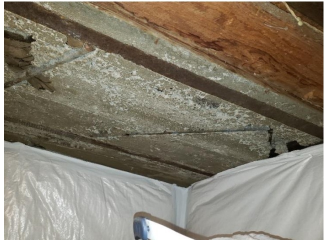
Concrete ceiling in what was previously a coal room.
