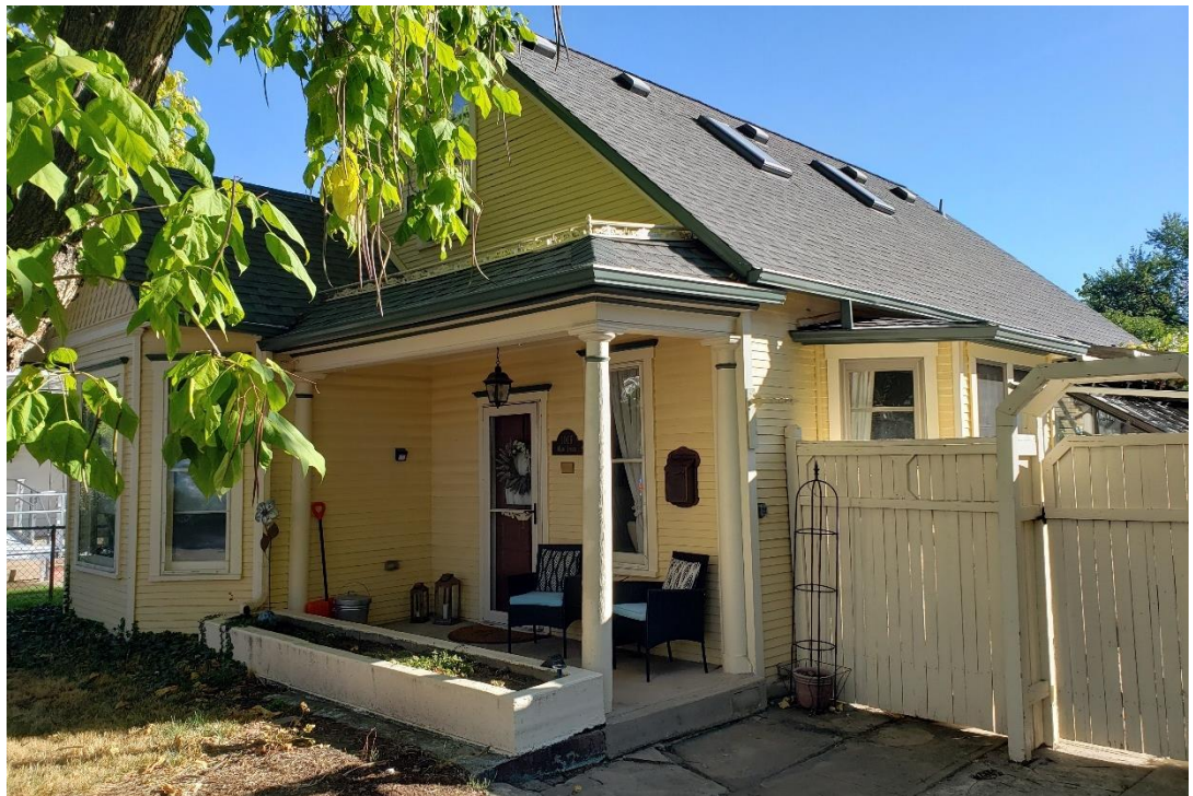
Asphalt shingle roof with roof venting near the ridge.
