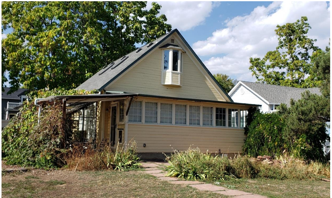
2024 View from the Southeast
