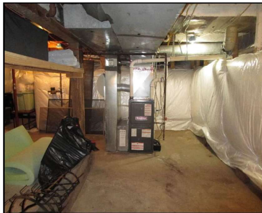
1016 Main St. CRAWL SPACE/MECH
