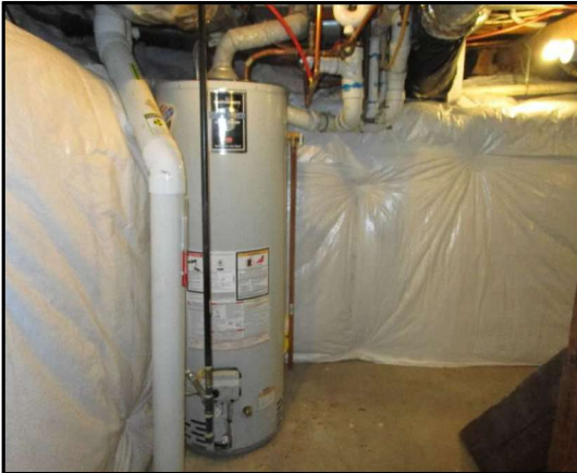
1016 Main St. CRAWL SPACE/MECH
