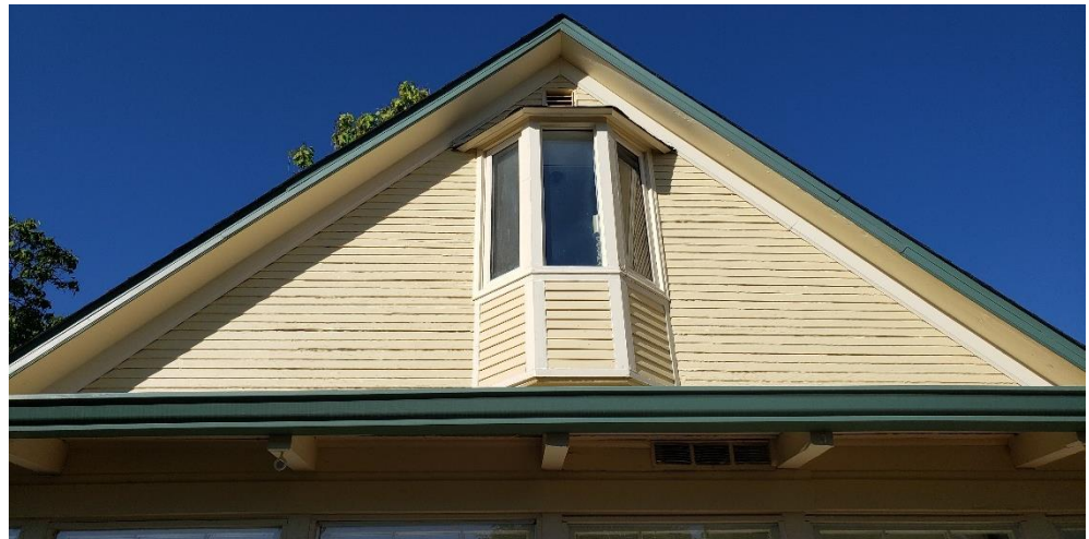
The original roof is a steep gable & the east addition roof is a low pitch with exposed rafter tails.
