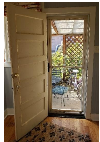
Door at east addition.
