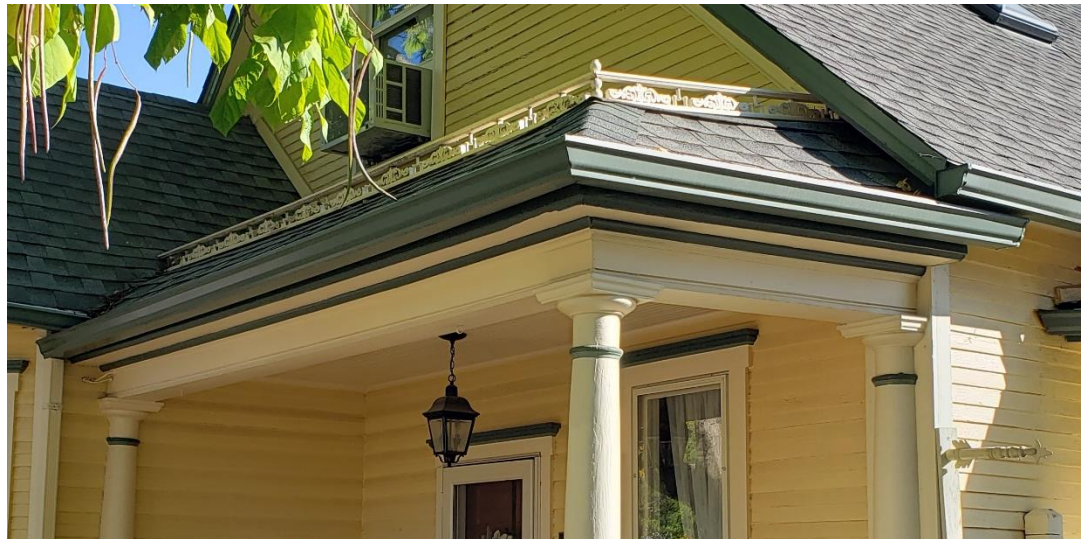
Decorative painted wood railing and column capitals at the front porch roof.
