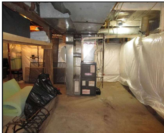
1016 Main St. CRAWL SPACE/MECH
