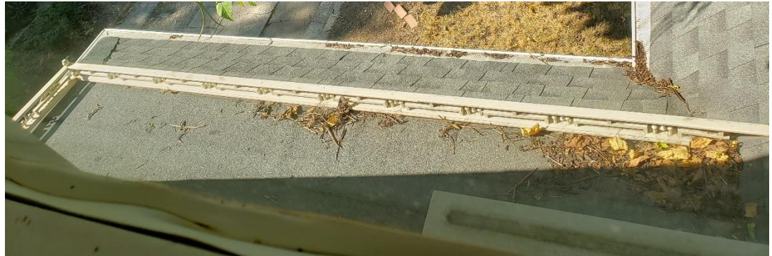
Membrane roof at the covered front porch that is also found on the east addition.
