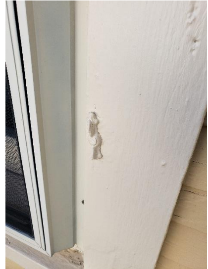
Exterior hardware previously used to hold window screens.
