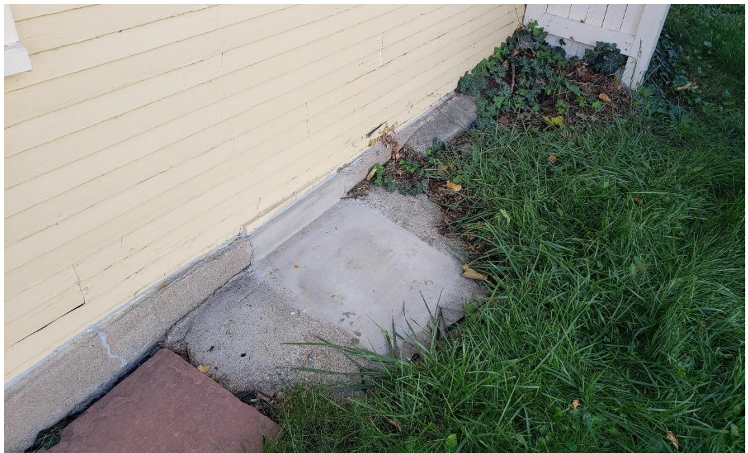
There is a slight downward grade slope to the east. The top of the foundation is minimally above grade at most locations. Also seen is the concrete foundation of an exterior chimney that was removed.
