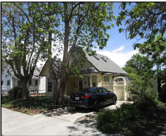
1016 Main St. FRONT VIEW 2
