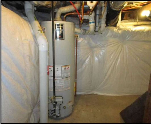
1016 Main St. CRAWL SPACE/MECH
