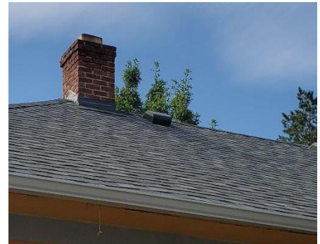
Metal flashing at the chimney-roof interface.
