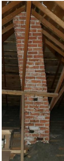
Chimney in the attic.
