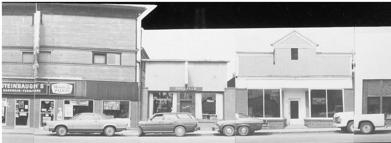
Main Street Buildings in 1978 (Photo Credit: Louisville Historical Museum)
