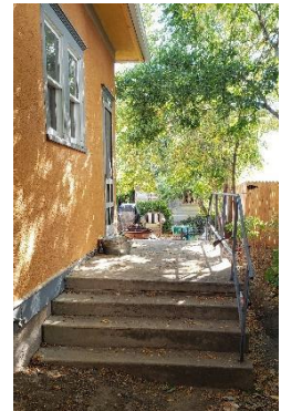
Concrete stoop on the south side of the house.
