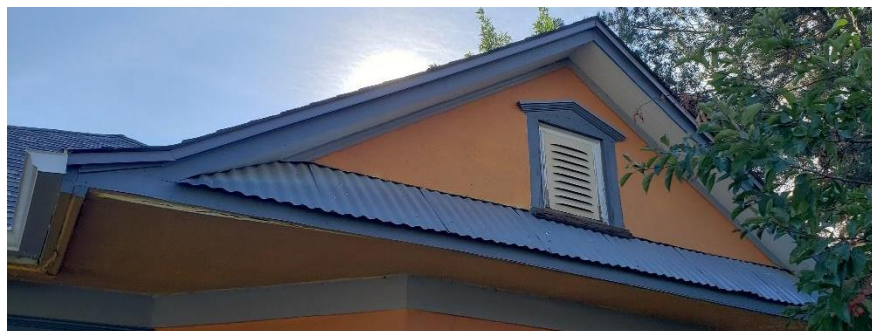
Corrugated metal roof at west facing Dutch gable.
