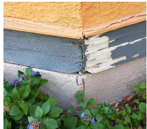
Skirt board & bead at the base of the exterior walls.
