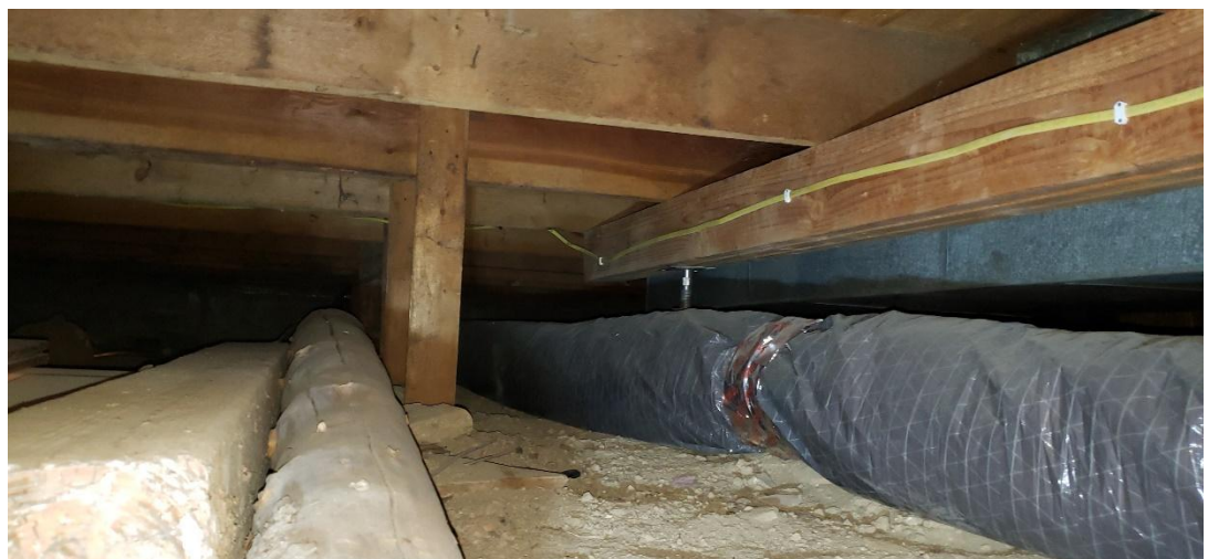
3-ply 2x6 beam, 1x joist supports, and what might have been original columns stored in the crawlspace.
