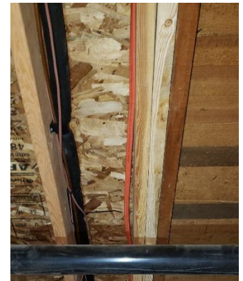
OSB sheathing left and original sheathing right.
