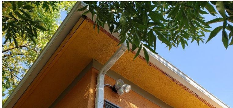
Stucco soffit and fascia ends. The fascia is minimally visible beneath the gutters.
