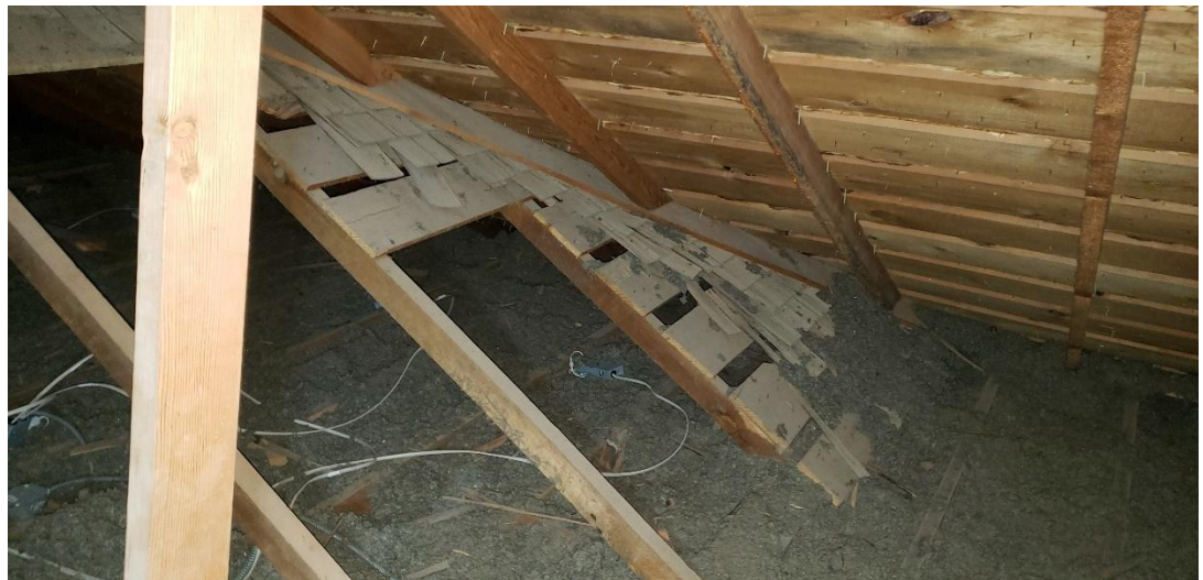
The east aspect of the original roof is visible in the attic. Some of the original skip sheathing was removed and repurposed while some of the original wood shake shingles still remain.
