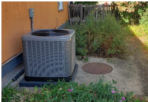
Condensing unit sitting on the concrete ceiling of the coal room.
