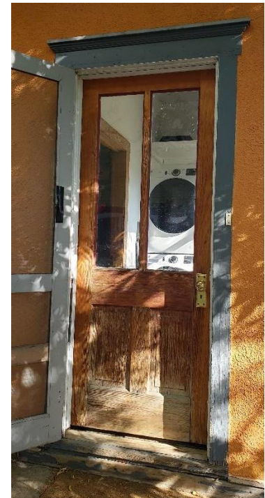
South entrance door and screen door.
