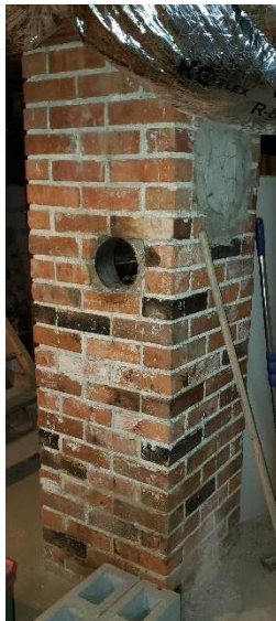
Chimney in the basement.
