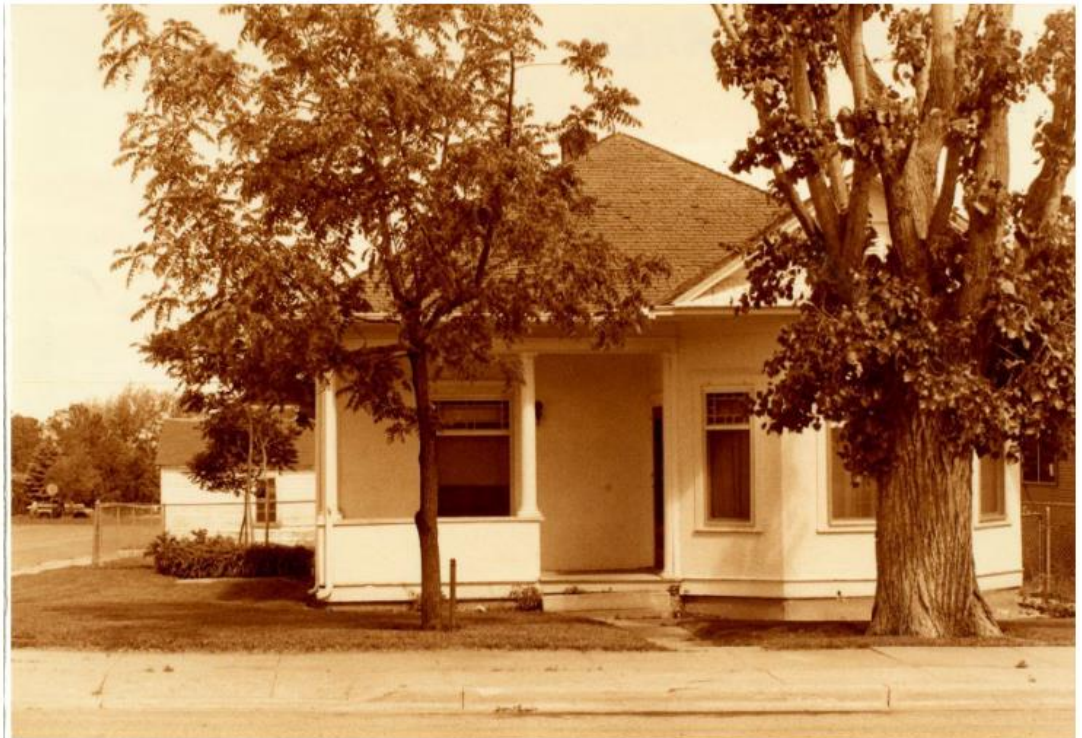
Ca. 1970s West Facade
