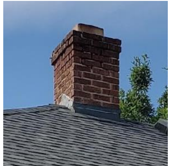
Chimney above the roof that appears to be original.
