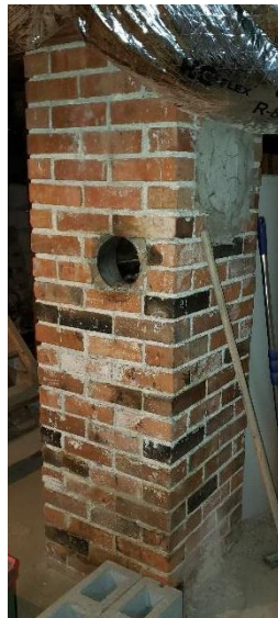
Chimney in the basement.
