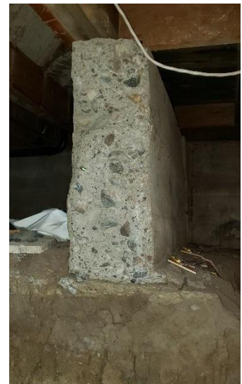
The original east foundation wall was cut to dig out the basement.
