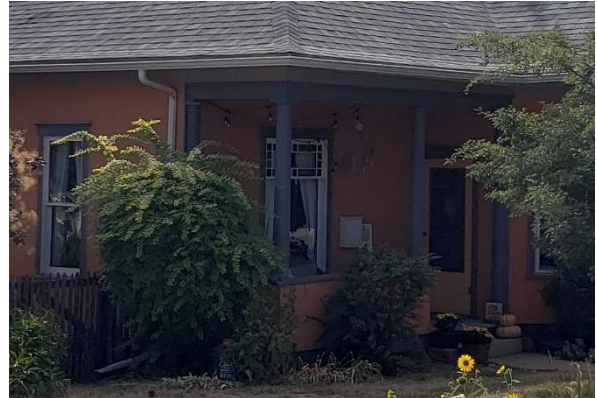
Covered front porch in the northwest corner of the house.
