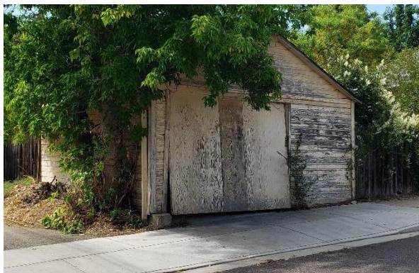
Northeast view of the garage facing South Street and near the alley. The overhead door does not appear to be operable.
