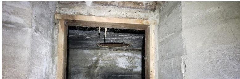
View inside the coal room looking up towards the ceiling. The concrete ceiling and cap are visible from above.
