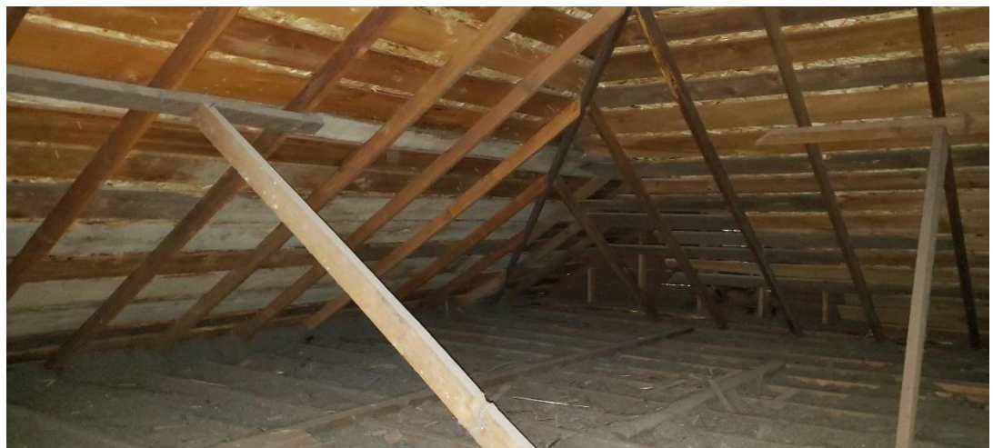
Original roof framing looking towards the west facing gable.
