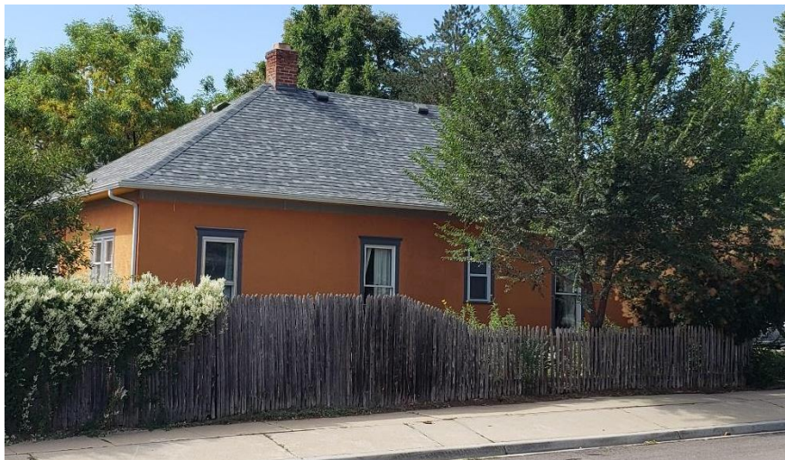
Asphalt roof and upper roof venting, both added in 2021.
