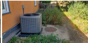
CONCRETE SUBTERRANEAN COAL ROOM ON NORTH SIDE OF THE HOUSE TO BE COMPLETELY DEMOLISHED.
