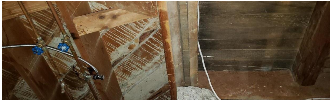
Diagonal skip sheathing of east addition on the left with original house sheathing on the right.
