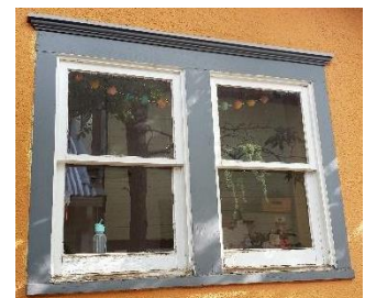
Paired, single-hung wood windows of the east addition.
