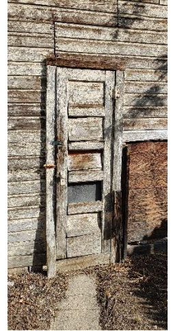
Person door on south side of the garage.
