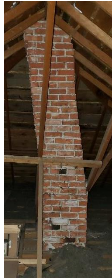
Chimney in the attic.
