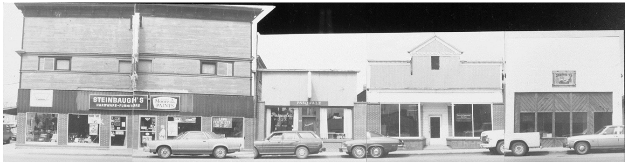
1978 view of the 800 block of Main St. showing 813 Main.
