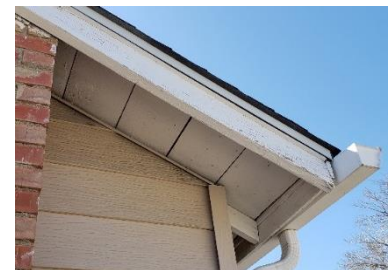
Exposed roof sheathing and rafter tails.
