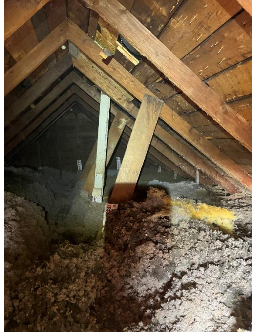
Roof framing members of original gable roof.
