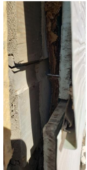
Wood shiplap siding exposed in the southeast corner.
