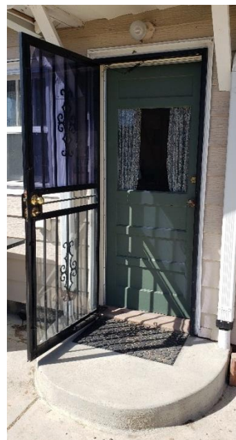
East side door and storm door.
