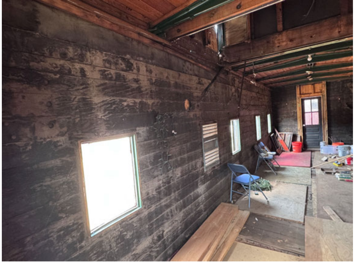
(Interior shot, Northwest wall of The Louisville Caboose, showing original wood cladding)
