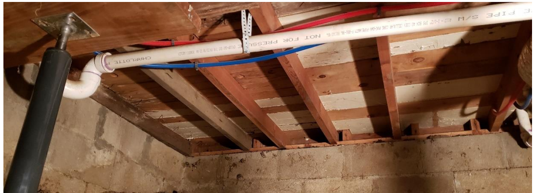
Floor joists and sheathing of the northwest addition.
