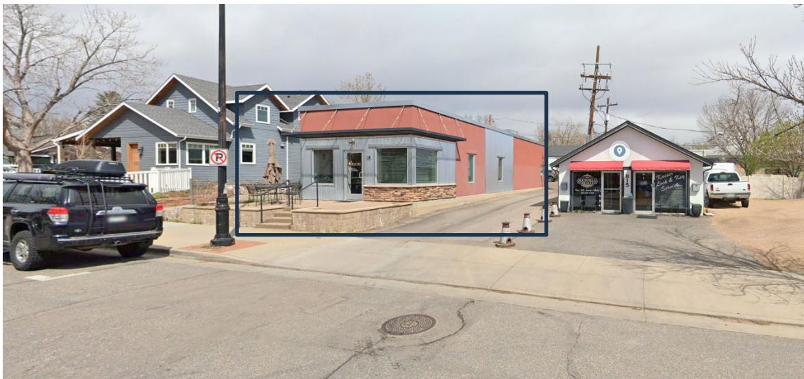
Current image of the subject property.
